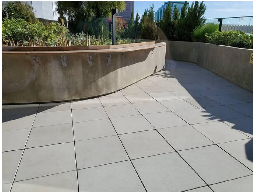
Figure 5 Pavements with High SRI Materials
