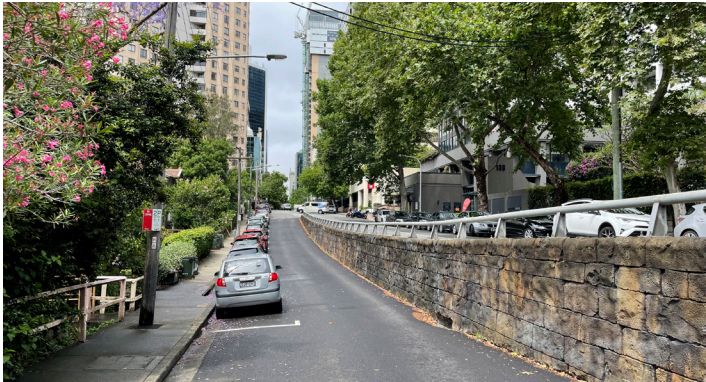
3. Level change along Walker Street Split level is divided by 2m tall retaining wall
