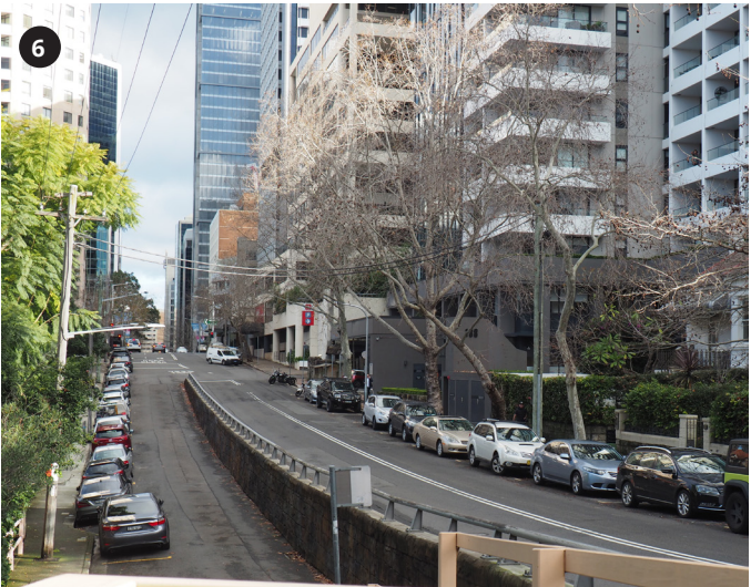
6. Hampden Street Corner Located on the northern edge of site, with a retaining wall to accomodate a significant level change
