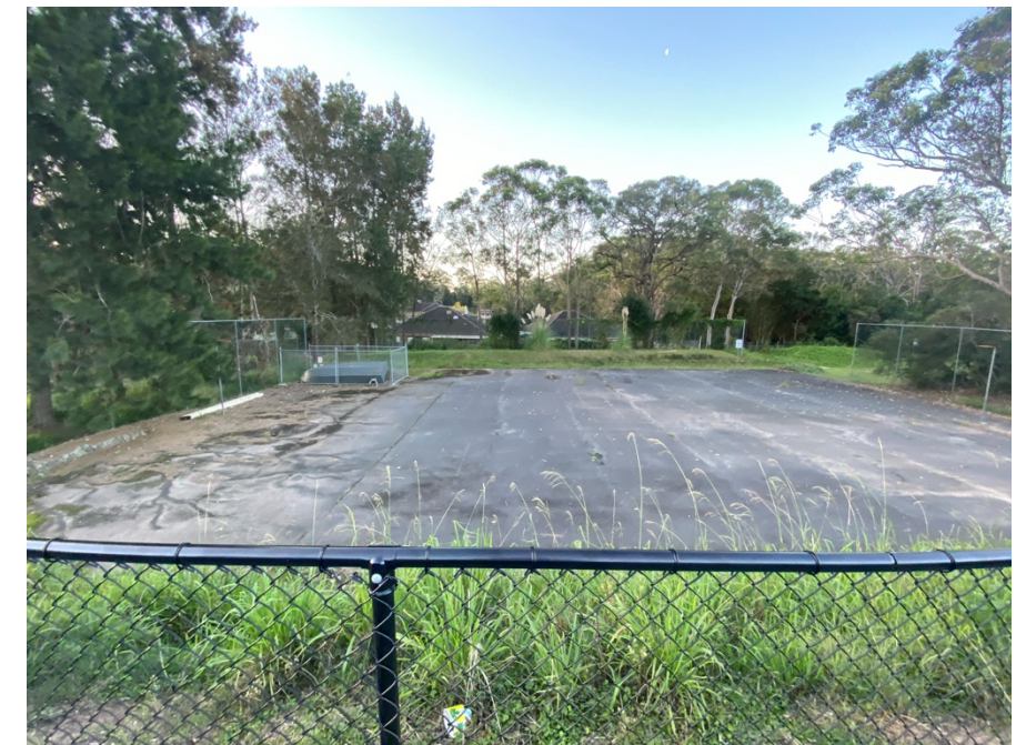
Image 18: View of Existing Eastern Netball Courts
