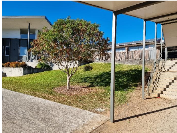
View toward south at maintained area next to existing buildings
