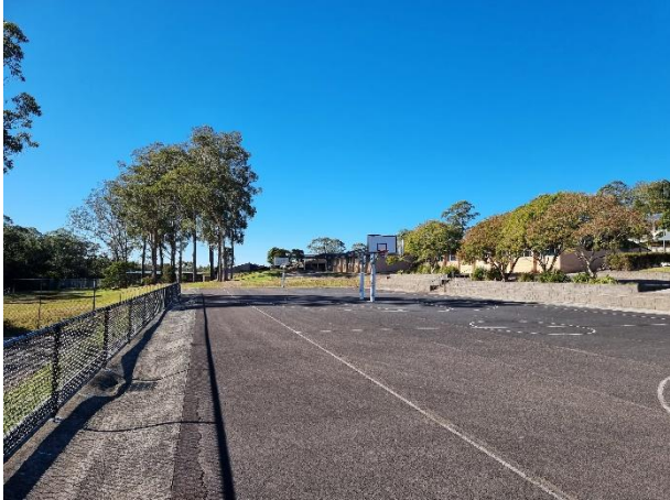
View toward east at existing basketball court
