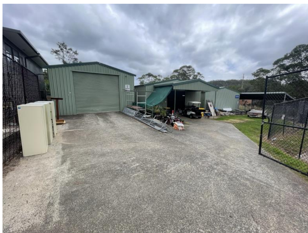
Photo 5: Picture showing the sheds present on site. Looking north-west.
