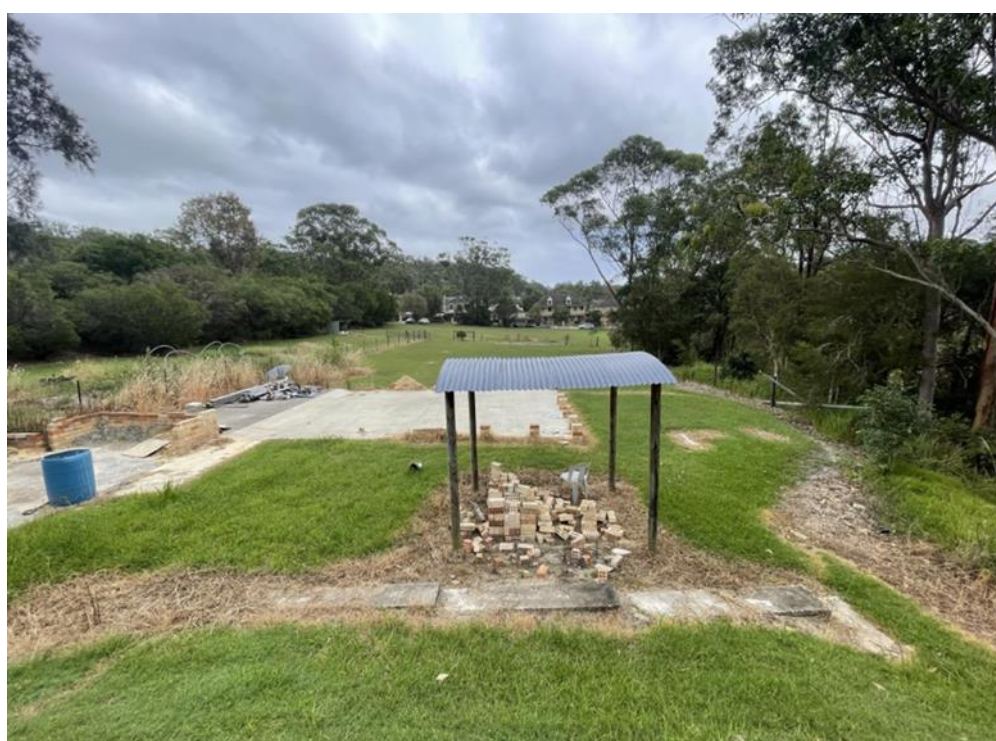
Photo 3: Overview of the site, looking west. Detail for concrete structure in front and surface water body on the right.
