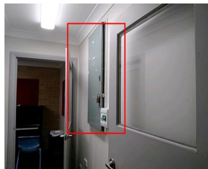
Photo No: 230621-102730 Result: Asbestos - Presumed Positive Location-Level: Interior - Ground Floor Room-Location: Electrical distribution cupboard Feature-Material: Internal insulation Item No - Risk Rating: 2 - Low
