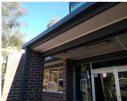
Photo No: 230620-115055 Result: Asbestos - Negative Location-Level: Exterior - Ground Floor Room-Location: All elevation of the building - eaves Feature-Material: FC sheeting
