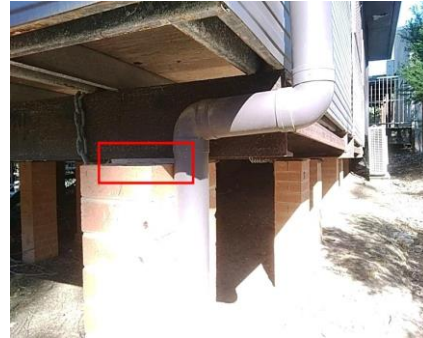
Photo No: 230620-130123 Result: Asbestos - Negative Location-Level: Exterior - Sub-floor Room-Location: All elevation of the floor - packer to support column Feature-Material: FC sheeting
