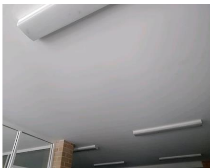
Photo No: 230620-122523 Result: Asbestos - Negative Location-Level: Interior - Ground Floor Room-Location: All elevation of the floor - ceilings Feature-Material: Plaster-like material
