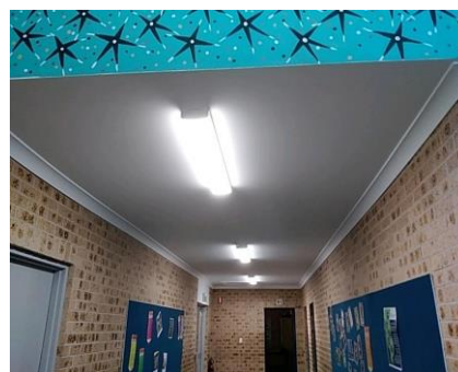
Photo No: 230620-100935 Result: Asbestos - Negative Location-Level: Interior - 1st Floor Room-Location: All elevation of the floor classroom - ceiling Feature-Material: Plaster-like material
