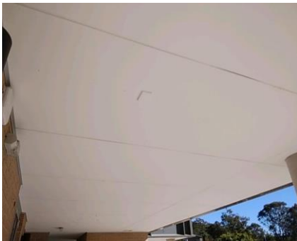
Photo No: 230620-112646 Result: Asbestos - Negative Location-Level: Exterior - Ground Floor Room-Location: All elevation of the floor - eaves Feature-Material: FC sheeting
