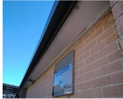
Photo No: 230621-103140 Result: Asbestos - Negative Location-Level: Exterior - Ground Floor Room-Location: All elevation of the building - eaves Feature-Material: FC sheeting
