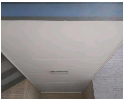
Photo No: 230620-122229 Result: Asbestos - Presumed Positive Location-Level: Exterior - 1st Floor Room-Location: Southern entrance - eaves Feature-Material: FC sheeting Item No - Risk Rating: 4 - Low
