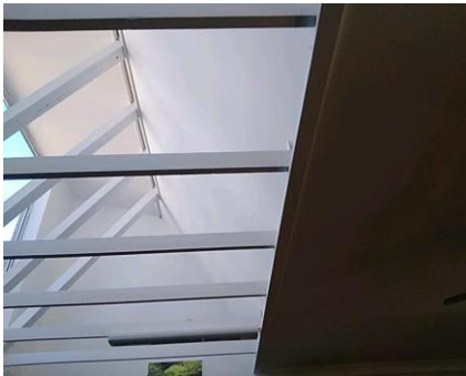
Photo No: 230621-104730 Result: Asbestos - Negative Location-Level: Interior - Ground Floor Room-Location: All elevation of the floor - internal ceilings Feature-Material: Plaster-like material
