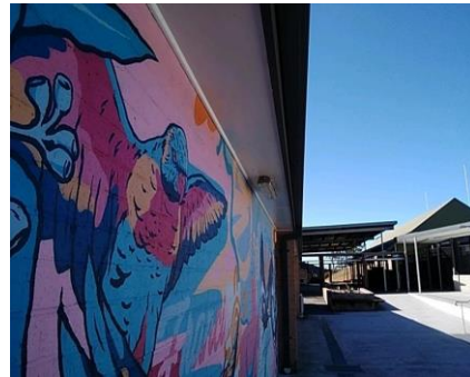
Photo No: 230621-104914 Result: Asbestos - Negative Location-Level: Exterior - Ground Floor Room-Location: All elevation of the building - eaves Feature-Material: FC sheeting
