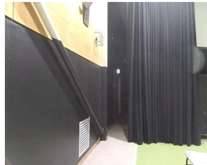
Photo No: 230620-105529 Result: Asbestos - Negative Location-Level: Interior - Ground Floor Room-Location: Hall - internal walls Feature-Material: FC sheeting
