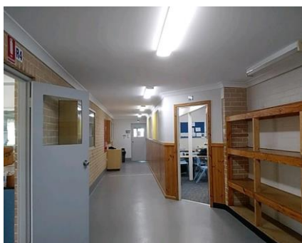
Photo No: 230620-124915 Result: Asbestos - Negative Location-Level: Interior - Ground Floor Room-Location: All elevation of the floor - division walls Feature-Material: Plaster-like material
