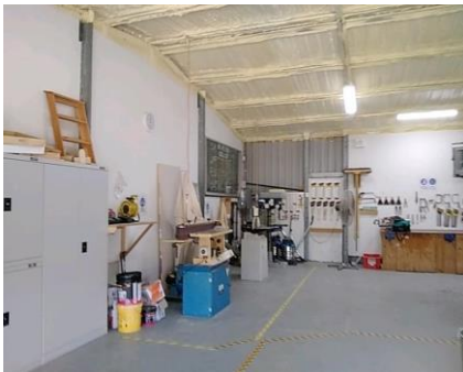
Photo No: 230620-104931 Result: Asbestos - Negative Location-Level: Interior - Ground Floor Room-Location: All elevation of the floor - walls Feature-Material: Plaster-like material
