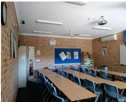
Photo No: 230626-003710 Result: Asbestos - Negative Location-Level: Interior - Ground Floor Room-Location: All elevation of the floor: classrooms - ceilings Feature-Material: Plaster-like material
