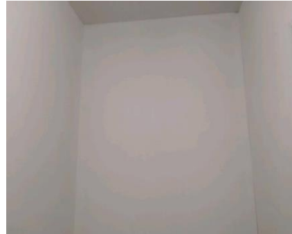
Photo No: 230620-120450 Result: Asbestos - Negative Location-Level: Interior - Ground Floor Room-Location: All elevation of the floor - internal walls Feature-Material: Plaster-like material
