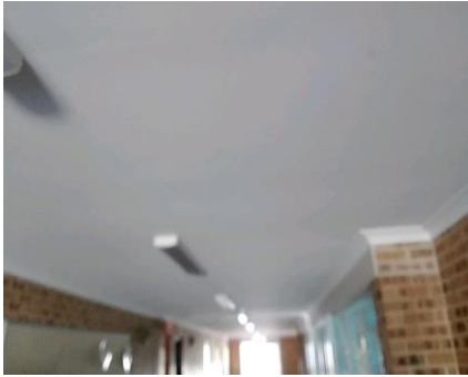
Photo No: 230621-105154 Result: Asbestos - Negative Location-Level: Interior - Ground Floor Room-Location: All elevation of the floor - ceiling Feature-Material: Plaster-like material
