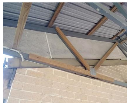
Photo No: 230620-122759 Result: Asbestos - Negative Location-Level: Interior - Ground Floor Room-Location: roof gables Feature-Material: FC sheeting
