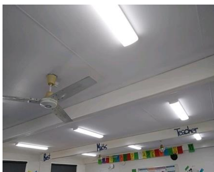
Photo No: 230620-100435 Result: Asbestos - Negative Location-Level: Interior - Ground Floor Room-Location: All elevation of the floor - ceilings Feature-Material: Plaster-like material
