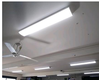
Photo No: 230620-095403 Result: Asbestos - Negative Location-Level: Interior - Ground Floor Room-Location: Classroom - ceiling Feature-Material: Plaster-like material
