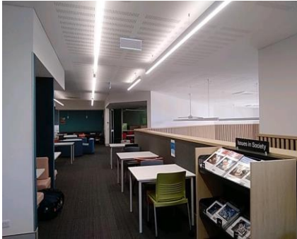
Photo No: 230620-112929 Result: Asbestos - Negative Location-Level: Interior - 1st Floor Room-Location: All elevation of the floor - internal walls and ceilings Feature-Material: Plaster-like material
