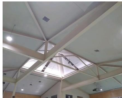
Photo No: 230620-105805 Result: Asbestos - Presumed Positive Location-Level: Interior - Ground Floor Room-Location: Hall - internal ceilings Feature-Material: FC sheeting Item No - Risk Rating: 2 - Low
