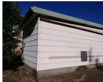
Photo No: 230621-101520 Result: Asbestos - Negative Location-Level: Interior and Exterior - Ground Floor Room-Location: All elevation of the building - walls and eaves Feature-Material: FC sheeting
