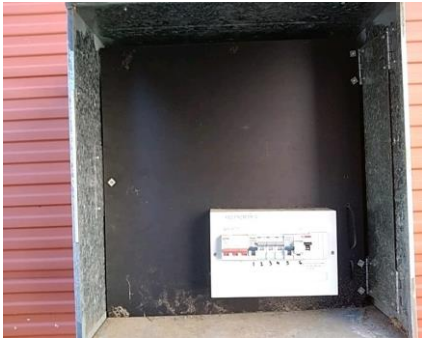
Photo No: 230620-095900 Result: Asbestos - Presumed Positive Location-Level: Exterior - Ground Floor Room-Location: Western elevation of the building - electrical distribution board Feature-Material: Bituminous-like material Item No - Risk Rating: 4 - Low
