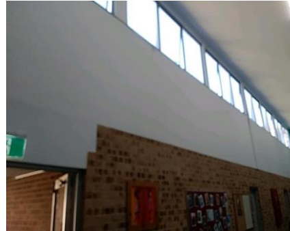
Photo No: 230620-102755 Result: Asbestos - Negative Location-Level: Interior - 1st Floor Room-Location: All elevation of the floor - infill panels to walls Feature-Material: Plaster-like material
