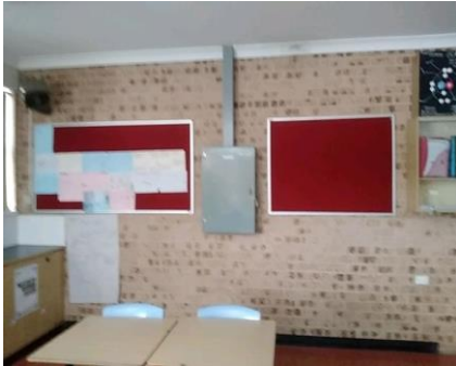
Photo No: 230620-111158 Result: Asbestos - Presumed Positive Location-Level: Interior - Ground Floor Room-Location: Electrical box Feature-Material: Backing board, no access Item No - Risk Rating: 3 - Low
