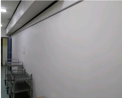
Photo No: 230620-120214 Result: Asbestos - Negative Location-Level: Interior - 1st Floor Room-Location: Canteen storage area - internal walls Feature-Material: FC sheeting
