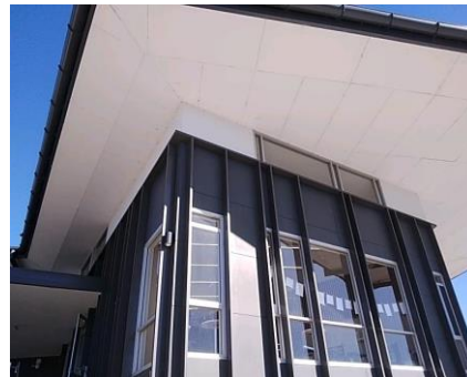
Photo No: 230620-112721 Result: Asbestos - Negative Location-Level: Interior - Roof Room-Location: All elevation of 1st and roof - eaves Feature-Material: FC sheeting
