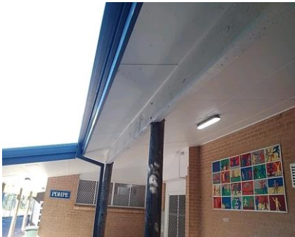
Photo No: 230620-125531 Result: Asbestos - Negative Location-Level: Exterior - Ground Floor Room-Location: All elevation of the building - eaves Feature-Material: FC sheeting
