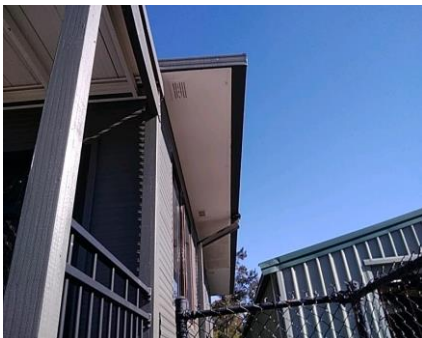
Photo No: 230620-104559 Result: Asbestos - Presumed Positive Location-Level: Exterior - Ground Floor Room-Location: All elevation of the building - eaves Feature-Material: FC sheeting Item No - Risk Rating: 2 - Low
