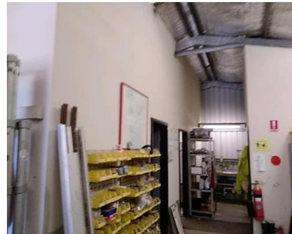
Photo No: 230620-104750 Result: Asbestos - Negative Location-Level: Interior - Ground Floor Room-Location: All elevation of the floor - division walls Feature-Material: Plaster-like material
