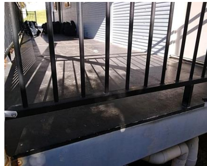
Photo No: 230620-103753 Result: Asbestos - Negative Location-Level: Exterior - Ground Floor Room-Location: Landing - flooring Feature-Material: FC sheeting
