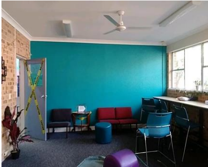
Photo No: 230620-101152 Result: Asbestos - Negative Location-Level: Interior - 1st Floor Room-Location: All elevation of the floor - division walls Feature-Material: Plaster-like material
