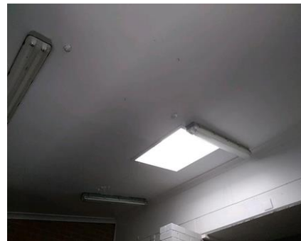
Photo No: 230621-094823 Result: Asbestos - Negative Location-Level: Interior - Ground Floor Room-Location: All elevation of the floor - ceilings Feature-Material: FC sheeting
