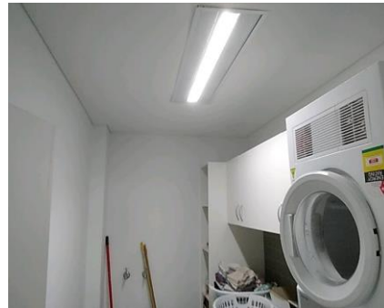
Photo No: 230620-121421 Result: Asbestos - Negative Location-Level: Interior - 1st Floor Room-Location: Laundry - internal walls and ceiling Feature-Material: Plaster-like material
