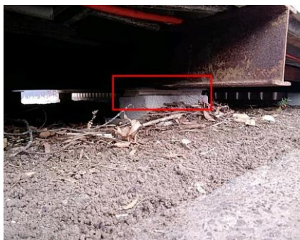
Photo No: 230620-095652 Result: Asbestos - Negative Location-Level: Exterior - Sub-floor Room-Location: All elevation of the floor - packer to support column Feature-Material: FC sheeting
