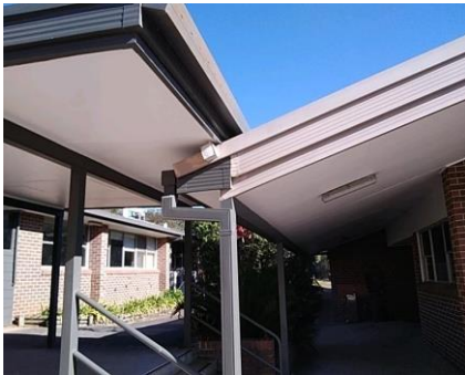
Photo No: 230620-102828 Result: Asbestos - Negative Location-Level: Exterior - 1st Floor Room-Location: Corridor to courtyard Feature-Material: FC sheeting
