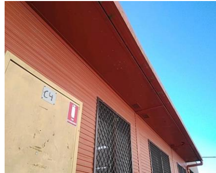
Photo No: 230620-095916 Result: Asbestos - Presumed Positive Location-Level: Exterior - Ground Floor Room-Location: All elevation of the building - eaves Feature-Material: FC sheeting Item No - Risk Rating: 5 - Low
