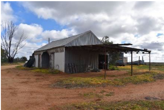
PHOTOGRAPH 5.5 VIEW WEST OF MACHINERY SHED ADJACENT TO SHEARING SHED (ERM 2024)
