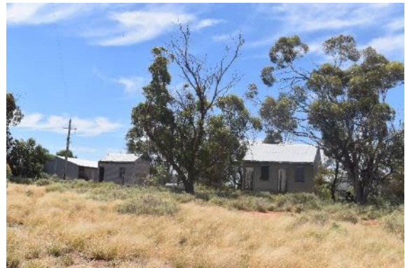
PHOTOGRAPH 5.6 VIEW EAST OF WORKERS ACCOMMODATION TO WEST OF MAIN RESIDENCE (ERM 2024)
