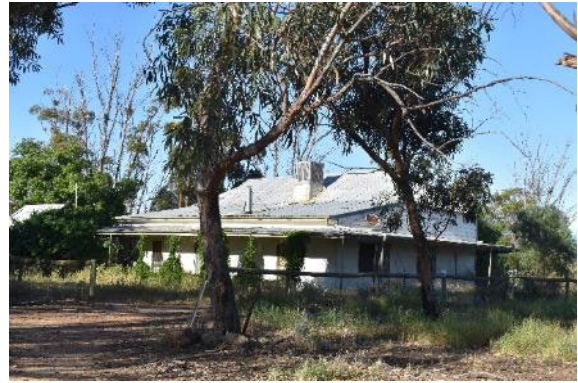
PHOTOGRAPH 5.2 EASTERN ELEVATION OF MAIN RESIDENCE AT PROPERTY (ERM 2024)
