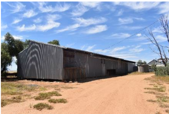
PHOTOGRAPH 5.3 VIEW EAST OF SHEARING SHED TO NORTH OF MAIN RESIDENCE (ERM 2024)
