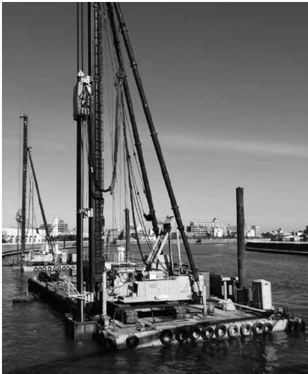
Figure 7: Barge mounted deep soil mixing equipment (Taguchi, 2015)
