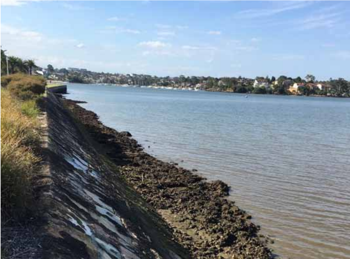
Figure 4.5. View of sloped seawall in Southern Remediation Area.
