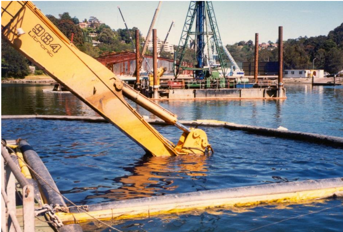
Figure 24: Excavation within a silt curtain enclosure
