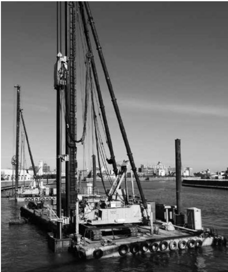
Figure 9.6. Barge-mounted deep sediment mixing
