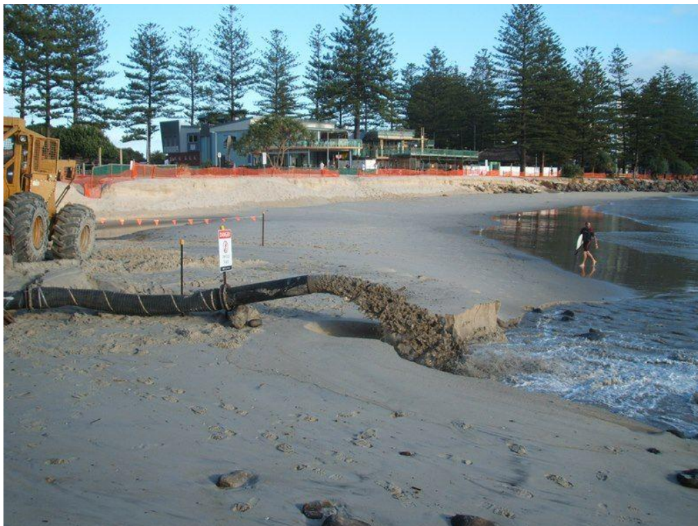
Figure 18: Hydraulic sand placement on beach area with small pipeline
