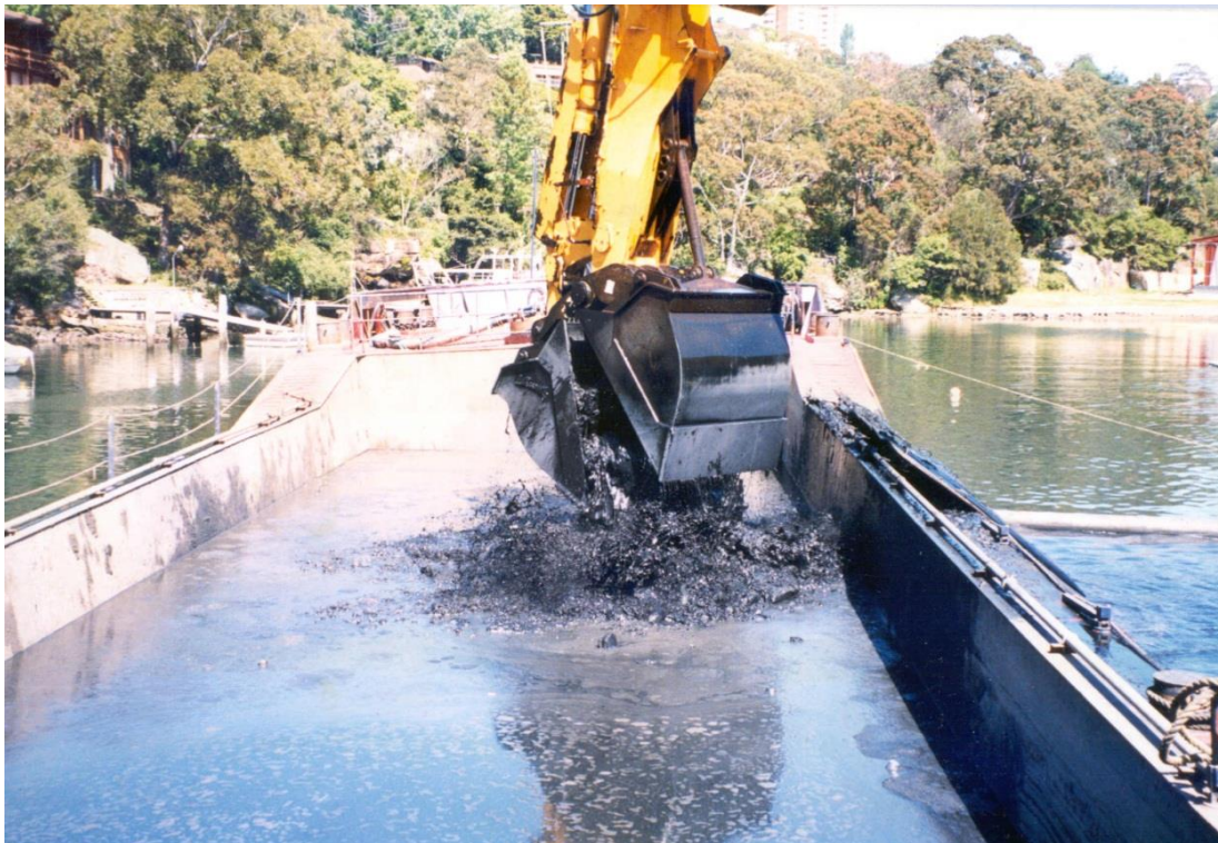
Figure 25: Hydraulically controlled environmental clamshell attachment
