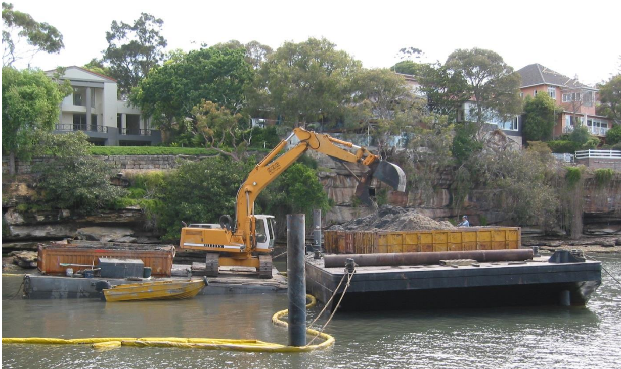
Figure 10: Barge mounted excavator loading material into a large skip bin
