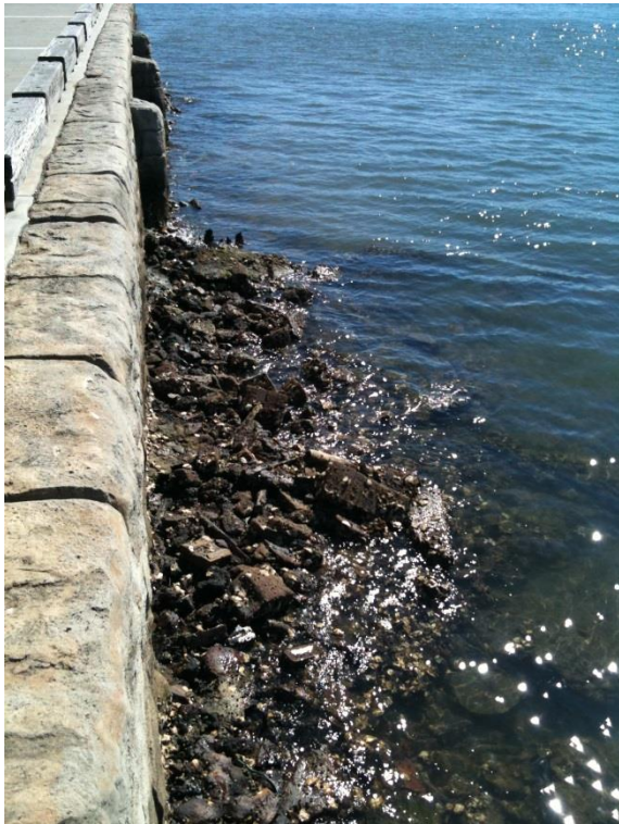
Figure 3: Vertical seawall along western side of Kendall Bay
