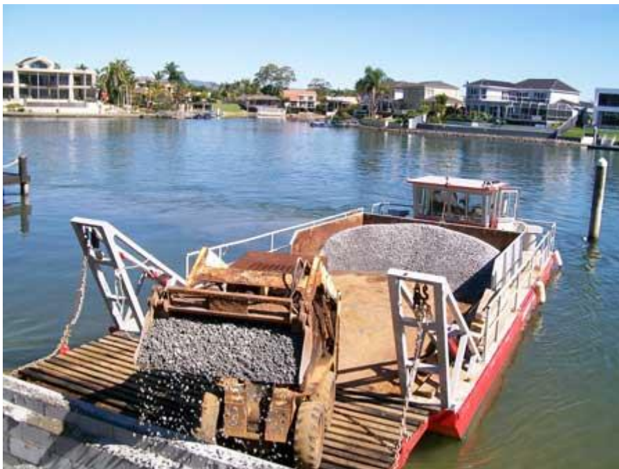
Figure 11: Small excavator tipping rock from floating barge
