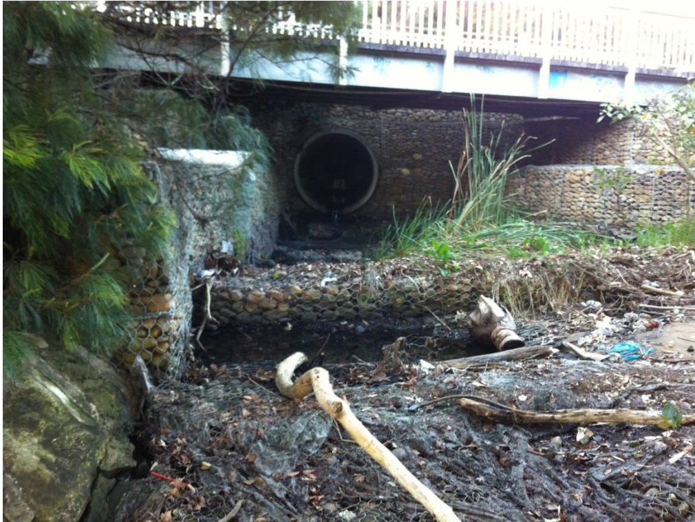
Figure 12: 1650mm diameter stormwater outlet behind the mangroves at the head of Kendall Bay (July 2016)
