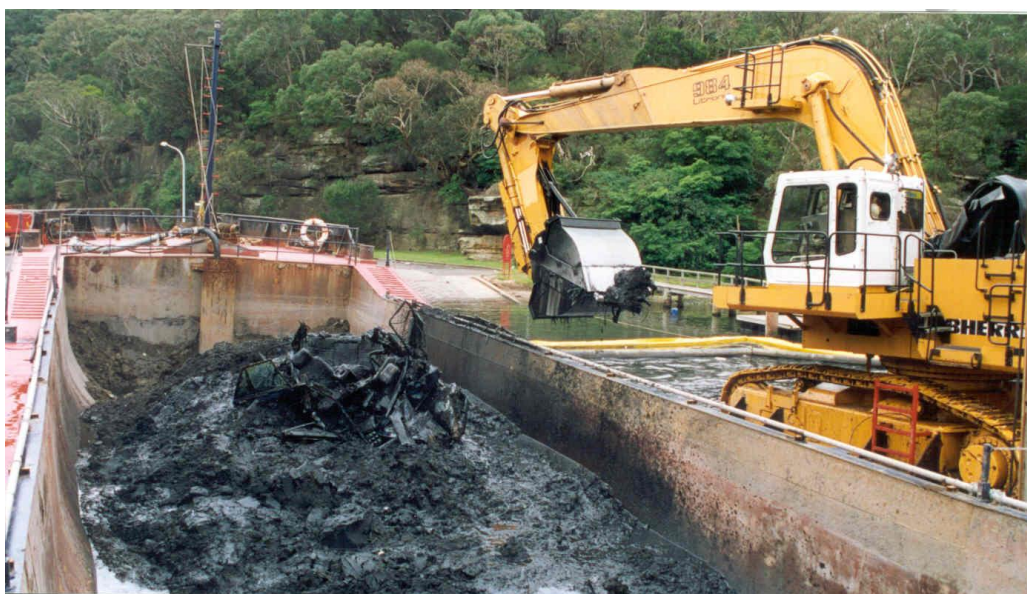
Figure 9: Barge mounted excavator loading into a hopper barge
