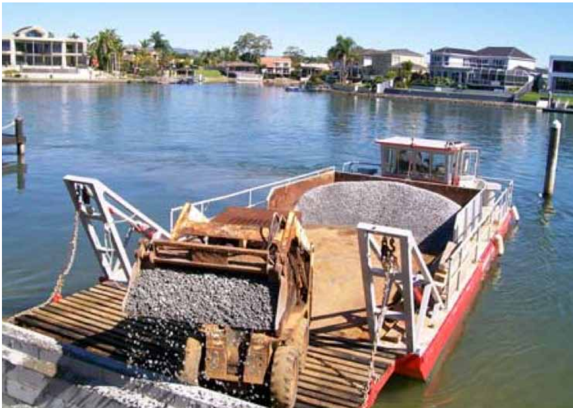
Figure 9.8. Small excavator tipping rock from floating barge
