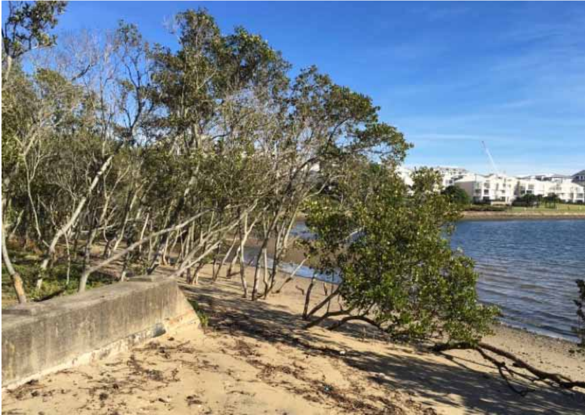
Figure 8.7. Existing cement-covered sandstone wall on western side of beach (SA4)
