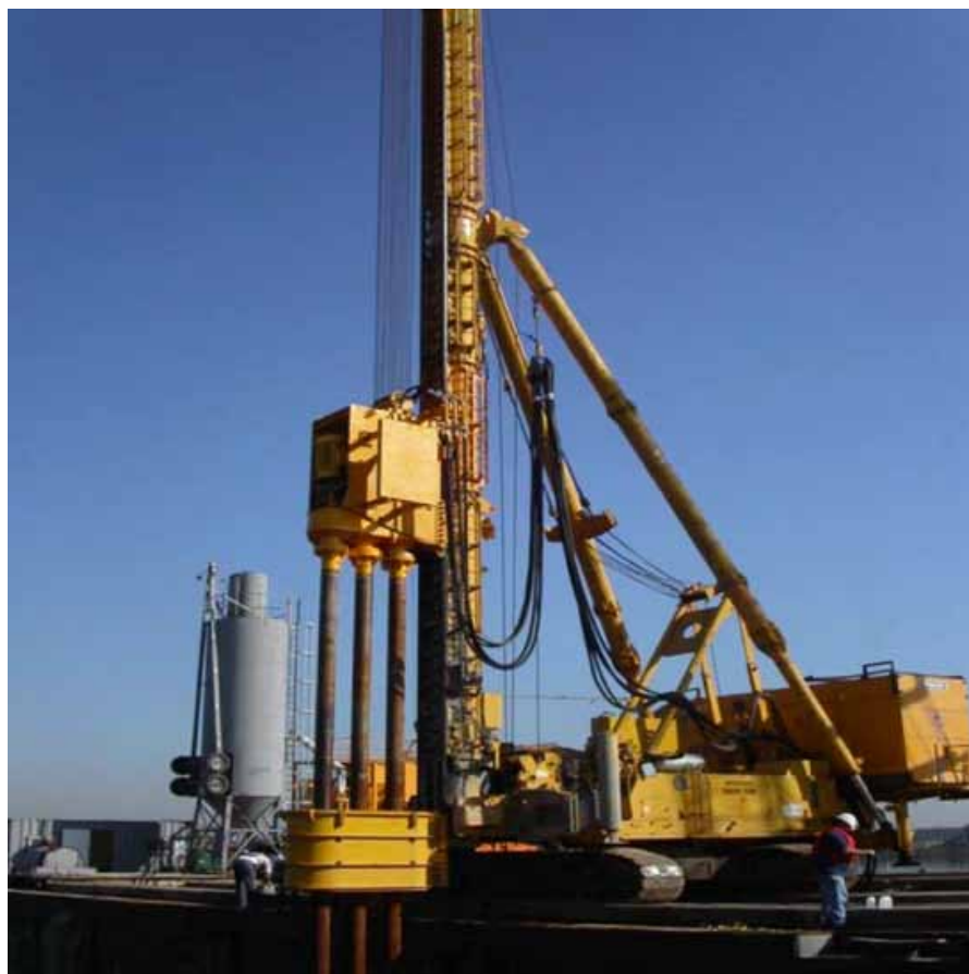
Figure 9.4. Barge-mounted drilling rig for deep sediment mixed columns
