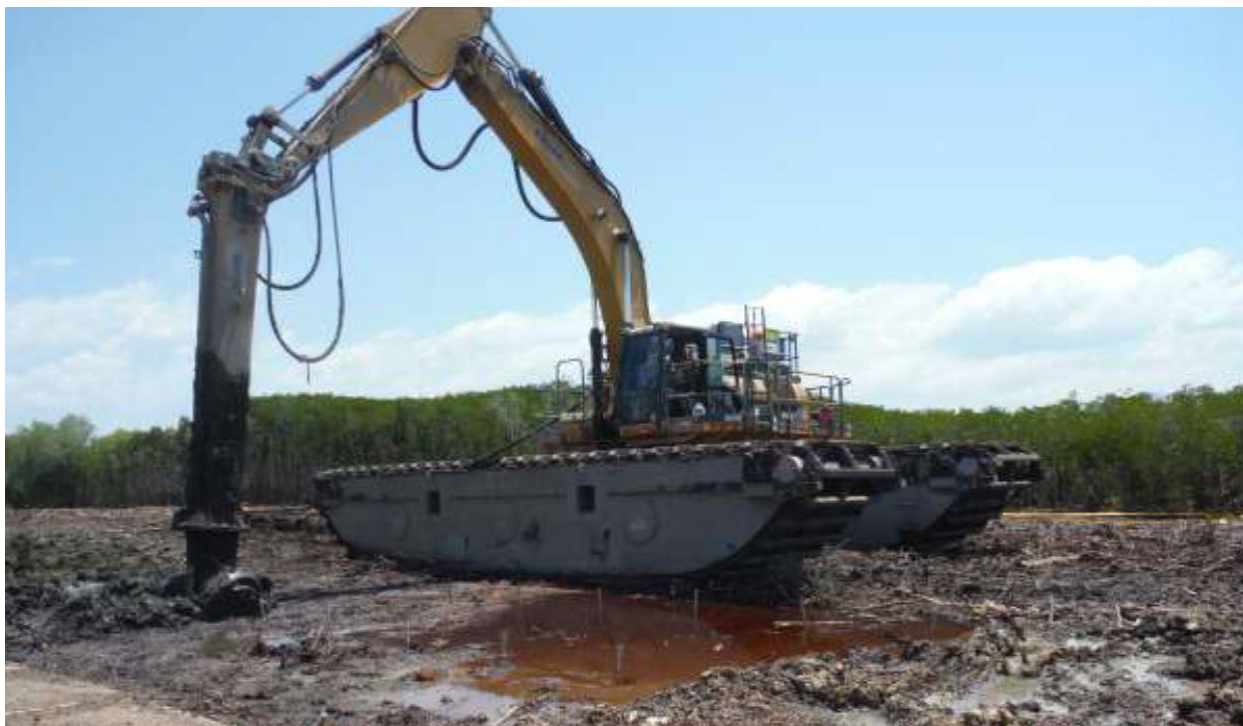
Figure 8: Amphibious excavator with mass mixing attachment (Keller Ground Engineering, 2016)
