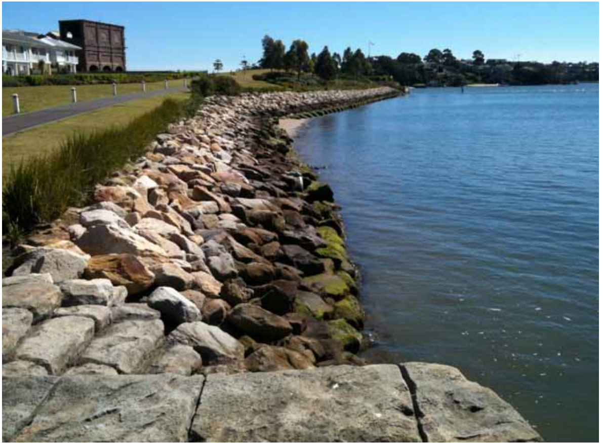
Figure 4.7 Transition between sandstone block seawall and sloping rock revetment looking north towards Breakfast Point. Note small beach midway.
