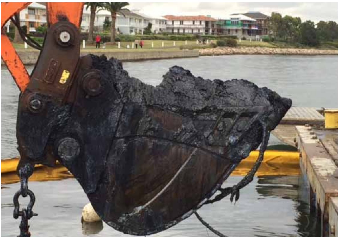
Figure 5.30. Excavator bucket full of gasworks-contaminated sediment. Note oily sheen on water within silt curtain.
