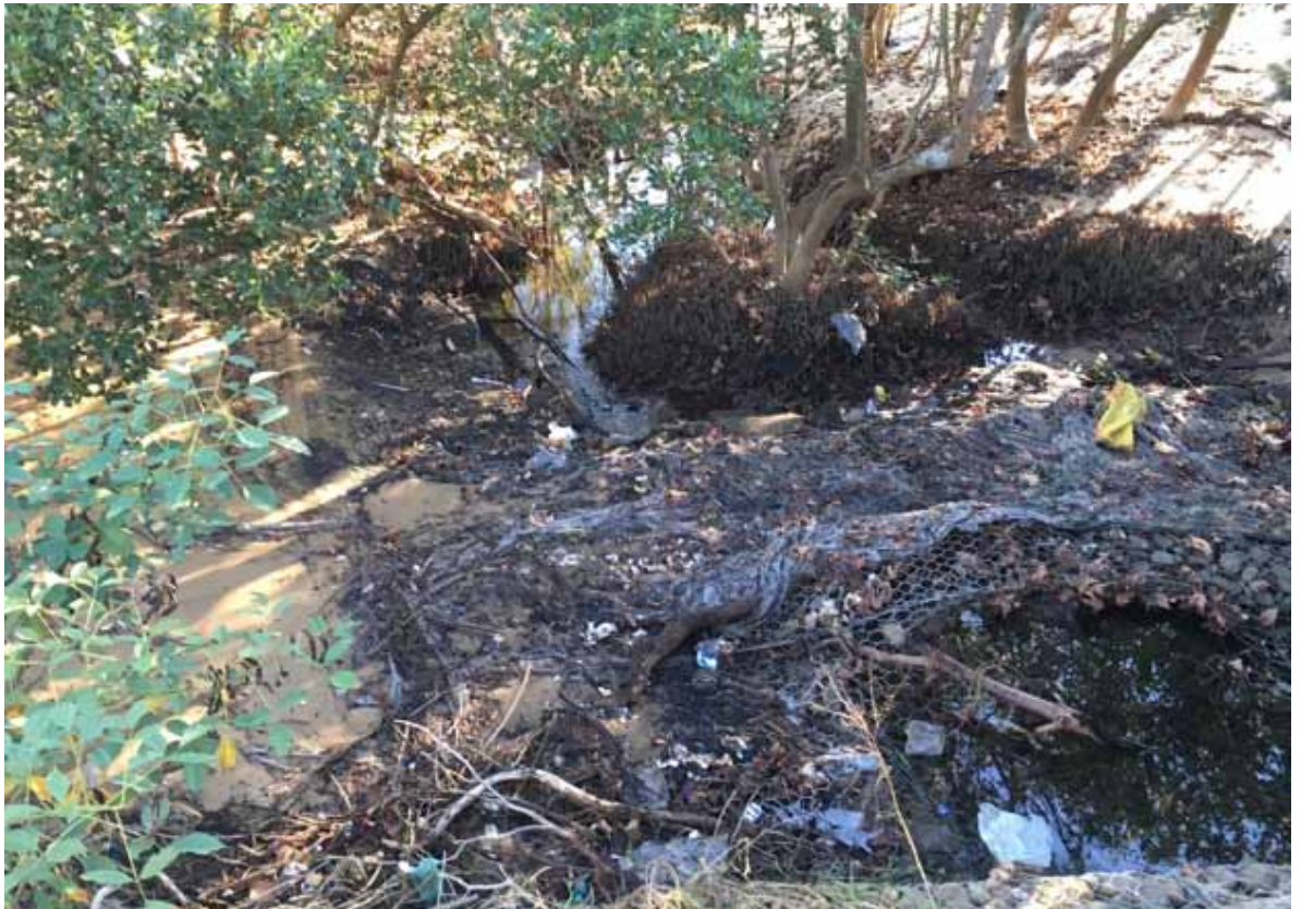
Figure 4.14. Erosion around mangroves below stormwater outlet after major storm event, June 2016 (Remediation Area SA 3)
