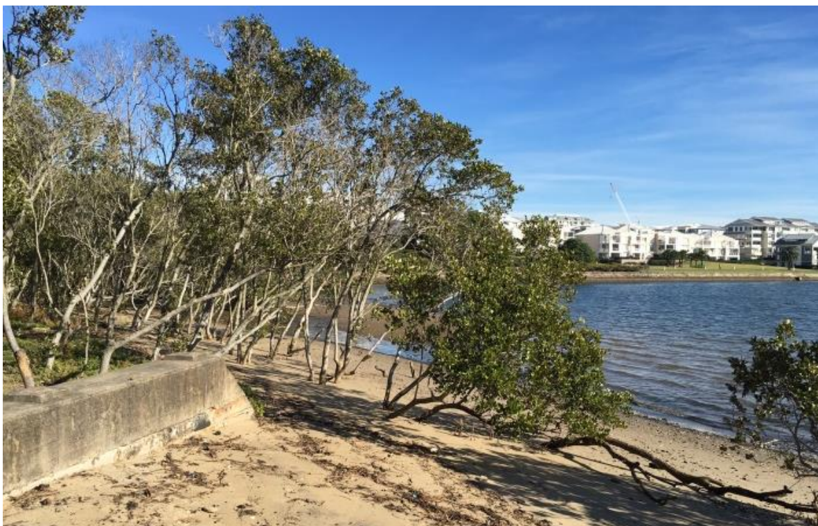
Figure 21: Existing sandstone wall on western side of beach area
