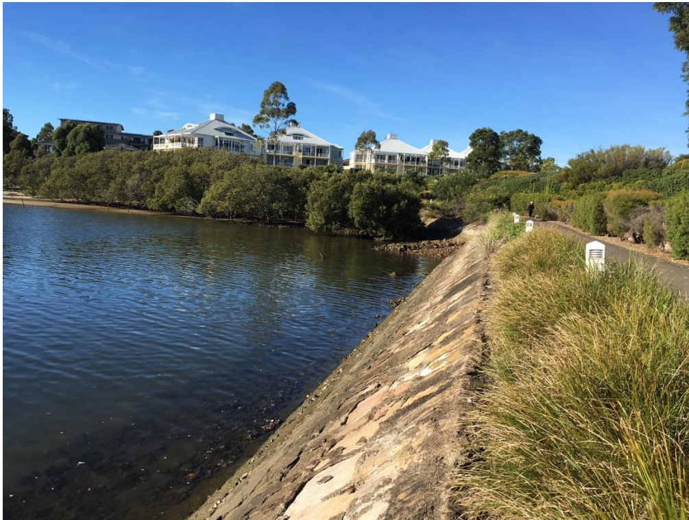
Figure 2: Sloped seawall along western side of Kendall Bay
