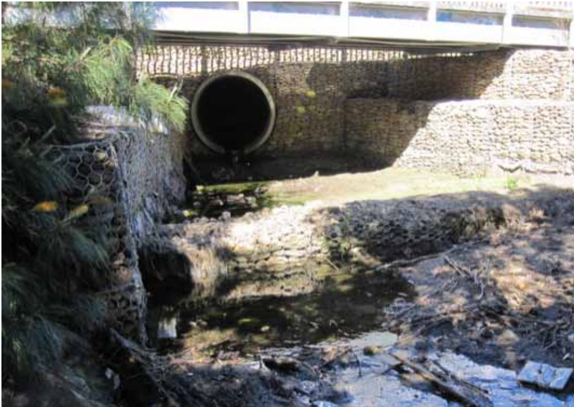
Figure 4.12. 1650 mm stormwater outlet at the head of Kendall Bay
