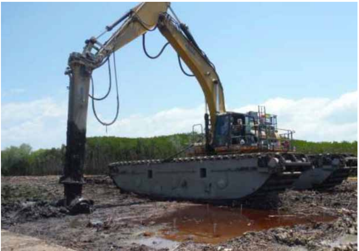
Figure 9.7. Amphibious excavator with mass mixing attachment
