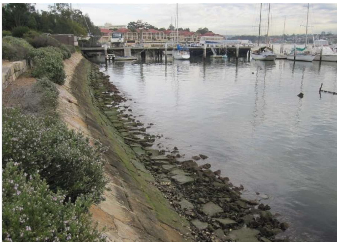
Plate 10-8: Sloped revetment within Fairmile Cove (looking towards proposed Staging Site). (Source: RHDHV, 2018a)
