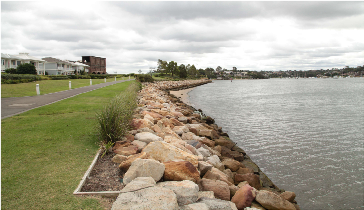
Plate 12-4: Looking north to Breakfast Point along man-made sea walls. (Source: Jemena 2018)
