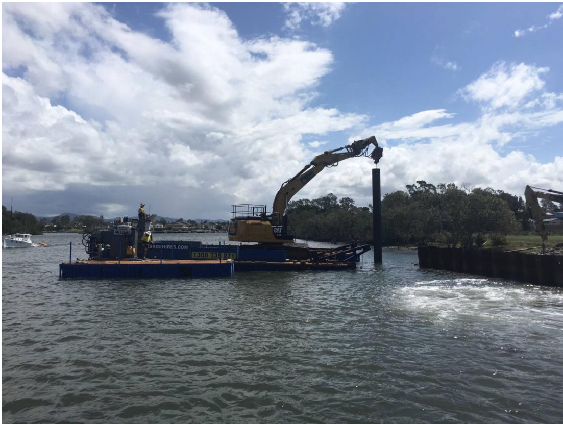
Plate 4-7: Example of barge mounted 30t excavator and sheet piles. (Source: EnviroMarine Services 2018)
