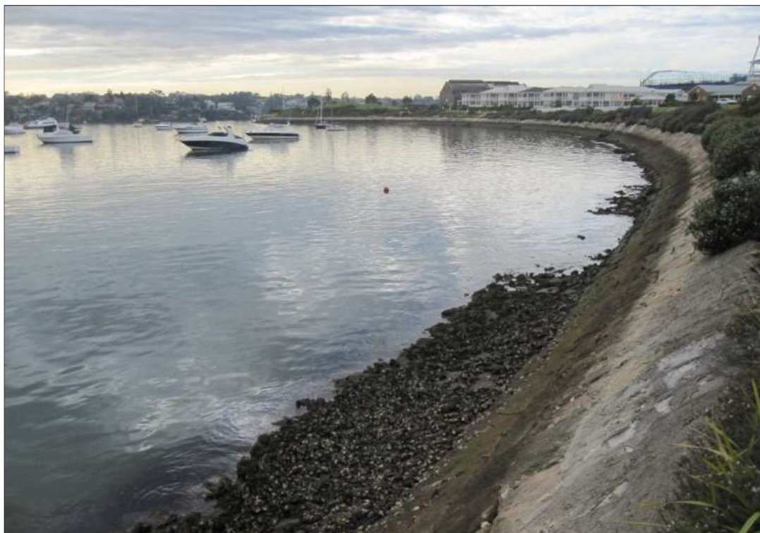
Plate 10-7: Sloped revetment within Fairmile Cove looking towards Breakfast Point. (Source: RHDHV, 2018a)
