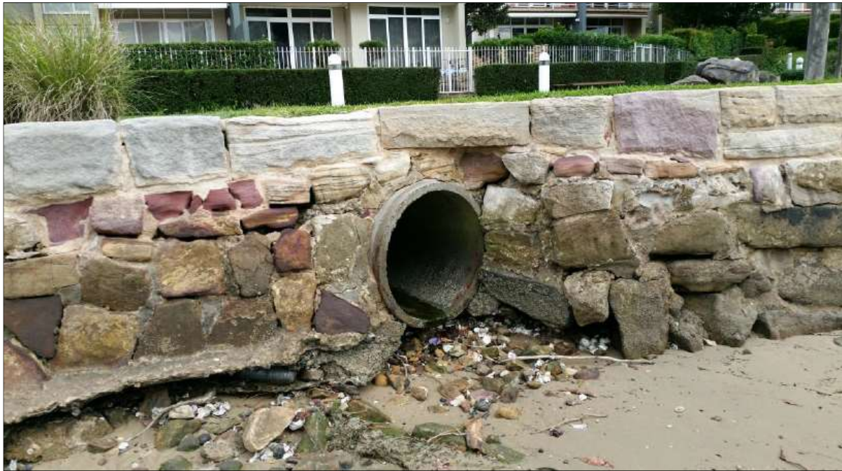
Plate 10-12: 670mm diameter stormwater outlet within Remediation Area SA4. (Source: RHDHV 2018a)
