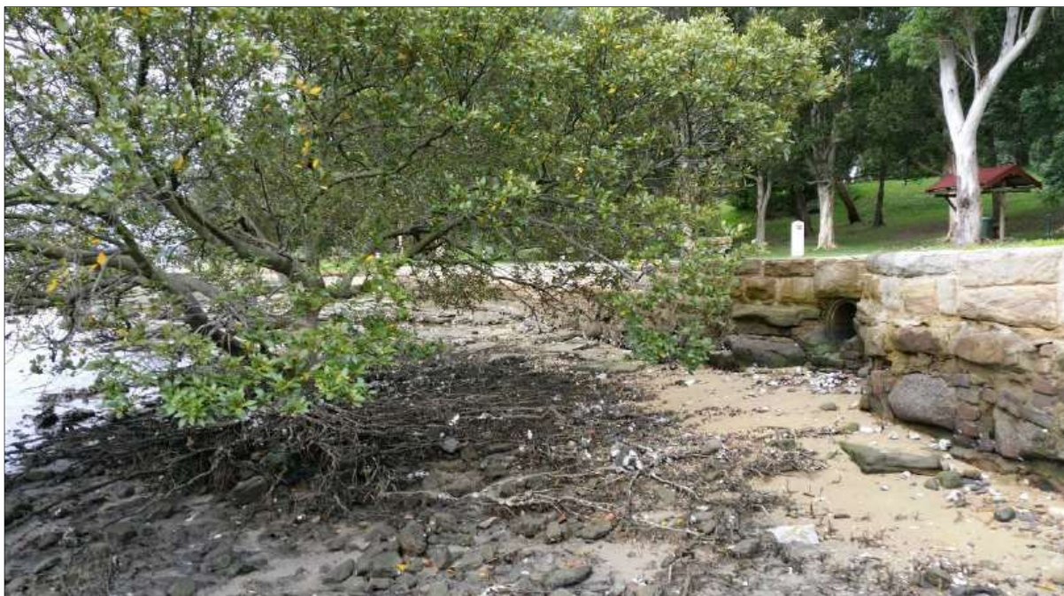
Plate 10-11: 450mm diameter stormwater outlet within Remediation Area SA4. (Source: RHDHV 2018a)
