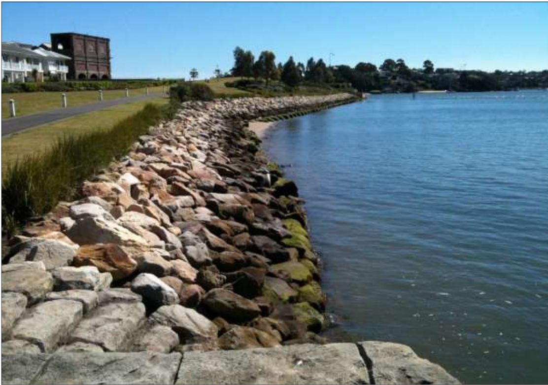
Plate 10-5: Transition between sandstone block seawall and sloping rock revetment (looking towards Breakfast Point) (Source: RHDHV, 2018a)
