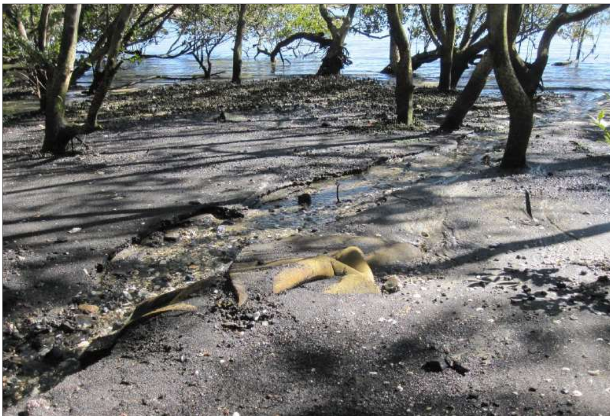
Plate 10-10: Shallow channel leading from 1650mm stormwater outlet. (Source: RHDHV 2018a)
