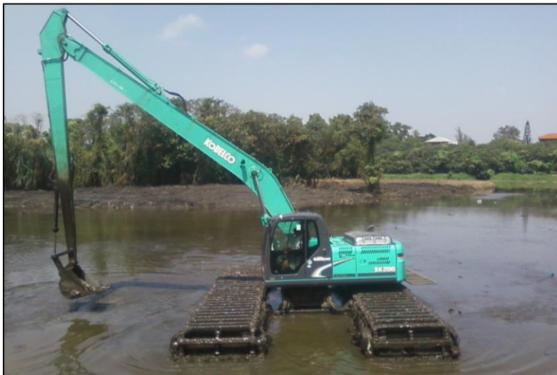
Plate 4-5: Indicative amphibious excavator (Source: Ultratrex, 2017)
