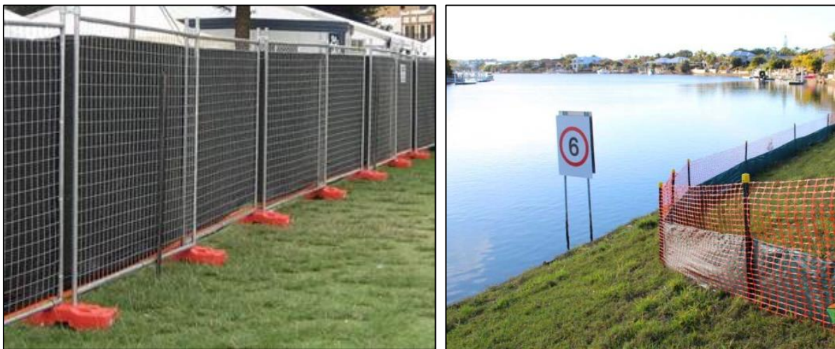
Plate 4-1: Indicative temporary screening / security fencing (Source: Aussie Erosion, 2017)
