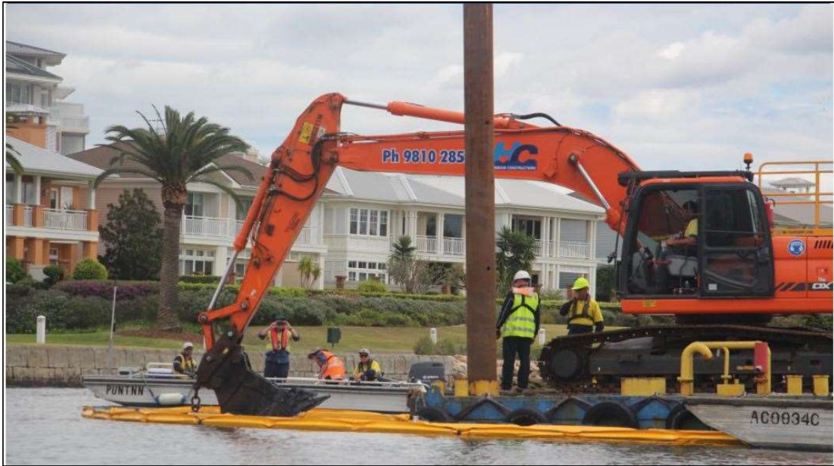
Plate 15-16: Barge mounted excavator and silt curtains used for trial
