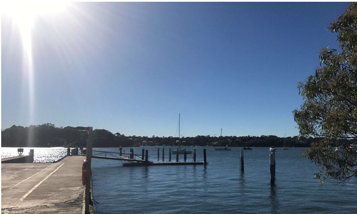
Plate 12-7: Staging Site wharf looking north. (Source: JBS&G 2017)
