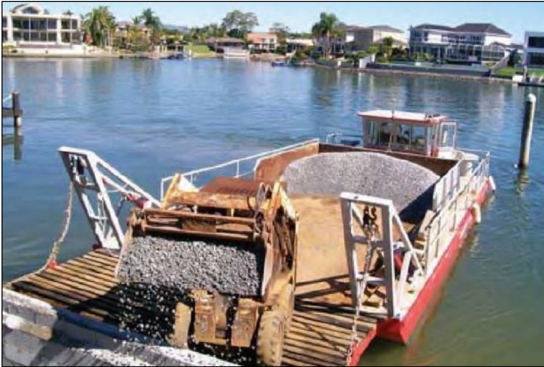
Plate 4-6: Example of small excavator tipping rock from floating barge. (Source: Jemena, 2017)
