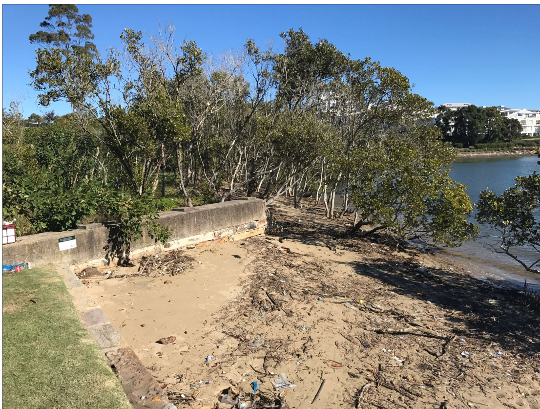
Plate 10-2: View from the eastern foreshore to the sandstone wall (Source: JBS&G, 2017)
