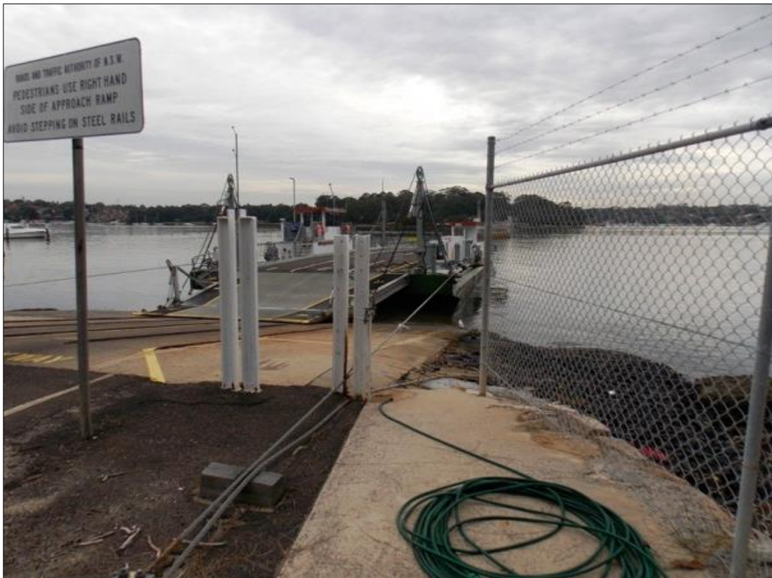
Plate 13-1: View of the Mortlake Ferry/ Putney Punt – looking north. (Source: ERM)
