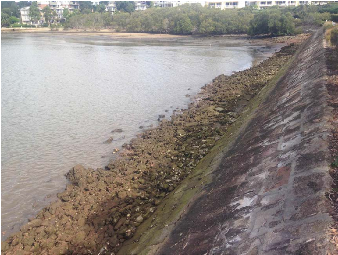
Figure 2.2. View along western seawall of Kendall Bay looking south and showing the mangroves.
