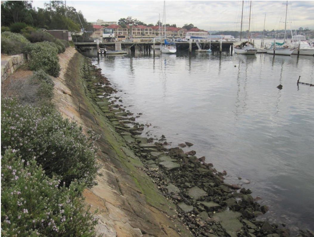
Figure 9: Sloped revetment within Fairmile Cove (looking towards the Staging Site)
