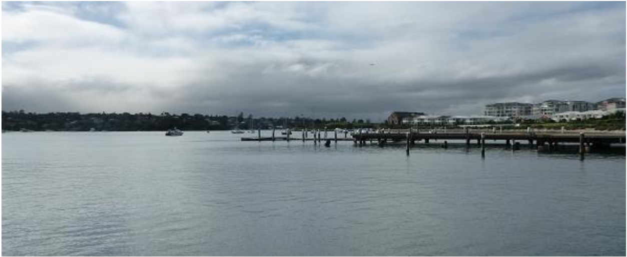
Figure 23: View of wharf structures at the old River Quays Marina (Staging Site)
