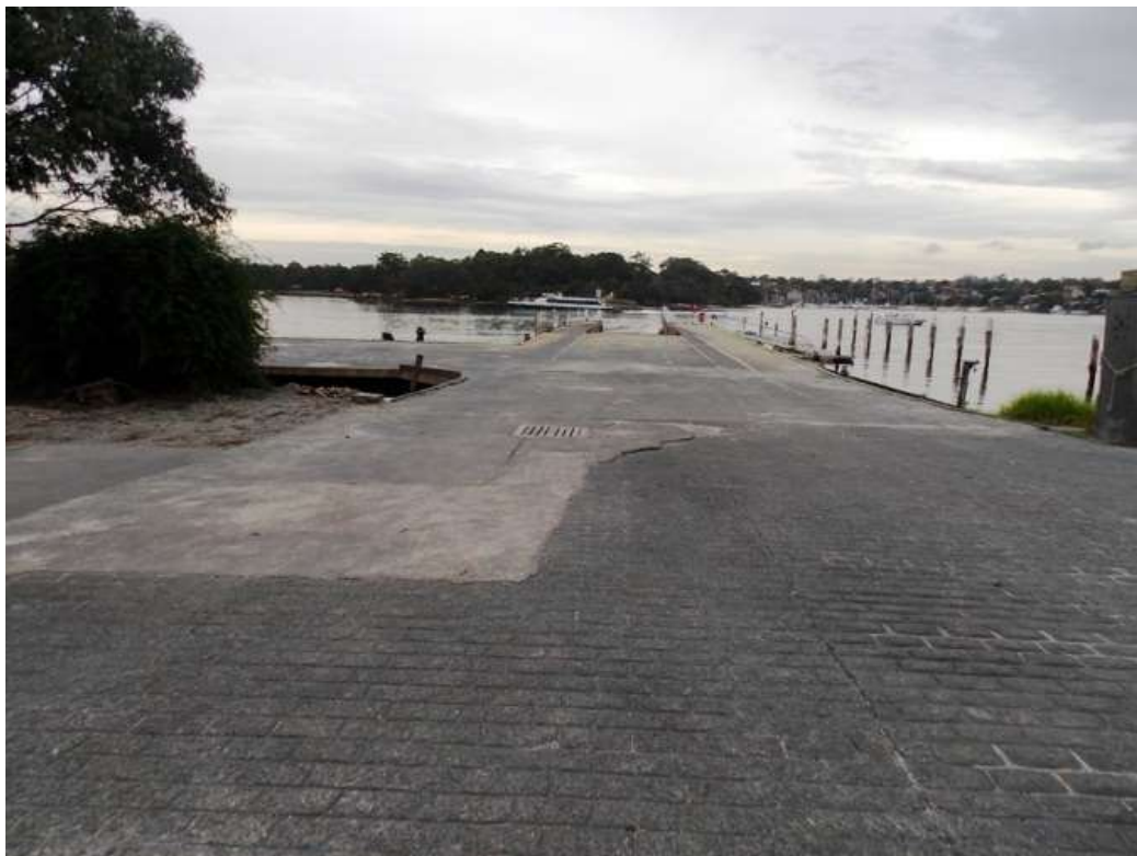
Plate 6-3: Cement and paved wharf and jetty north-east of the warehouse (ERM 2014)
