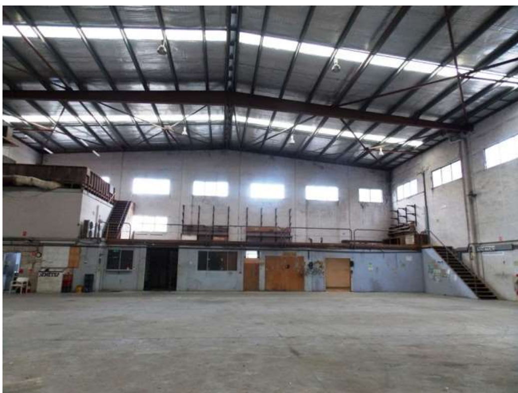
Plate 6-2: Vacant warehouse showing exposed steel framed ceiling (ERM 2014)
