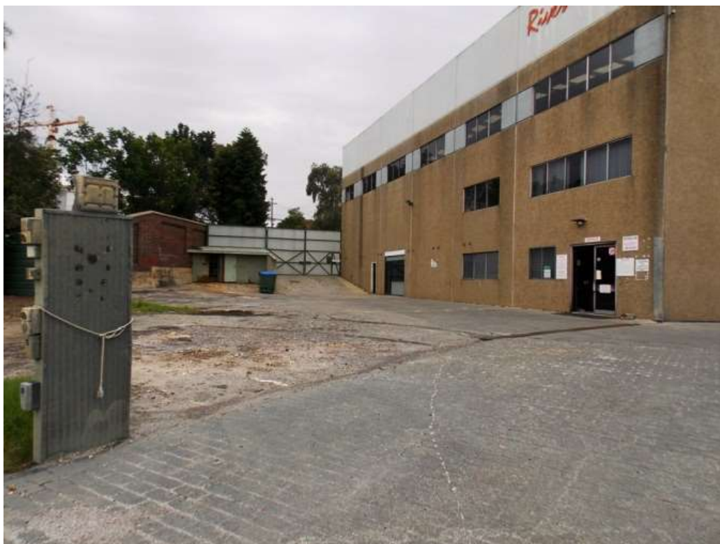
Plate 6-1: Vacant warehouse site to be used for excavated material processing (ERM 2014)
