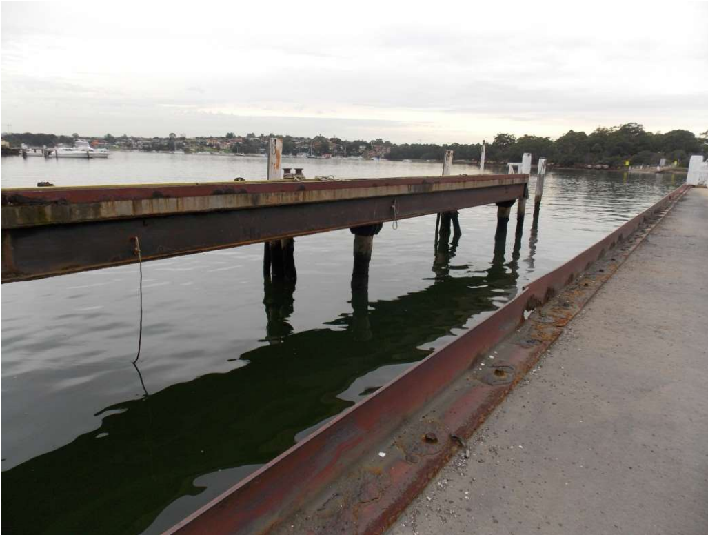
Plate 6-5: Two parallel jetties supported by timber piers (ERM 2014)
