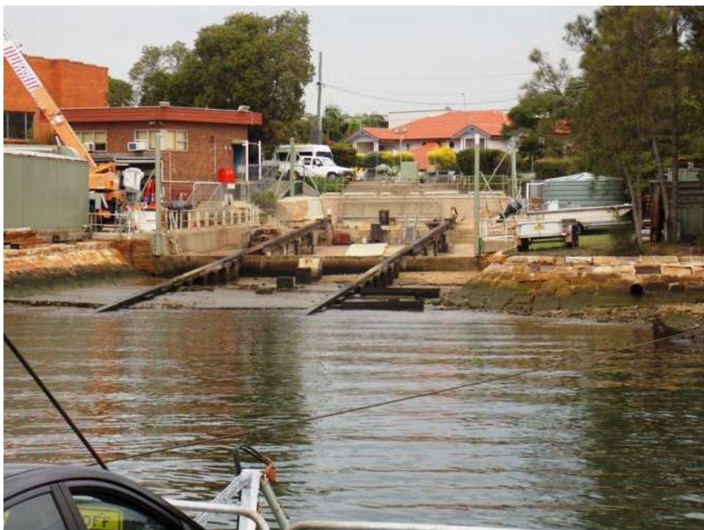
Plate 6-8: Slipway adjacent to the Mortlake Punt ramp showing sandstone block construction along the embankment (ERM 2014)
