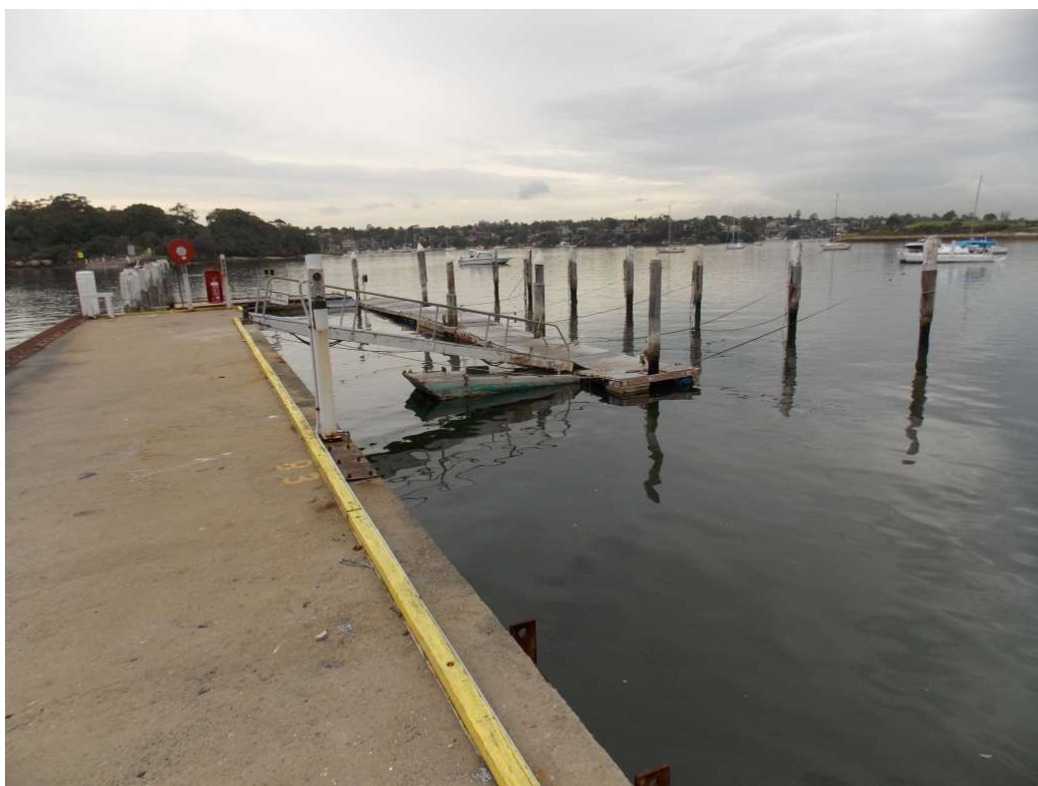
Plate 6-4: Jetty, floating pontoons and free standing timber piers (ERM 2014)
