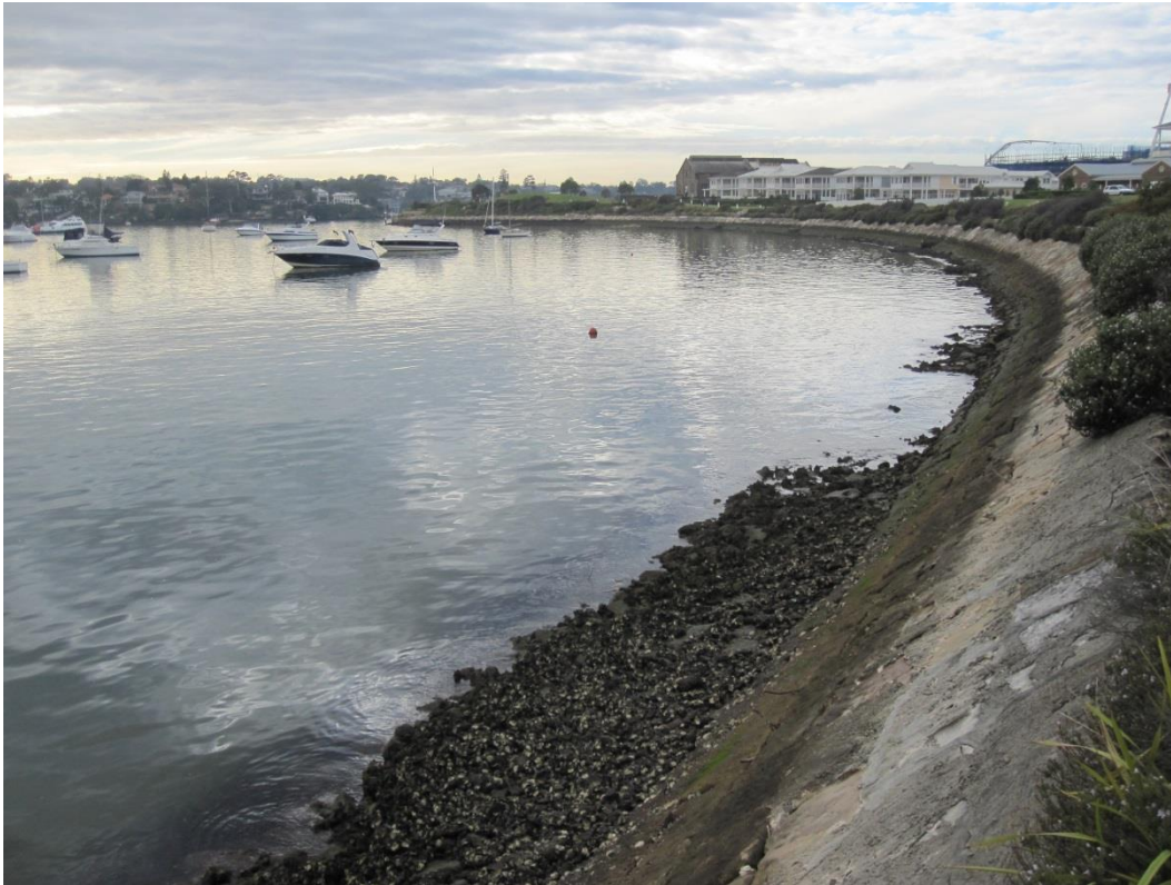
Figure 14: Sloped revetment within Fairmile Cove (looking towards Breakfast Point)
