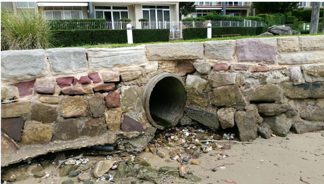
Figure 20: 670mm diameter stormwater outlet within Remediation Area SA4
