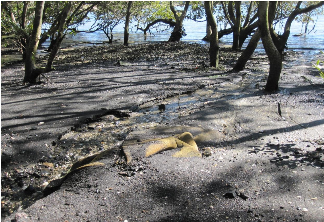
Figure 18: Shallow channel leading from 1650mm stormwater outlet
