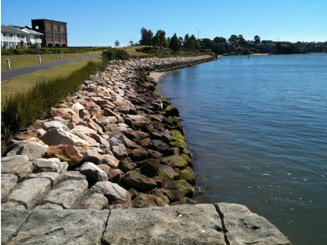
Figure 12: Transition between sandstone block seawall and sloping rock revetment (looking towards Breakfast Point)
