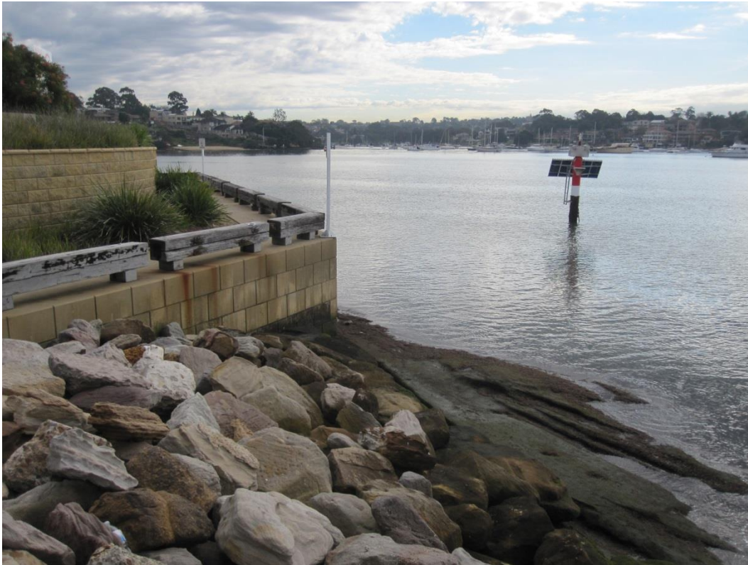
Figure 13: Vertical block seawall at Breakfast Point
