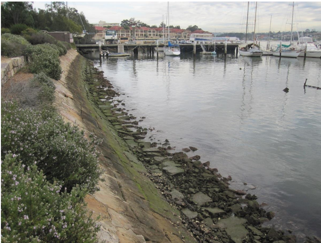
Figure 15: Sloped revetment within Fairmile Cove (looking towards the Staging Site)
