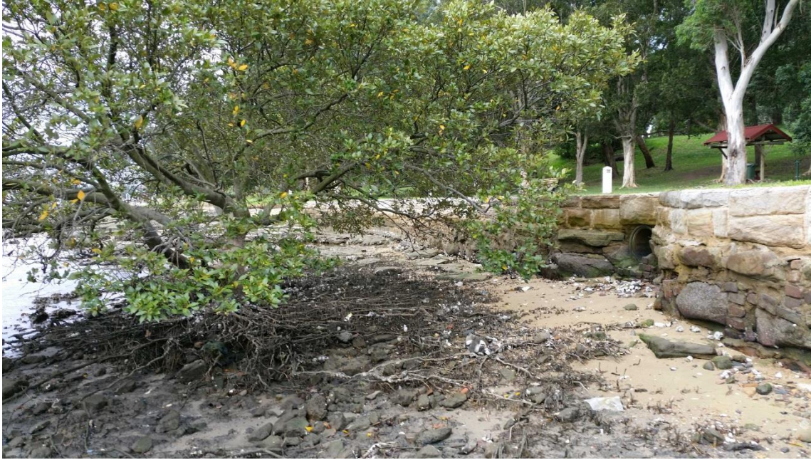
Figure 19: 450mm diameter stormwater outlet within Remediation Area SA4
