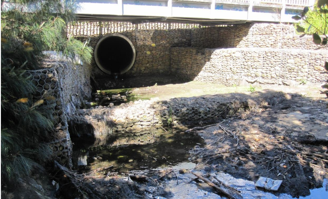
Figure 17: 1650mm stormwater outlet at the head of Kendall Bay
