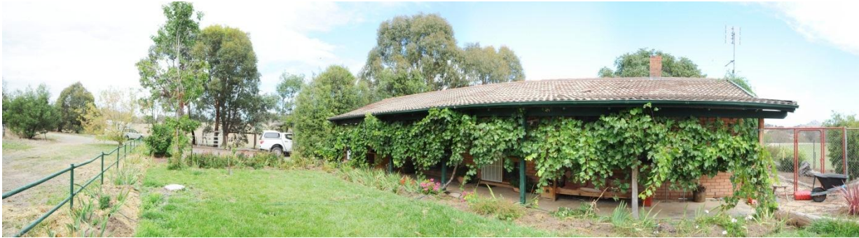
Figure 5-43 View west of Dwelling C67 from the garden (649306E, 6148460S, 447m AHD)
