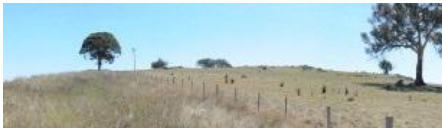
Figure 6-8 Enlarged photo showing existing power line
