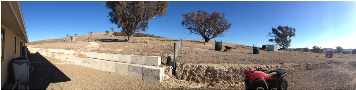
Figure 5-28 View west to rear yard of Dwelling M42 (Source YVWF)
