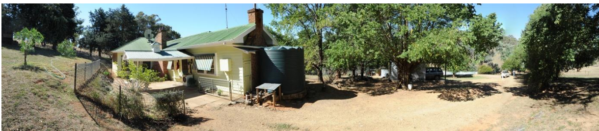
Figure 5-37 View south from driveway to the entrance of Dwelling C37 (635338E, 6159644S, 327m AHD)
