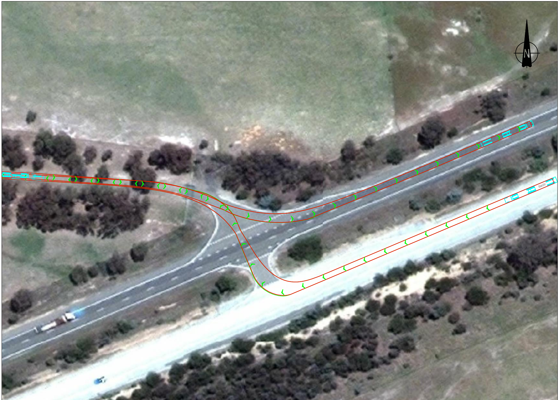
Hume Highway - Old Hume Highway. B-Double (25m)
