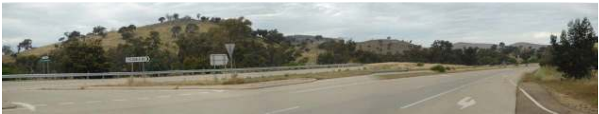
Figure 7.24 View looking north-east across the Hume Highway
