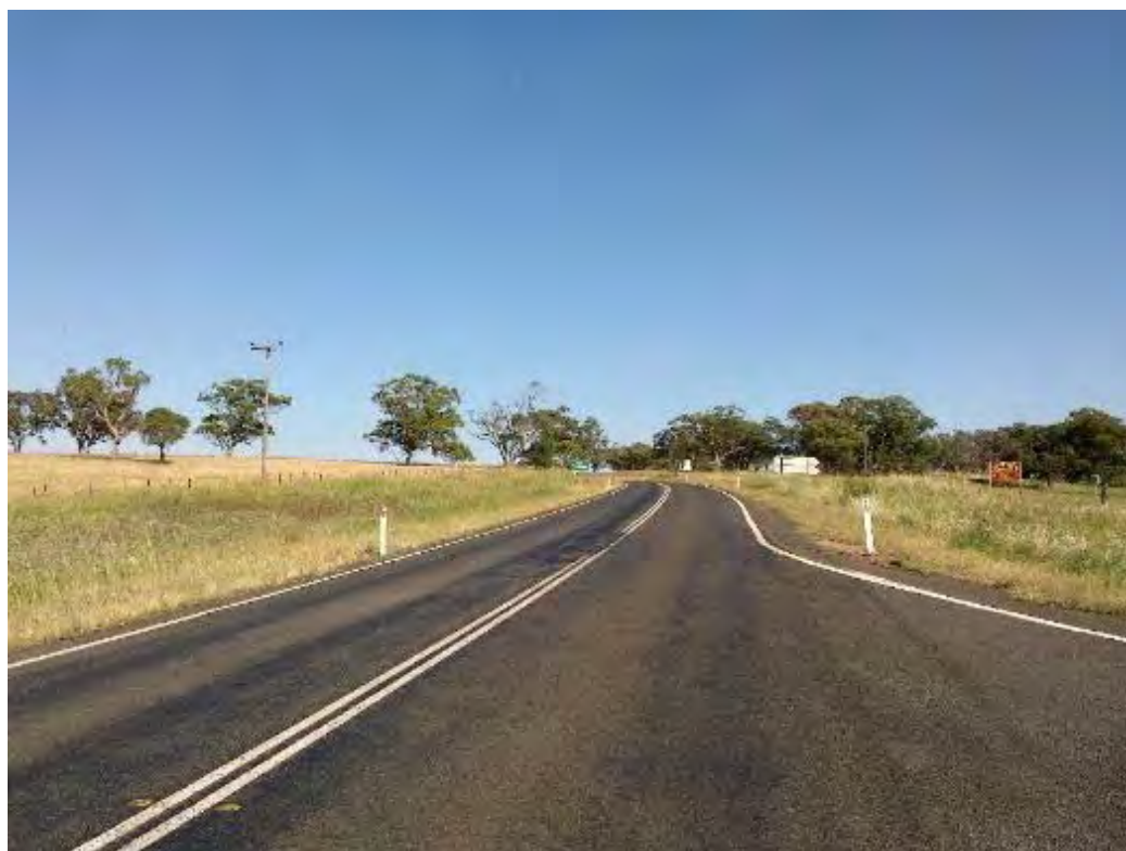
Figure 4.1.2 – View to West towards Golden Highway
