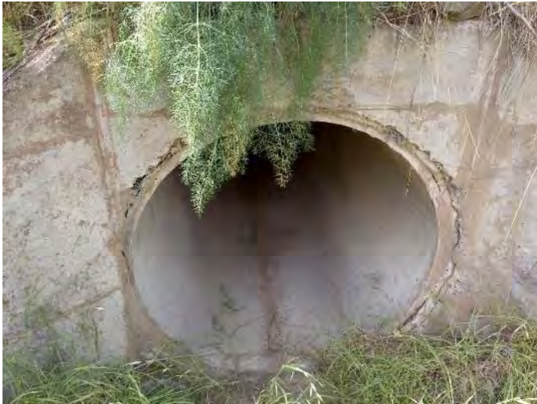
S013 – Single 1200mm Pipe Culvert
