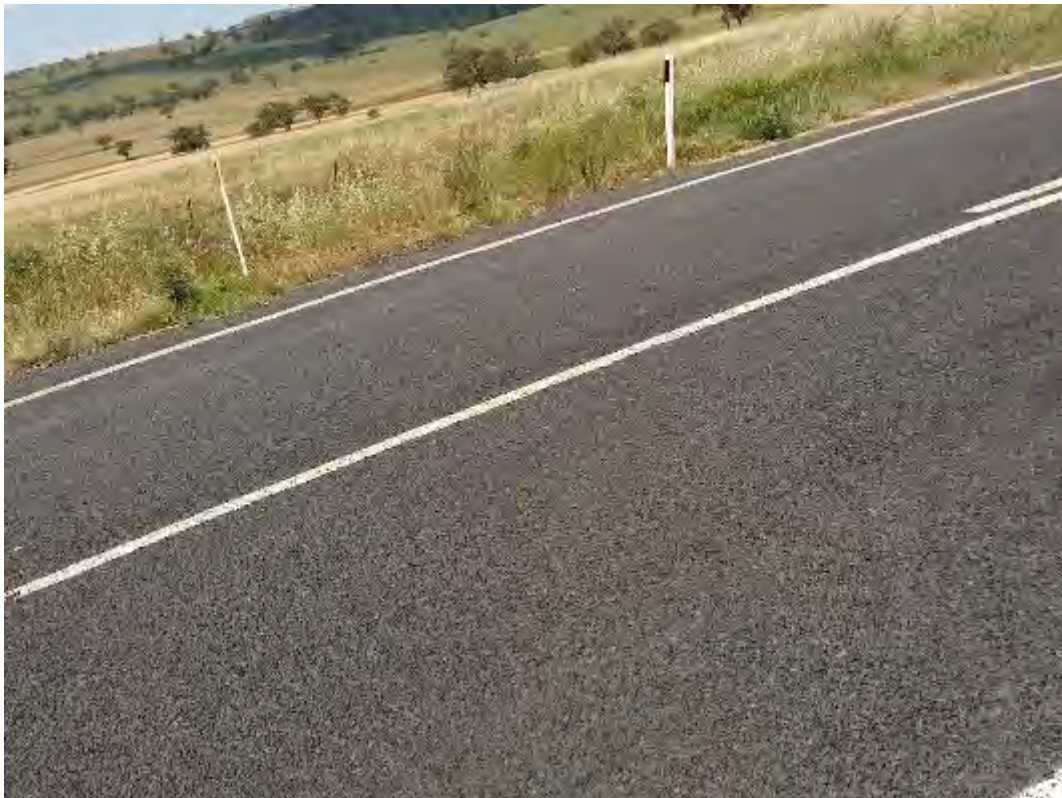
S013 – View to North
