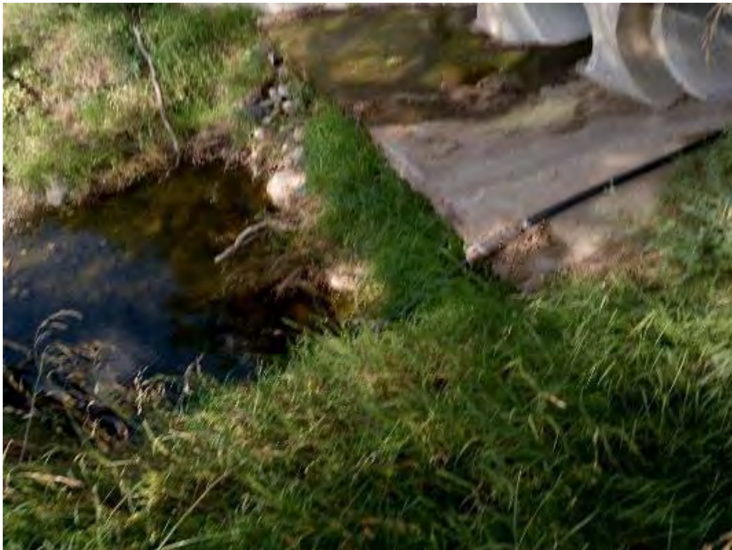
S008 – 3 × 1200mm Pipe Culvert
