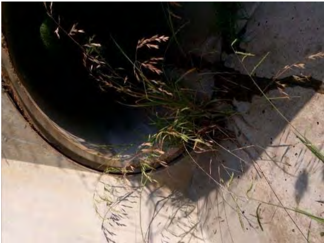
S065 – Internal View
