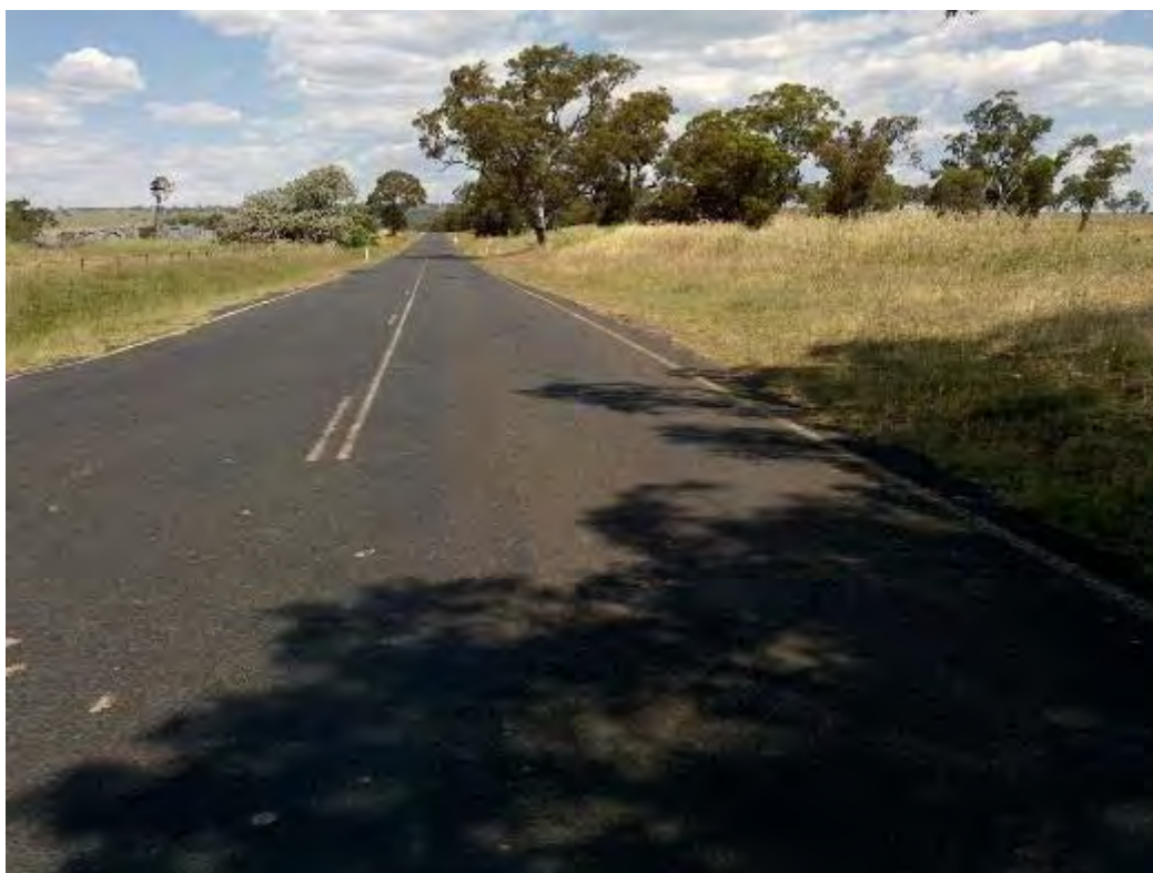
Figure 4.5.4 – View to South-East towards Vinegaroy Road
