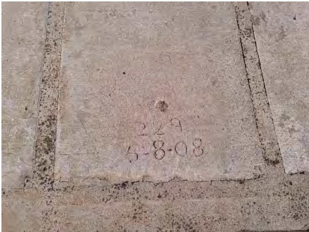
S045 – Marking showing completion date
