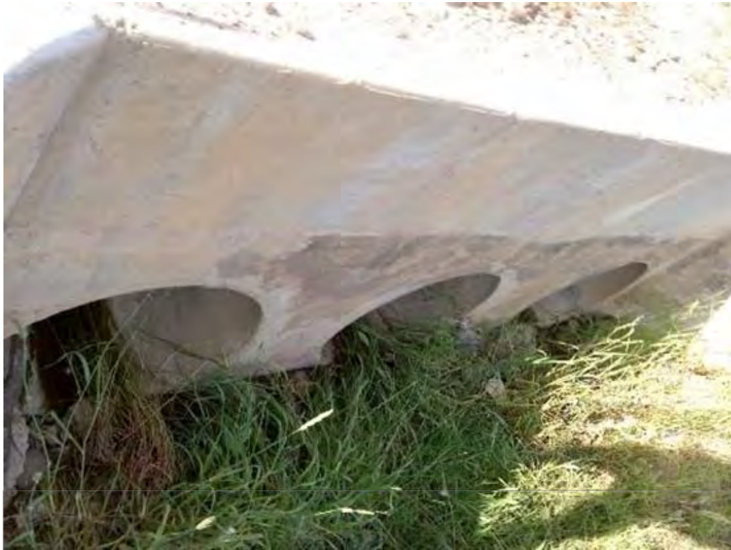
S003 – 3 - 900mm Pipe Culvert
