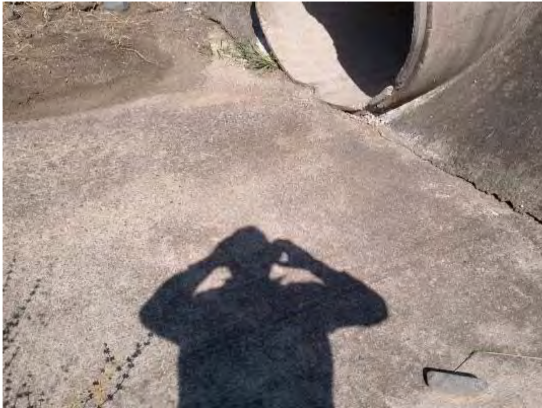
S038 - 1200mm Pipe Culvert
