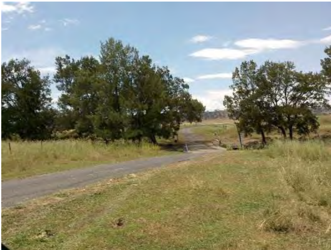
S025 – View East
