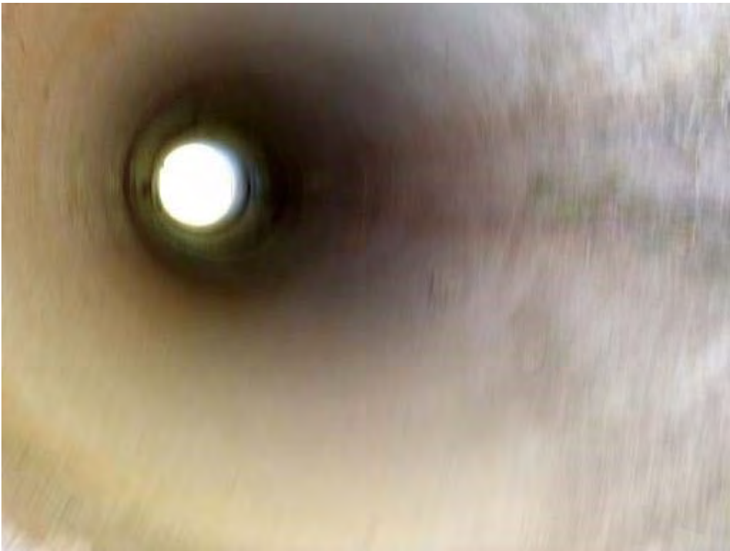
S002 – Internal View Good Condition
