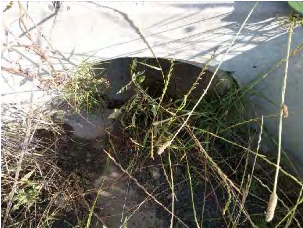
S070 - 450mm Pipe Culvert
