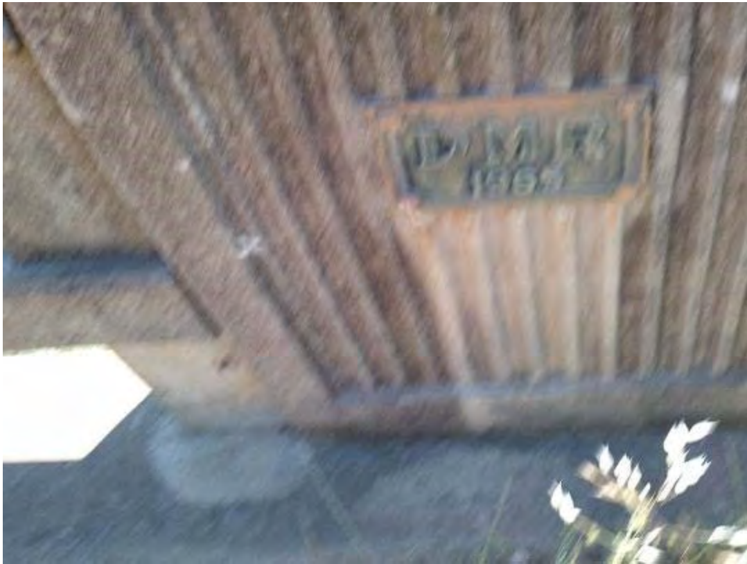
S036 – Bridge Label
