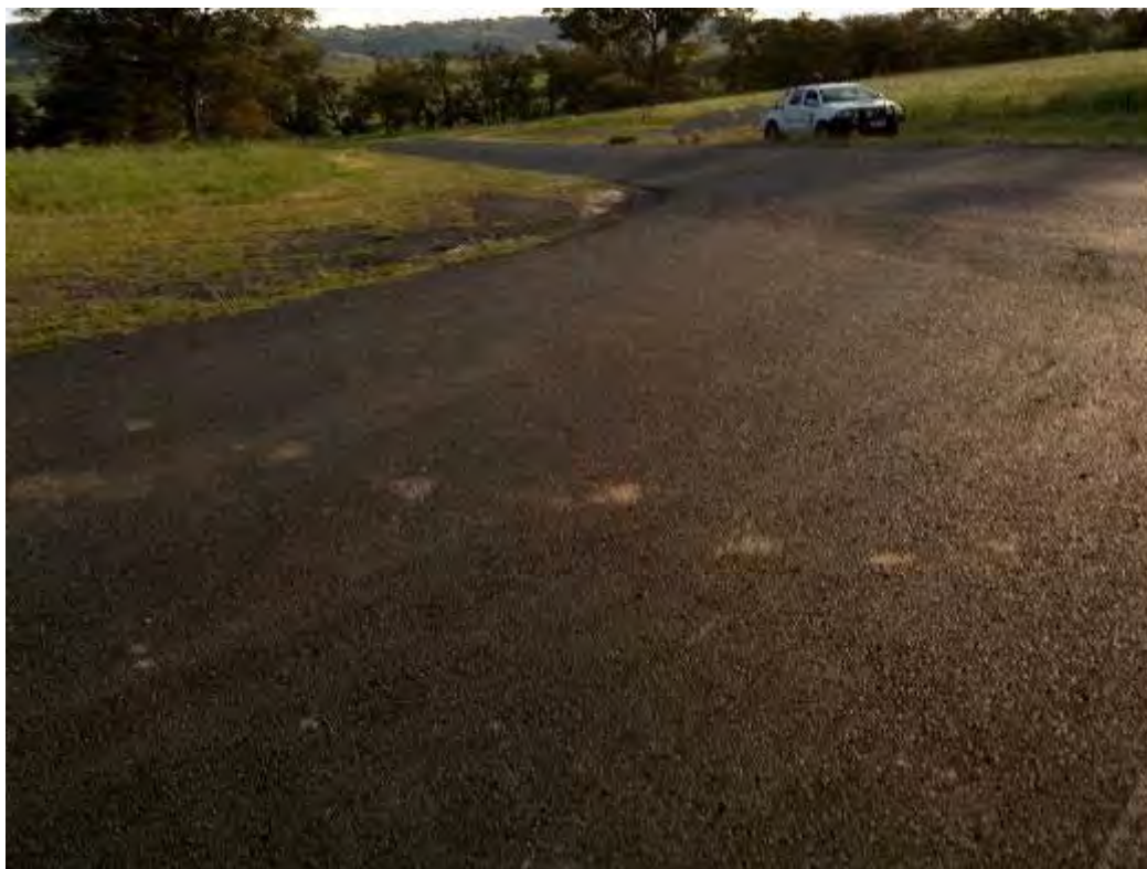
Figure 4.9.2 – View to South-West towards Coolah Creek Road
