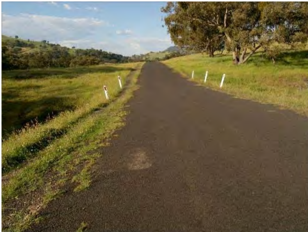
S054 – View to North
