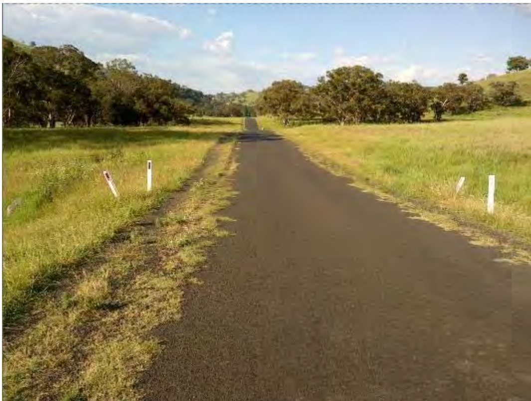
S053 – View to North
