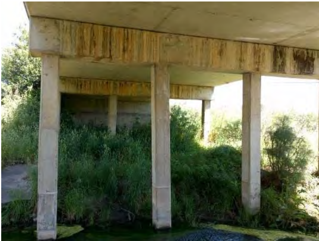
S036 – Soffit View
