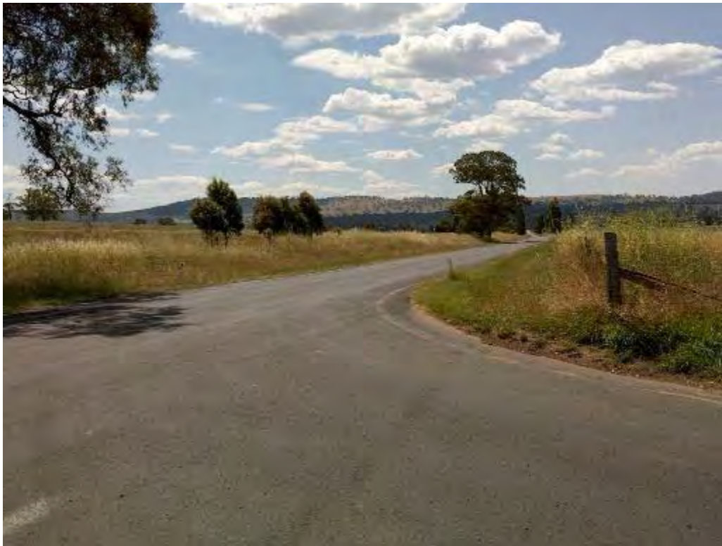
Figure 4.5.2 – View North-West towards Vinegaroy Road
