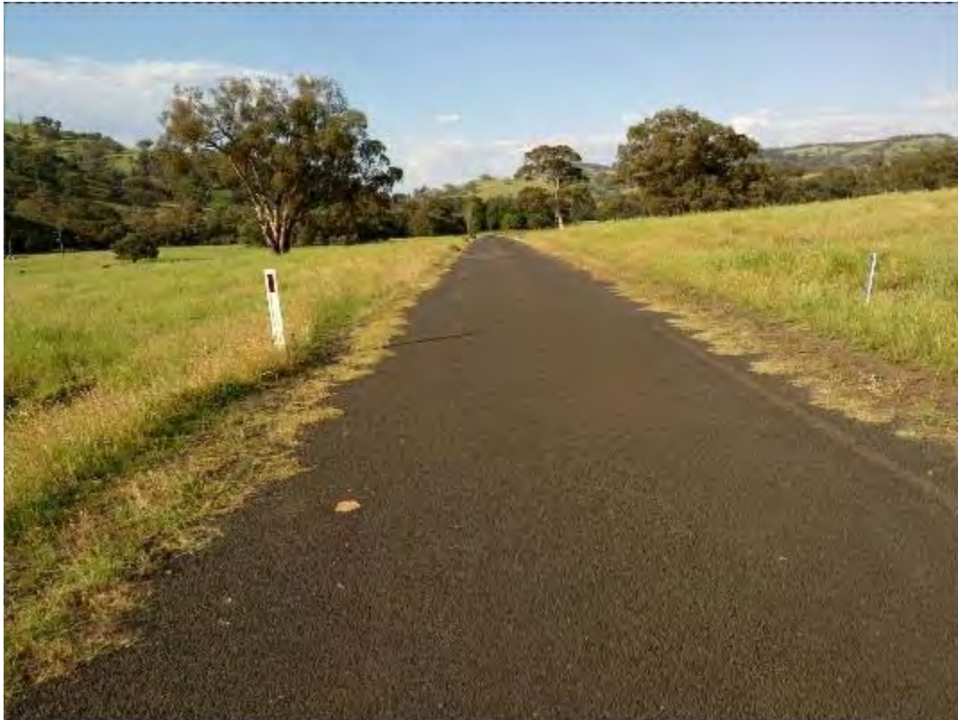
S057 – View to North
