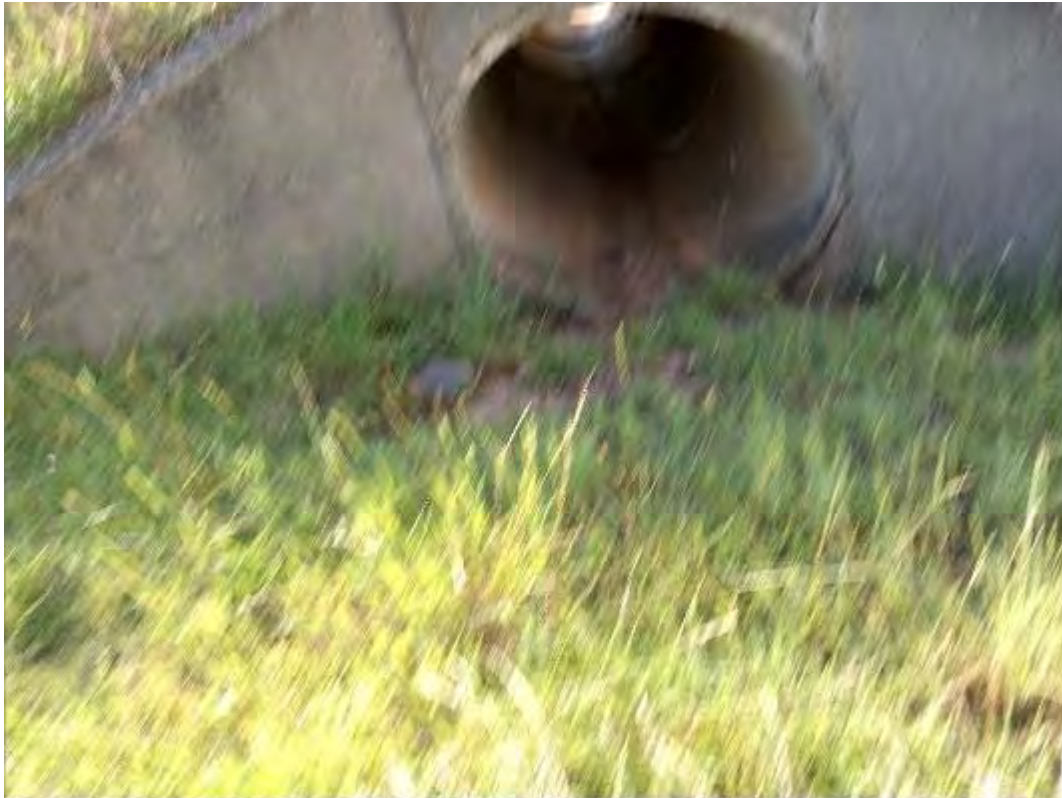
S053 – View of 1200 Pipe Culvert
