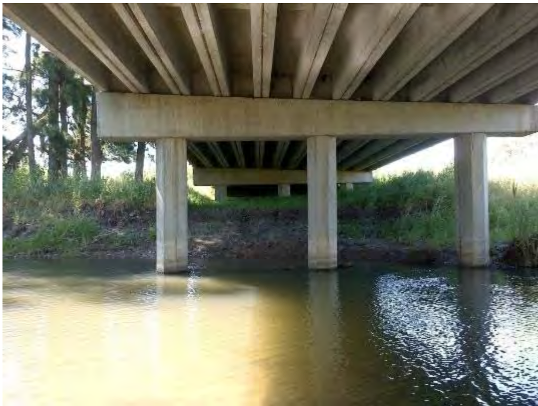
S045 – Soffit View
