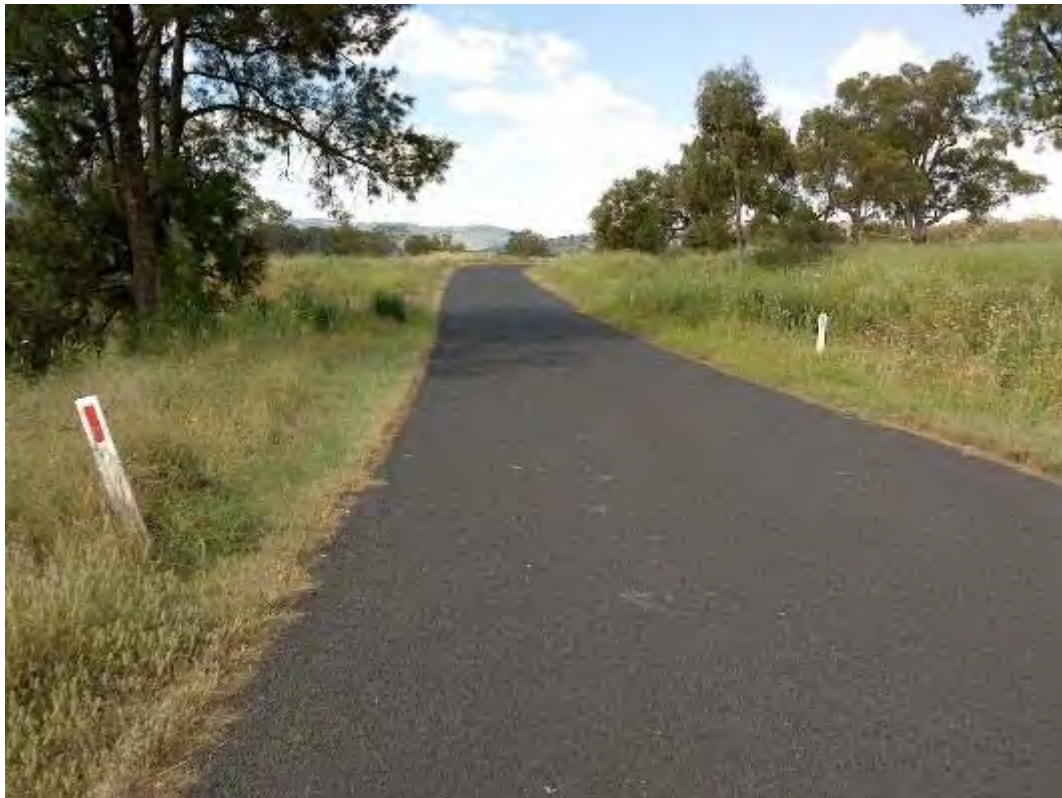
S008 – View to North
