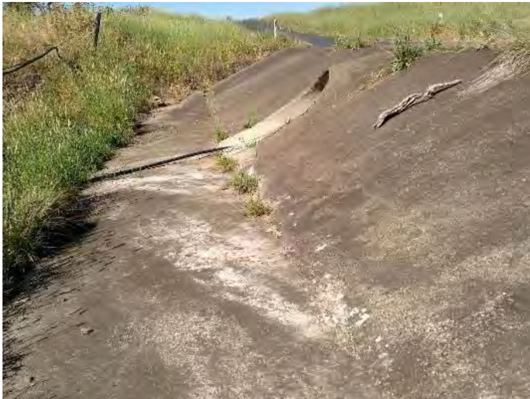
S037 – 1250mm Pipe Culvert
