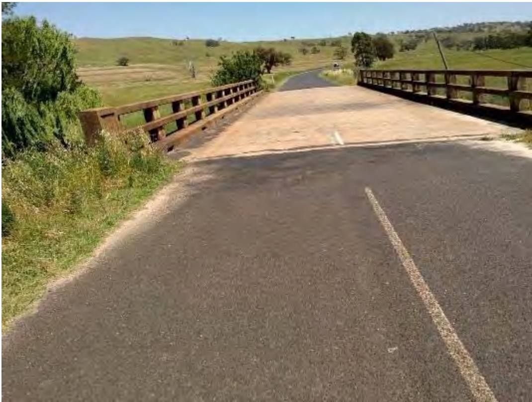
S036 – View to North
