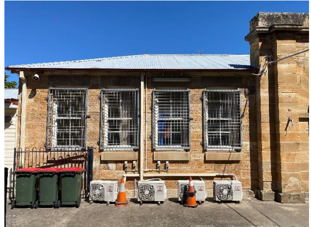
Figure 53 – South wing, constructed in 1940s with reused sandstone.
