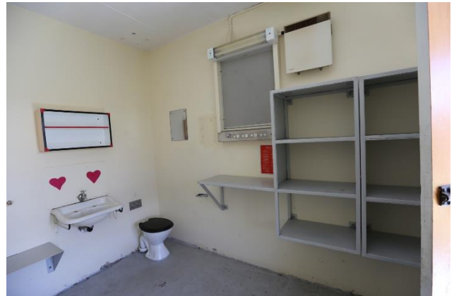
Figure 61 – Internal view of a typical cell within the eastern cell block, showing details of the amenities.
