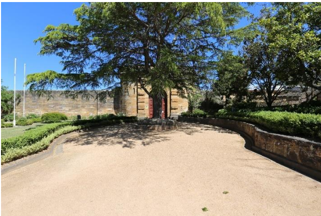
Figure 5 – View 1, principal view from Argyle Street.
