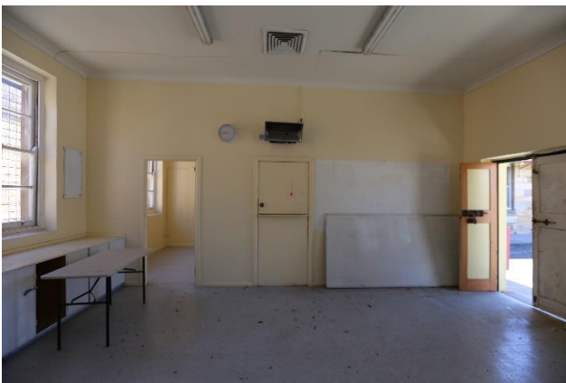
Figure 64 – Interior view of the amenities room, looking west.
