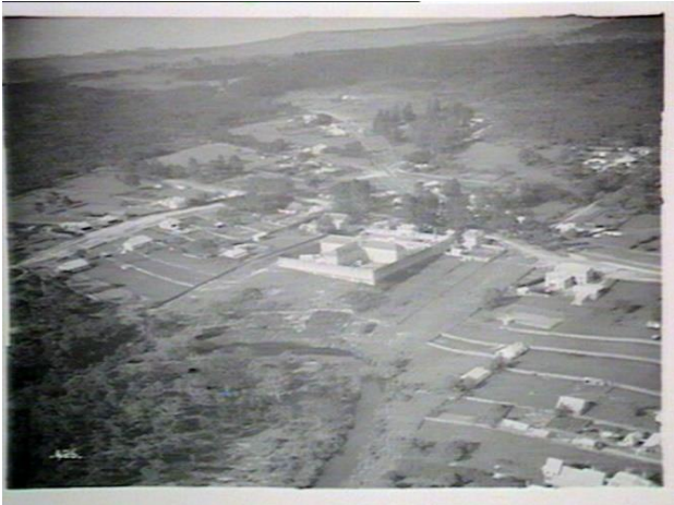
Figure A- 204 - Aerial view of Berrima Gaol, c.1930s.
