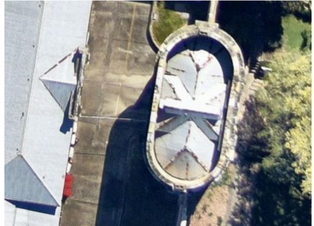
Figure 33 – Detailed aerial view of roof form and structure.
