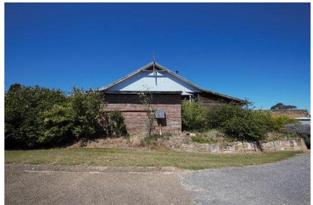
Figure 84 - The rear of garden at the northwestern section of the subject site, looking towards the rear of the Industries Building.
