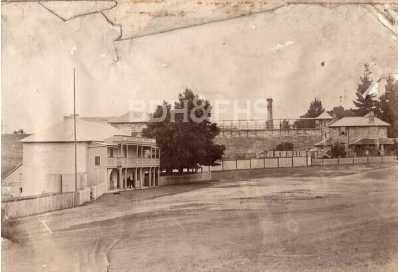
Figure 112 - The Surveyor General Inn, Berrima NSW, 1910. Note the view to the Governor's Residence, the former watch tower with catwalk and the chimney.
