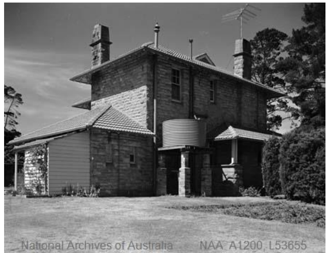
Figure 219 – Governor's Residence, 1966. View from rear.
