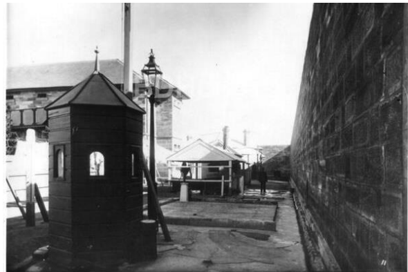
Figure A- 8 - Berrima gaol No 5 post sentry box in left foreground, wash shed in centre and large wing building, c.1897.
