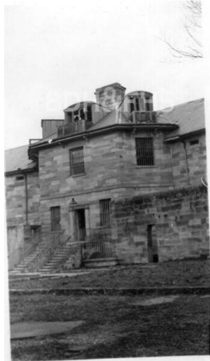
Figure A- 318 - Berrima Gaol Wing from the inside yard, undated.
