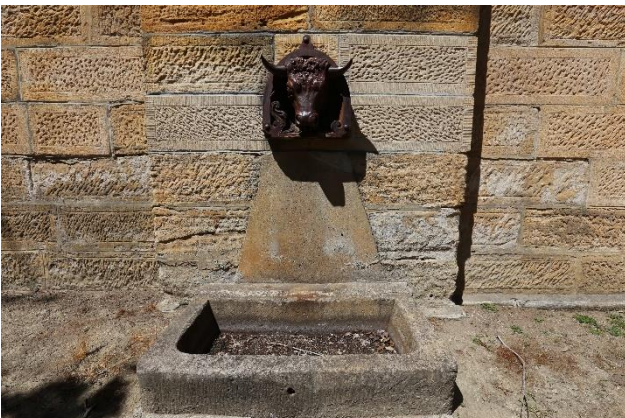
Figure 19 – Detailed view of the Bull's Head Drinking Fountain located at the northern wall of the gaol.
