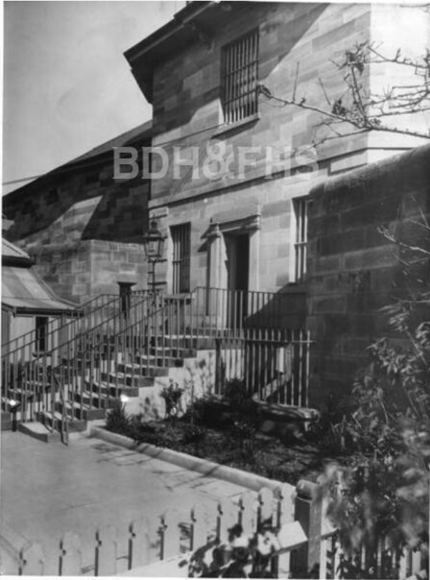
Figure A- 19 - Part of Berrima Gaol building including wing entrance steps, c.1897.
