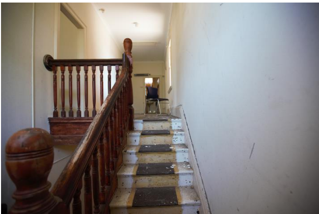
Figure 95 – Internal view of the staircase, from within the stairwell, looking south towards to first floor.
