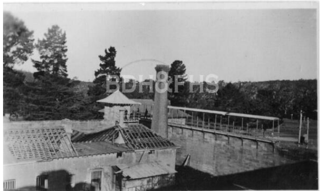
Figure A- 181 - Berrima gaol outbuilding in left foreground with dilapidated roof and a large brick chimney at the side, c.1930.
