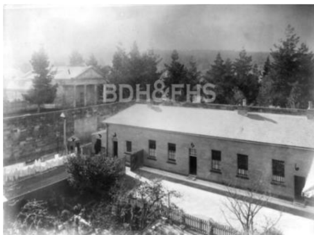
Figure 140 – Northeast corner of the gaol, showing courthouse, No. 5 Post, lamp room, library, church and school, room, and general store, c.1898.
