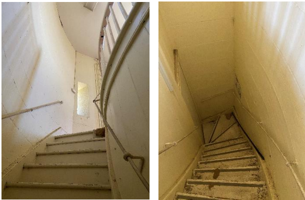
Figure 46 – Detail of timber stairs, south rooms.
