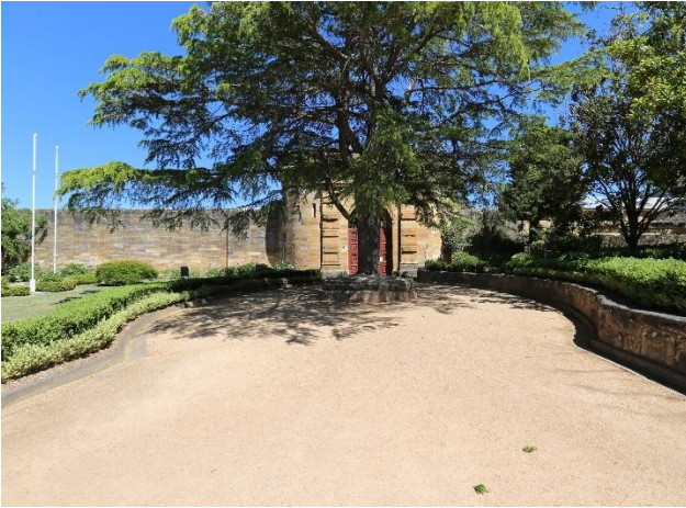
Figure 15 – General view of the exterior wall.
