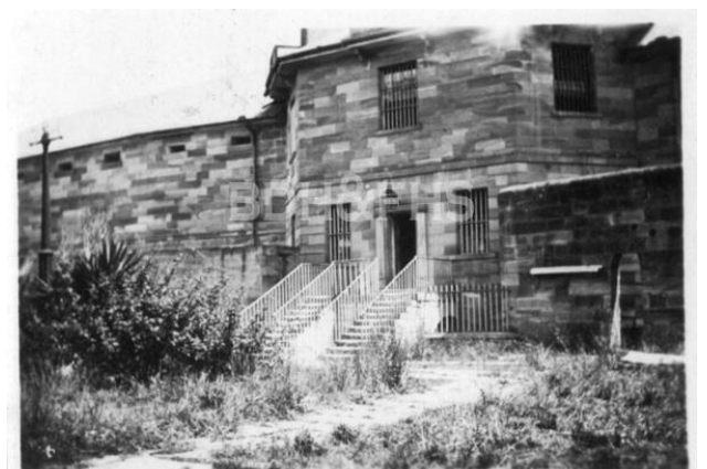
Figure A- 183 - Berrima gaol building during the period it was not occupied, c.1920s. Shows entrance steps to wing, gas lamp and garden.
