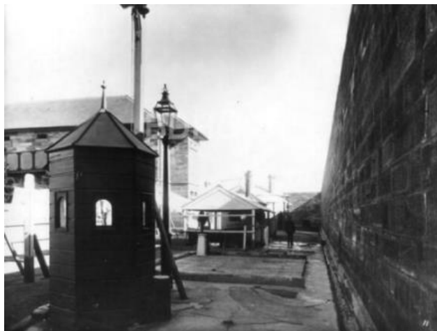
Figure 138 – No. 5 Sentry Box, Wash shed, and hospital in rear, c.1898.
