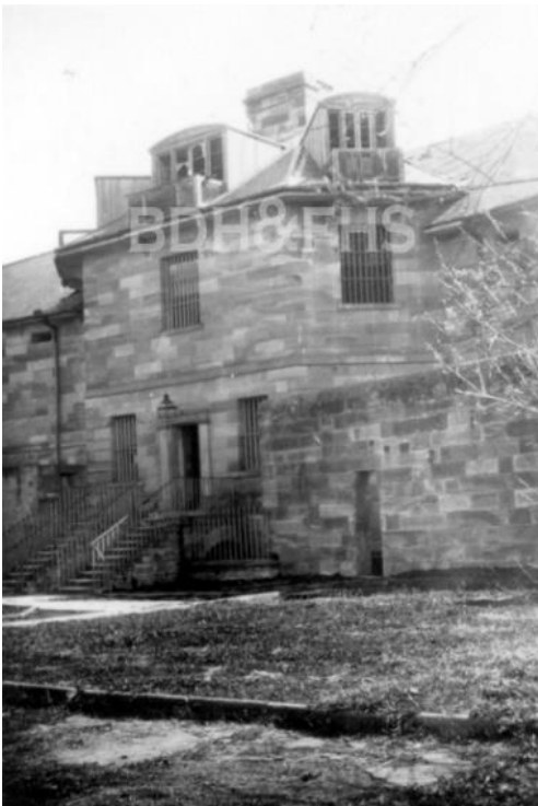
Figure A- 220 - Interior view of Gaol courtyard prior to renovation for the Berrima Training Centre, c.1930s.
