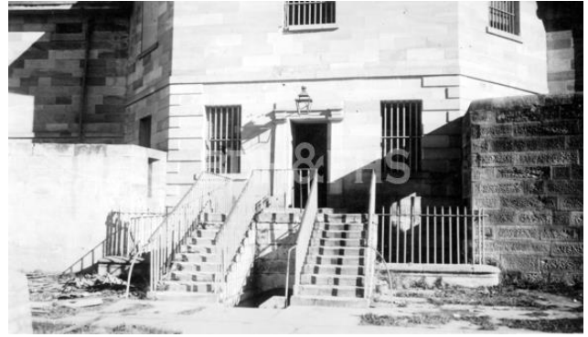
Figure A- 248 - Berrima Gaol, 1944. Photo shows the doorway into one of the buildings inside the gaol. Prior to work to establish Berrima Training Centre.
