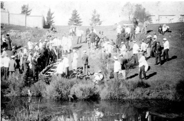
Figure A- 91 - German internees launching "Nelly" on the Wingecarribee River, with the gaol in the background, c.1916.
