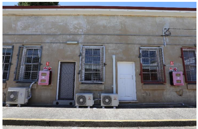
Figure 78 – Science block looking east.
