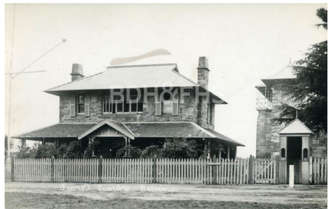
Figure A- 163 – Governor's Residence / Guards Quarters, Berrima Gaol, c.1920s.
