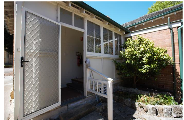
Figure 102 – View of the enclosed verandah opening at the rear of the building, looking north-east.
