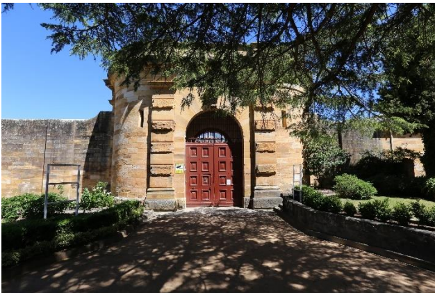
Figure 30 – View of the entrance gate from within the front courtyard, looking west.
