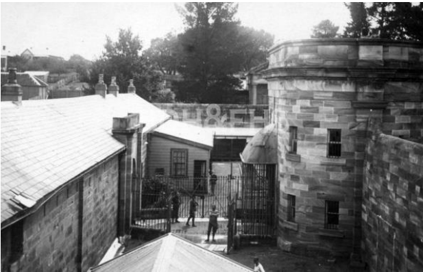
Figure A- 103 - View of small courtyard in Berrima Internment Camp between the entrance tower and the services building, c.1916.
