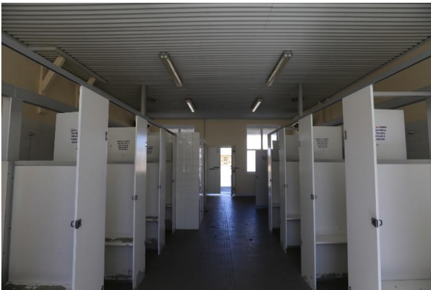
Figure 66 – Interior view of the bathroom, looking east.
