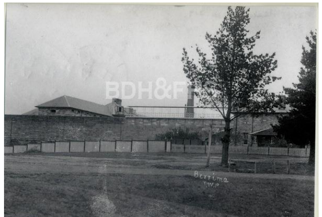
Figure A- 34 – View of southern side showing the old wing, catwalk and Governor's Residence, Berrima Gaol c.1918.
