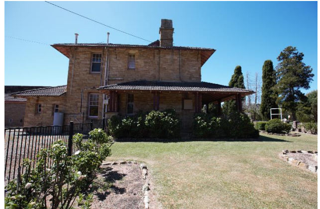
Figure 88 – View of the southern façade of the former Governor's Residence within the garden, looking north.
