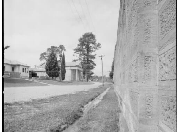
Figure A- 302 - Gaol wall and courthouse at a distance, Berrima, New South Wales, c.1970. Wes Stacey.
