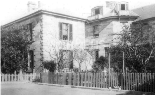
Figure A- 3 - Berrima Gaol old governor's quarters with cell block and central tower behind, c.1897.
