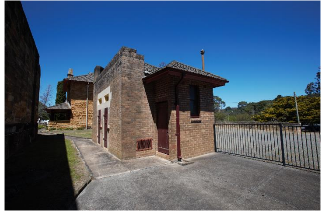
Figure 80 – View of the police cell blocks to the west of the former Governor’s Residence.
