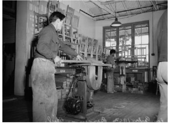
Figure 206 – Photograph, July 1953, by R. Donaldson showing the carpentry workshop at Berrima Training Centre.
