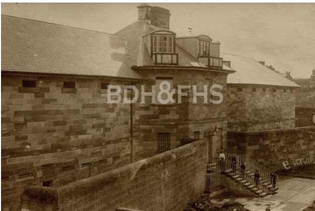
Figure A- 164 - Front of the gaol cells showing the central tower, c.1920s.
