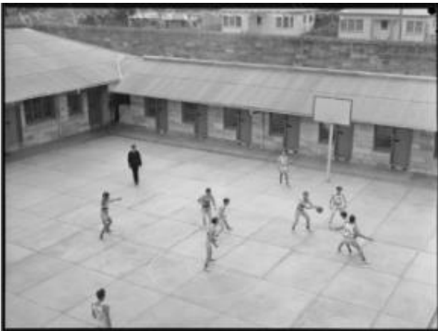
Figure 203 – Open courtyard of the western cellblock, 1953.
