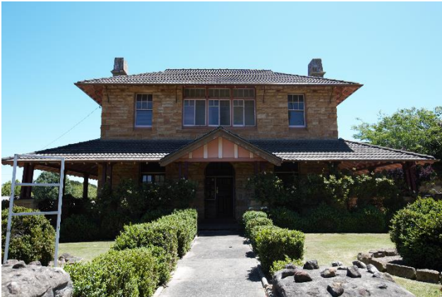
Figure 87 – View of the front façade of the former Governor's Residence and gardens, looking south.
