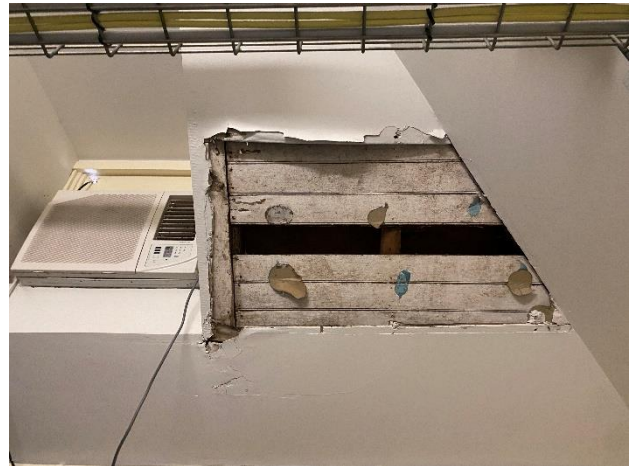
Figure 49 – Detail of remnant timber board ceiling, second floor.
