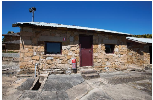
Figure 82 – The garden sheds to the south-west of the Governor’s Residence.
