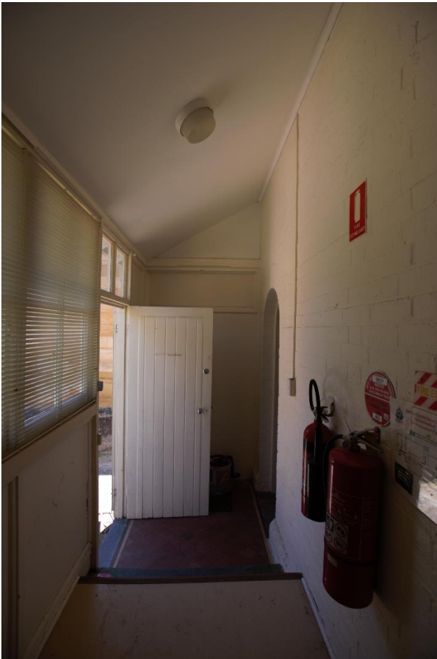
Figure 105 – View of the enclosed balcony, looking west.
