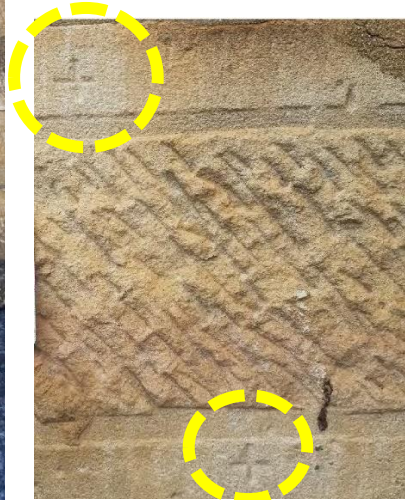
Figure 29 – Detail of date marking and crosses in stonework.
