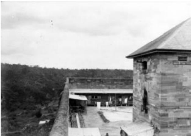
Figure 180 – Looking to the west along the south wall, 1916-9.
