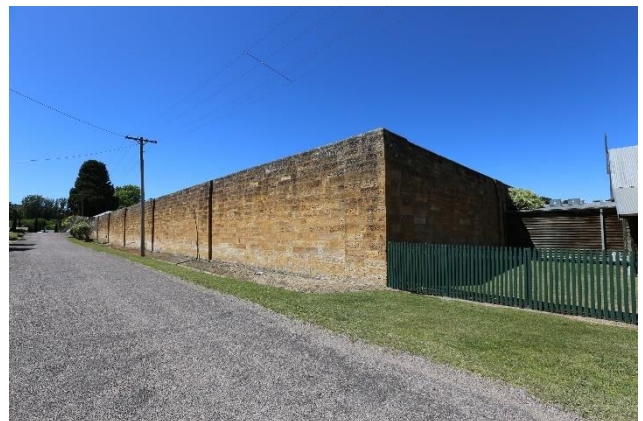
Figure 12 – View 6, a closer view of the rear of the former Gaol walls.
