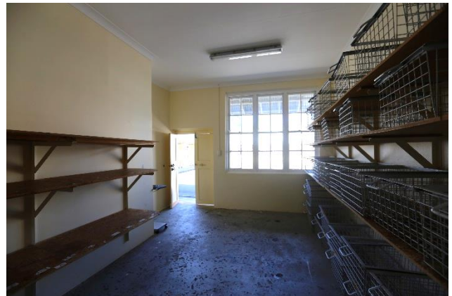
Figure 67 - Interior view of the storage room, looking west.
