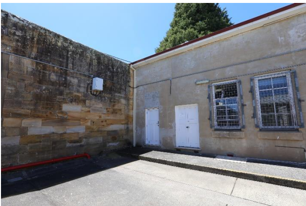
Figure 77 – Science block looking north east at junction with gaol wall.
