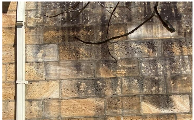
Figure 26 – Detail of 1866 section of north wall. Note the 'picked-and-boasted' finish of this section which differs from the original 1839 finishes.
