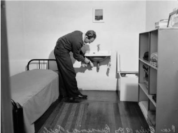
Figure 205 – Photograph, July 1953, by R. Donaldson showing a cell at Berrima Training Centre.
