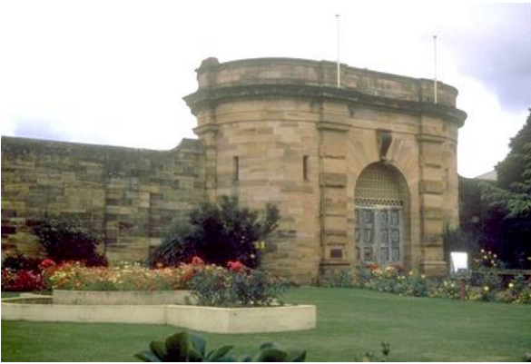
Figure A- 303 - Gatehouse and Walls of Gaol (former), November 1965.
