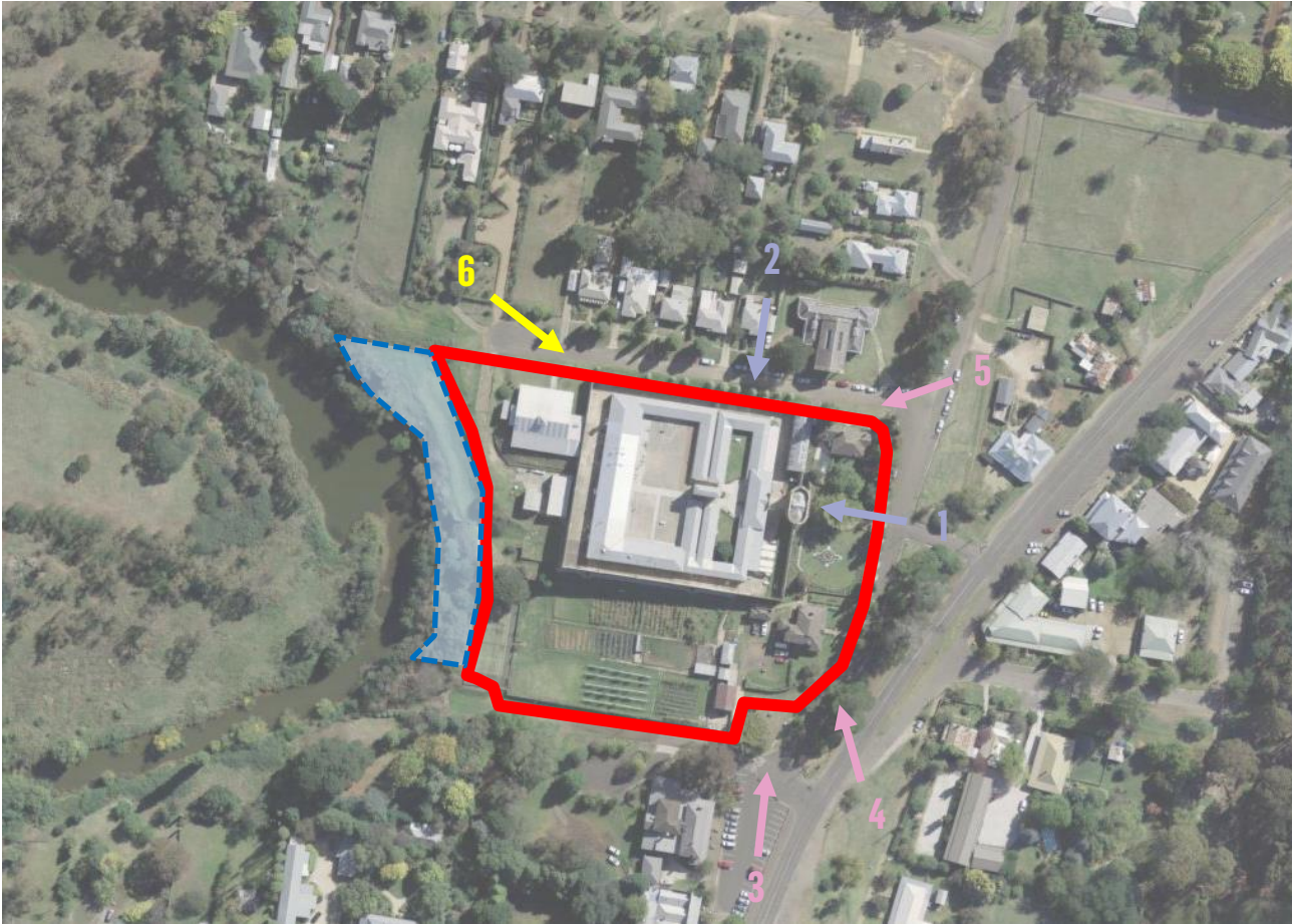
Figure 4 – Detailed views in close vicinity of the subject site (outlined in red).
