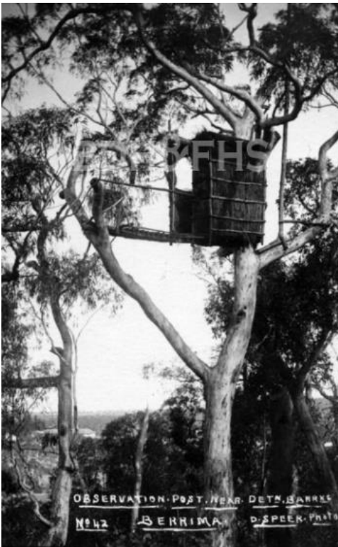
Figure A- 145 - Observation Post (Crow's Nest) built in a tree on top of 'Nobbys' by German Internees near the Detention Barracks at Berrima Gaol, c.1916.
