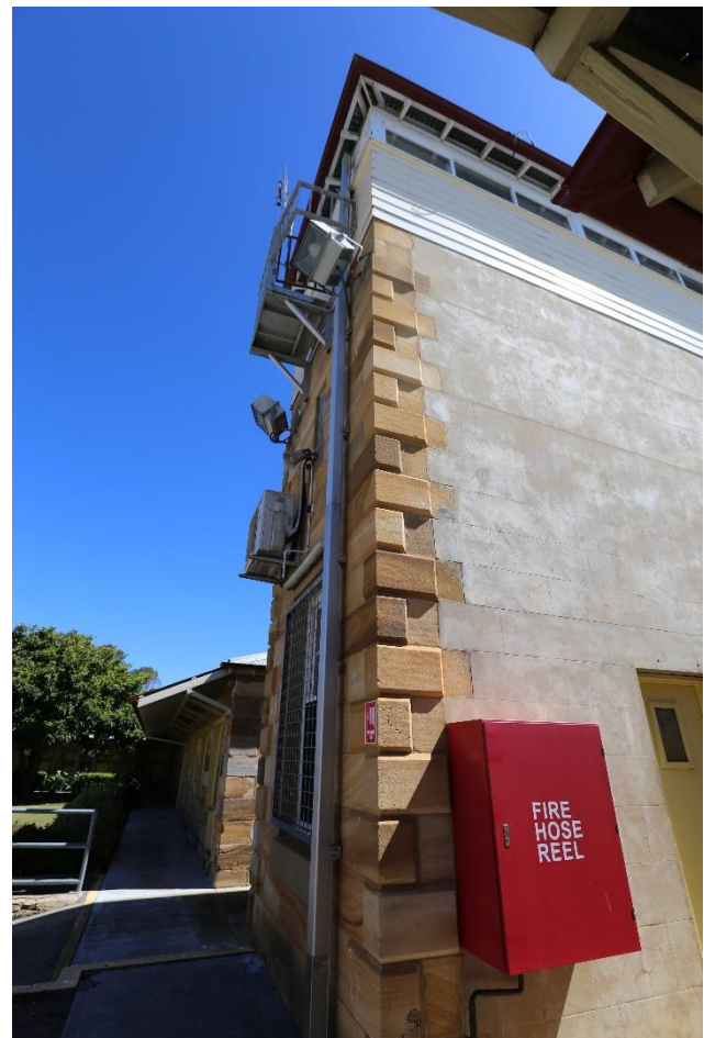
Figure 69 – Detailed view of quoining on the guard tower, looking south from within the eastern courtyard.
