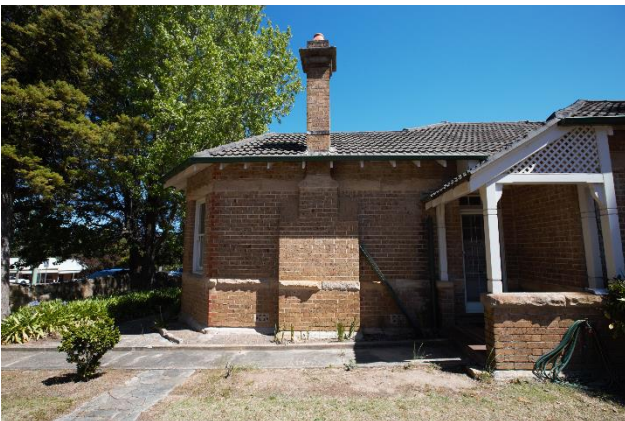
Figure 99 – View of the northern façade, looking south.
