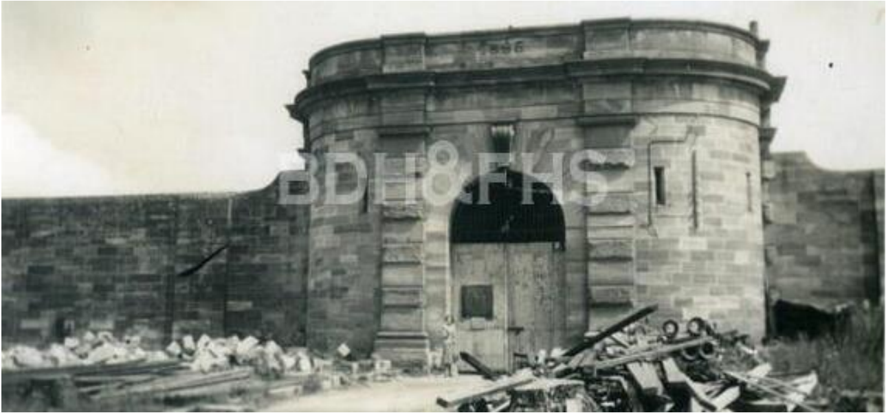
Figure 194 – Berrima Gaol entrance in 1949 during re-building works (note debris, and removal of mature pines).
