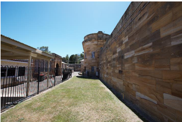
Figure 23 – Internal view of the gaol wall, looking north towards the front entrance gate.
