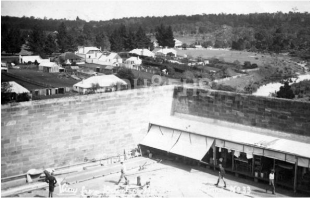
Figure A- 59 - View over the north-east corner of Berrima Gaol towards services building and Courthouse, c.1916.
