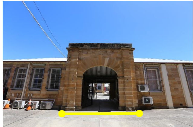
Figure 51 – Distanced view of the eastern side of the early entrance gate, showing the adjacent, flanking wings. Extent of original 1839 gate shown in yellow.
