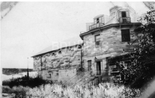
Figure A- 170 – Guard tower of Berrima Gaol during the period it was unoccupied after it ceased to be a World War I internment camp, 1923.
