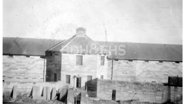
Figure A- 250 - Berrima Gaol, 1944. Photo inside the gaol showing the state of disrepair of some of the buildings prior to work to establish Berrima Training Centre.
