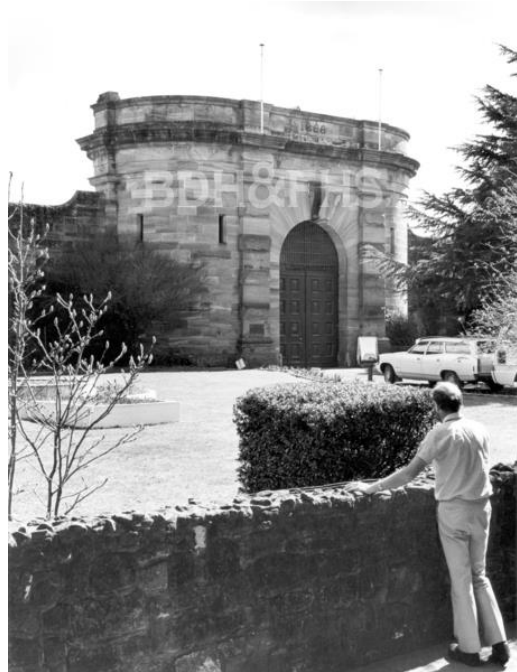
Figure 217 – Berrima Gaol wall and landscaping outside the main entrance, 1975.
