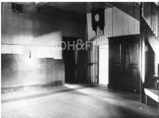
Figure 139 – Interiors of entrance wing, showing gate, staircase, clock, and cupboard, c.1898.
