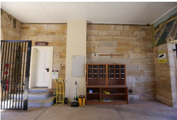
Figure 56 – View of south wing showing later door, steps, services, etc. Note the reconstructed wall.
