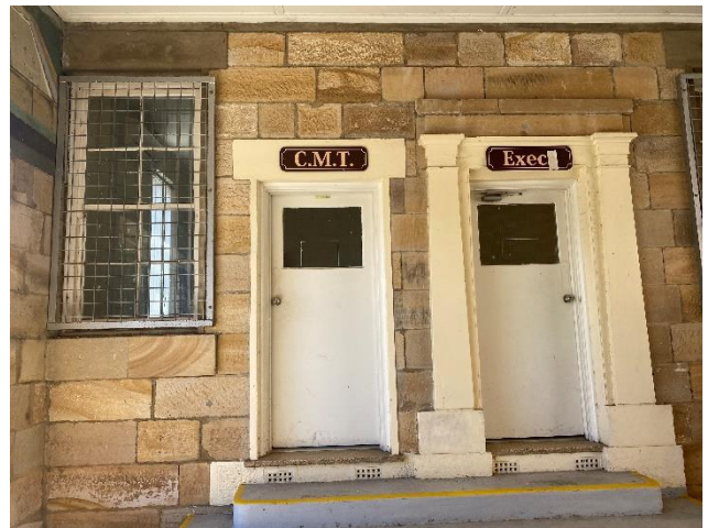
Figure 55 – View of northern wing showing 1940s doors and window. Note the reconstructed walls.
