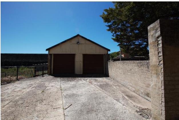
Figure 83 – The garden shed to the southern section of the subject site.
