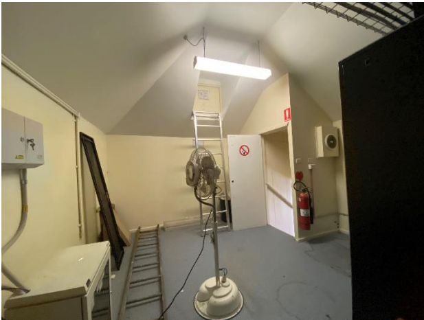
Figure 48 – Interior view from within south, second floor room
