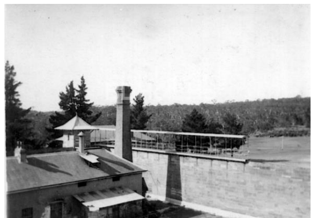
Figure A- 94 - Side wall featuring catwalk and guard's watch tower behind the service centre, c.1918.
