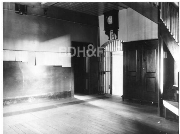
Figure A- 6 - Berrima gaol, immediately inside entrance to wing showing a gate, staircase, clock and cupboard, c.1897.
