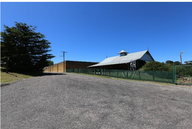
Figure 11 - View 6 from the western end of Wilshire Street, looking southeast towards the rear of the subject site, with the Industries building in the foreground.
