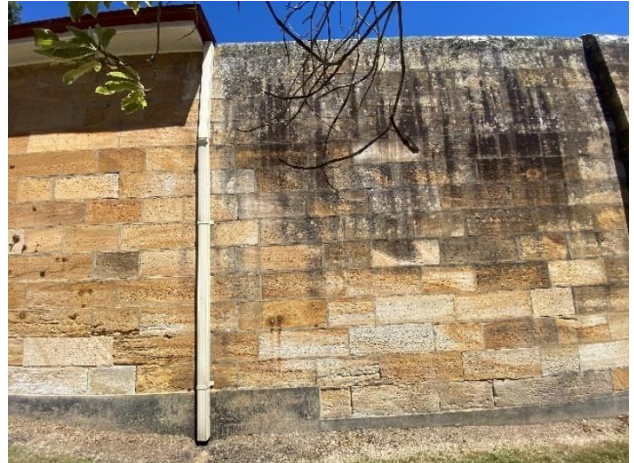
Figure 16 – Northern wall showing extension (LHS).
