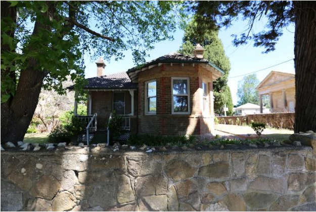
Figure 97 – View of the building from Argyle Street, looking west.
