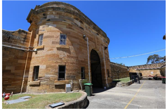
Figure 39 – View from within the 'sterile zone', looking south-west.
