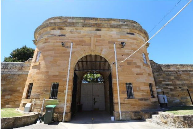
Figure 38 – View from within the 'sterile zone', looking east towards the main entrance gate.
