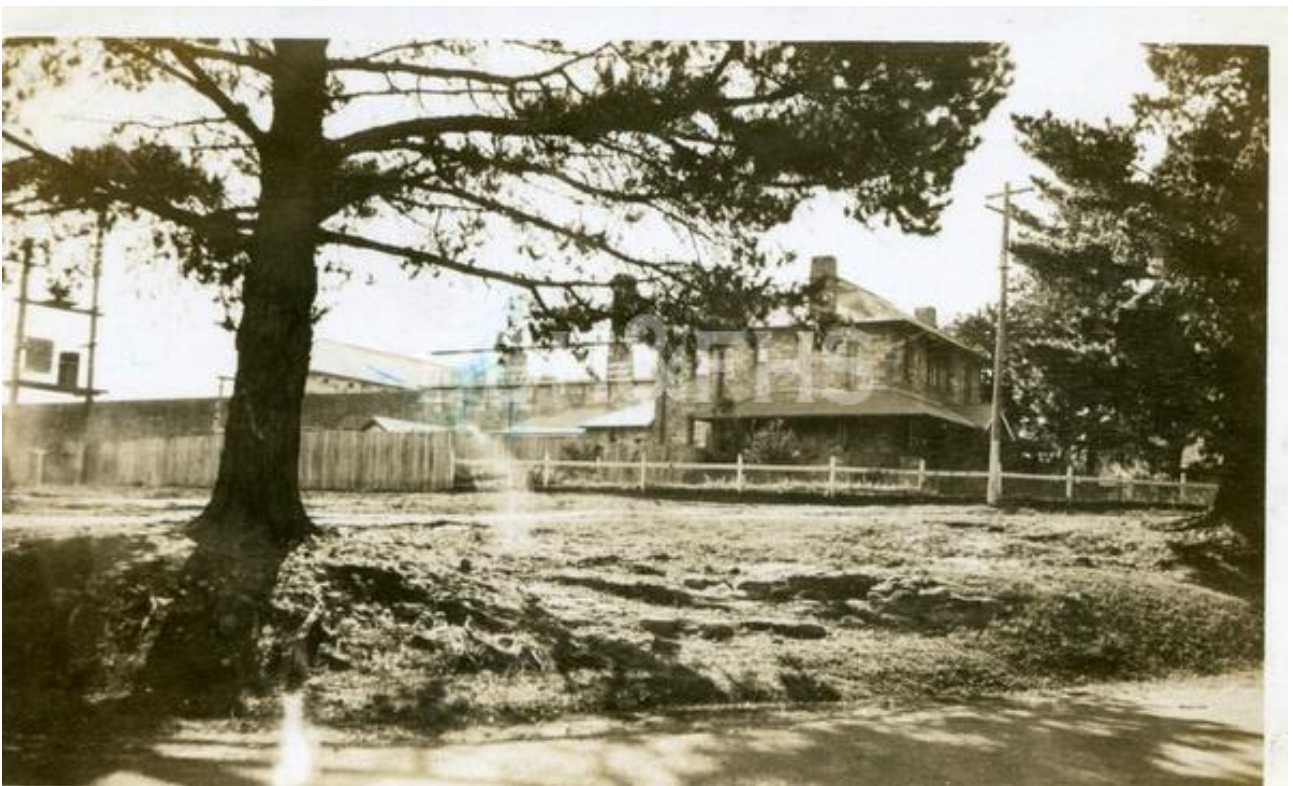
Figure 153 – Berrima Gaol walls and Governor's Residence and garden, 1936. Note the rear configuration of the building, fencing to the lot and higher timber fencing to the rear.
