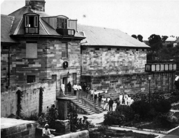
Figure 166 – Photograph of Berrima Gaol viewed from inside the gaol walls, showing the central building as seen from the south-east, c.1916.
