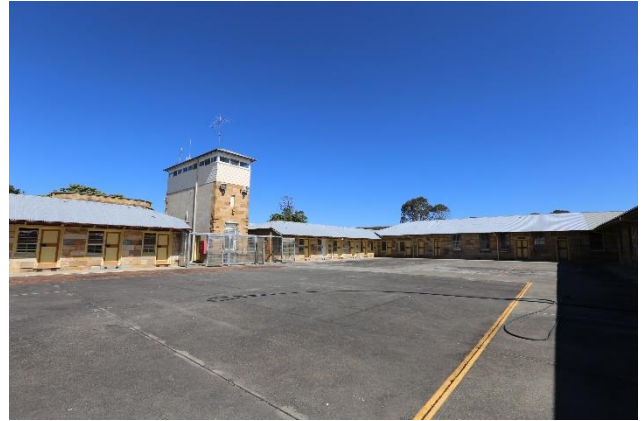
Figure 63 – View from within the western cell block courtyard, looking southeast towards the guard tower.
