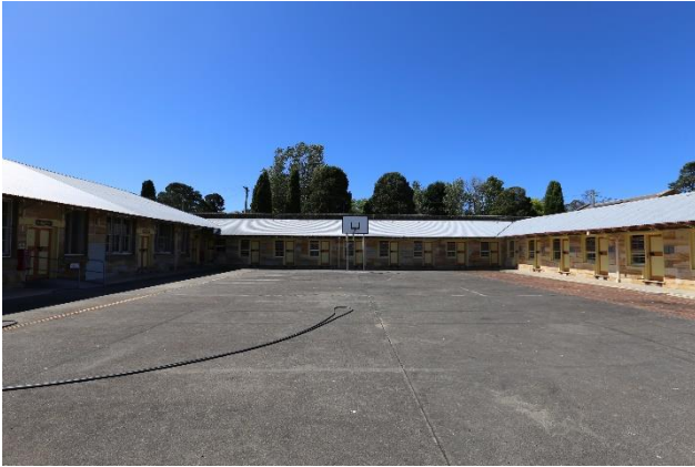
Figure 62 - View of the basketball court and courtyard from within the western cell block, looking north.
