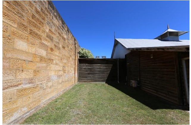
Figure 22 – View of the western wall and Industries Building, looking west.
