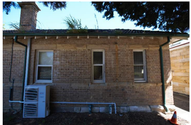
Figure 100 – View of the western portion of the northern façade, looking south.
