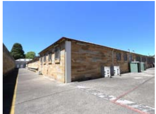
Picture 26 View east showing eastern cell block.
