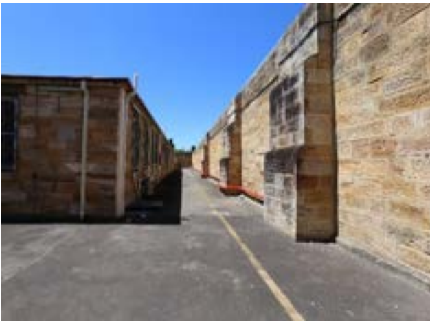
Picture 25 View west alongside eastern cell block, showing buttresses introduced on northern Gaol wall.
