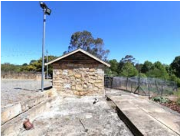
Picture 41 Sandstone and brick garden sheds located outside the Gaol wall on the south.
