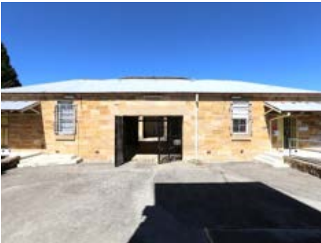
Picture 37 View east into east cell block looking back towards entrance.
