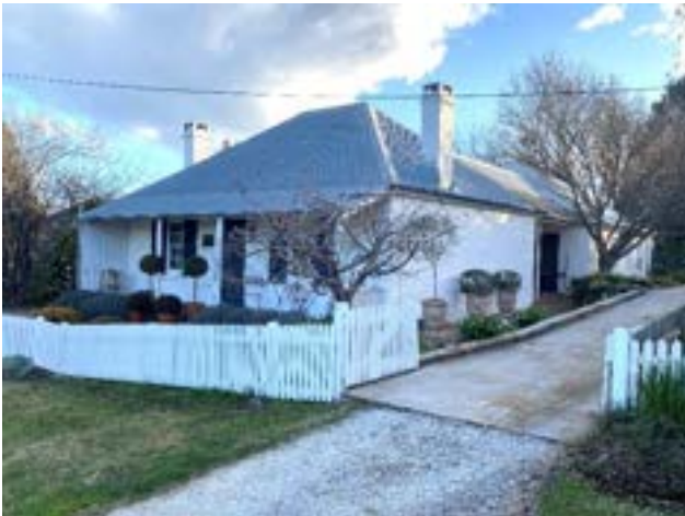
Picture 61 Sovereign Cottage, 8 Argyle Street (Item I214)
