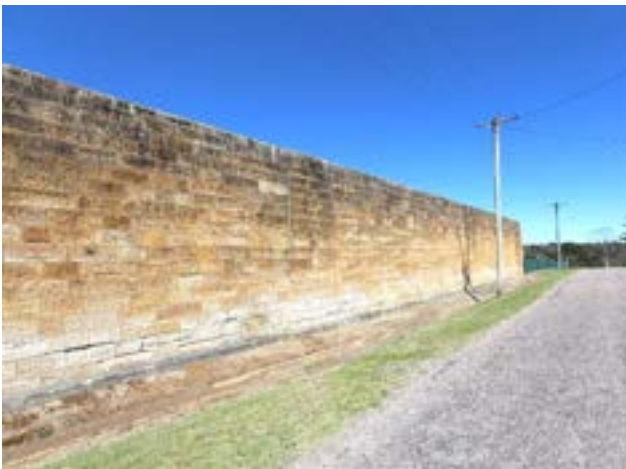
Picture 19 Northern Gaol wall, viewed from Wilshire Street. Source: Urbis
