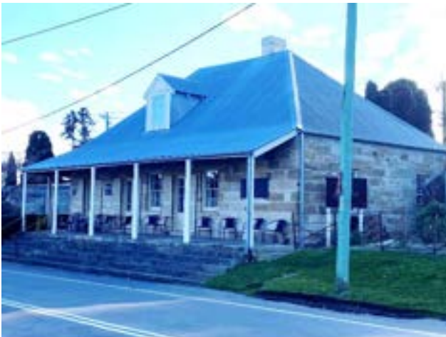
Picture 55 Old Breens Inn (former Colonial Inn), 24 Old Hume Highway (Item I140).
