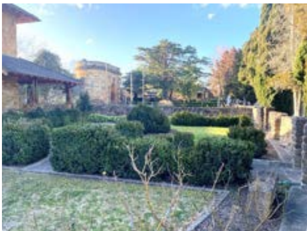
Picture 15 Berrima Gaol, looking north west across former Governor's Residence garden.
