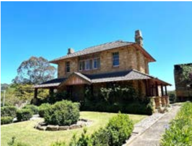
Picture 47 Former Governor's residence and front garden, facing Argyle Street.
