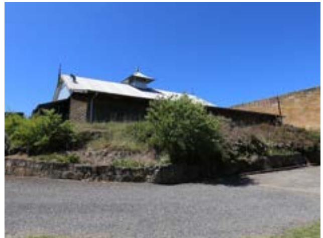
Picture 38 Industries Building viewed from adjacent to the western boundary of the subject site.
