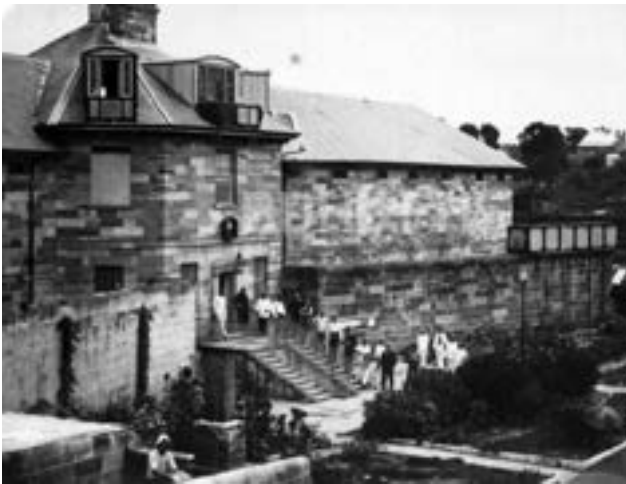
Figure 8 –Berrima Gaol viewed from inside the gaol walls, showing the central building as seen from the south-east, c.1916.
