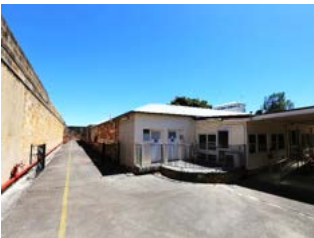
Picture 27 View west showing eastern cell block adjacent to southern Gaol wall.
