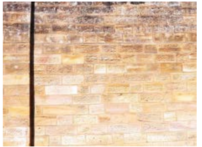
Picture 20 Detail view of stone work of southern Gaol wall, showing different finishes. Source: Urbis
