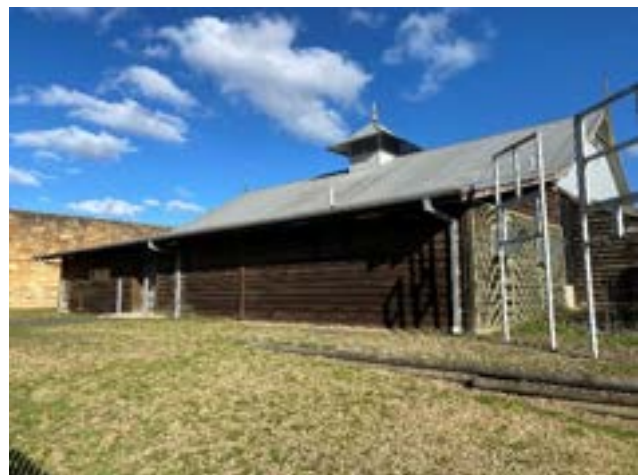
Picture 40 Industries Building, looking south east from Wilshire Street.
