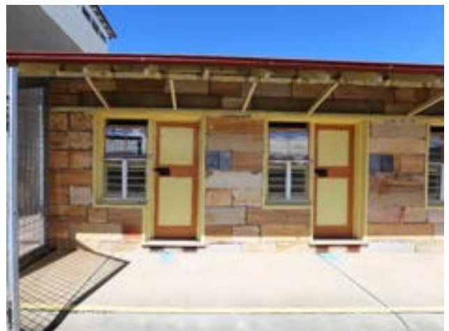
Picture 28 Detail elevation of cell block showing arrangement of windows and doors to cells.
