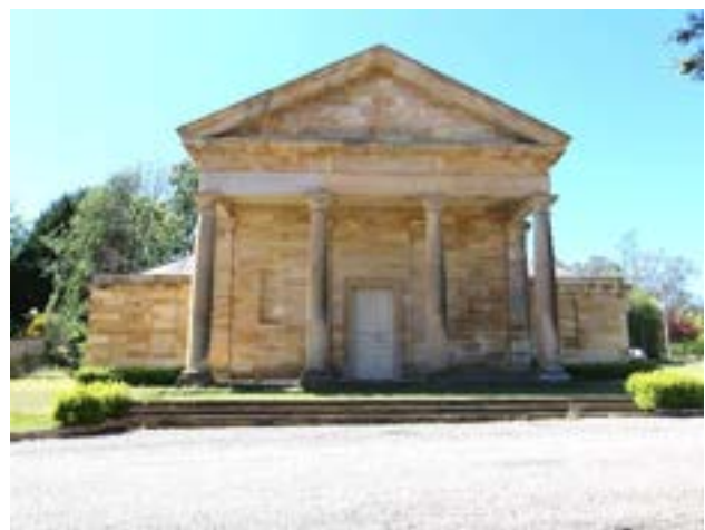
Picture 4 Southern elevation of Berrima Court
