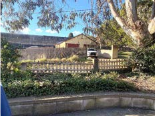
Picture 11 View to the southern wall of the Gaol from the outdoor seating area of the Surveyor General public house.
