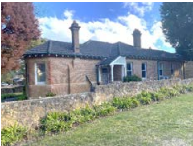
Picture 49 Former Deputy Governor's residence; elevation to Wilshire Street.
