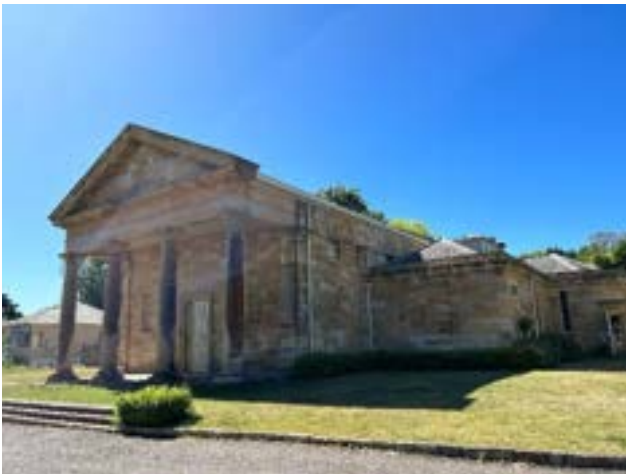
Picture 51 Berrima Court House, corner Wilshire and Argyle Streets (Item I108).
