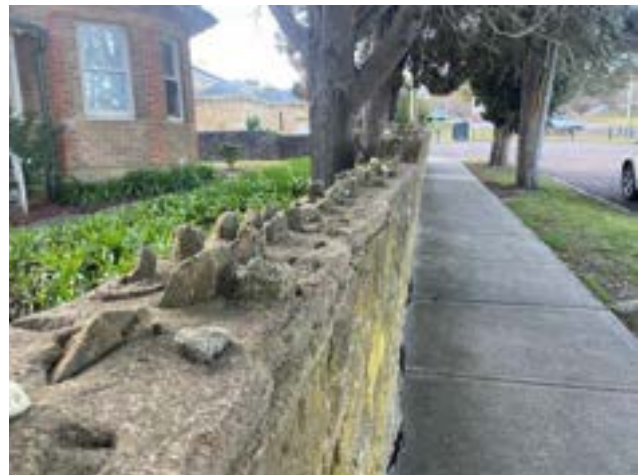
Picture 50 Detail view of wall around former Deputy Governor's residence.
