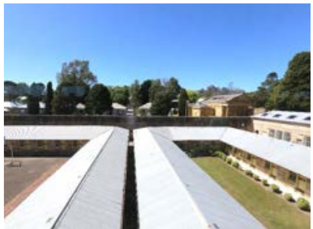
Picture 34 View north across the cell blocks from the guard tower.
