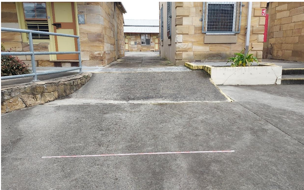
Figure 7.5 West-facing view of courtyard concrete floor (2 m scale).
