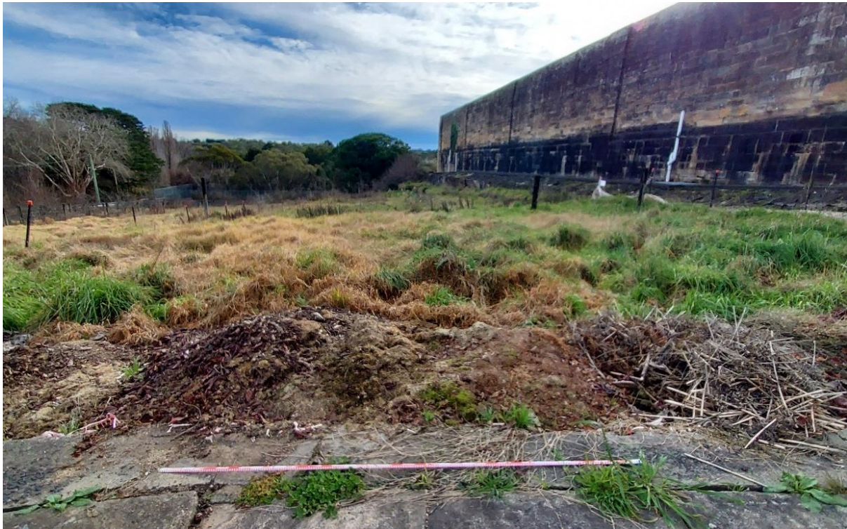
Figure 7.28 West-facing view of slope (2 m scale).
