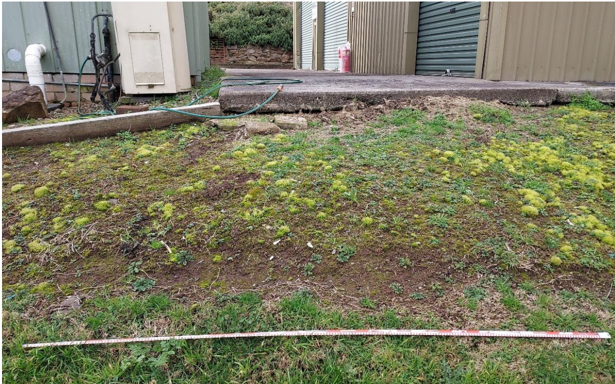
Figure 7.24 North-facing view of exposed slope near warehouses (2 m scale).
