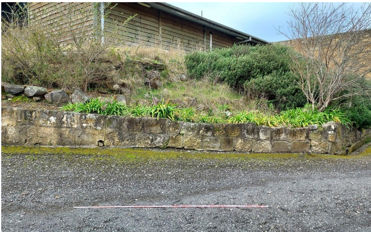
Figure 7.21 Northeast-facing view of modified ground level at western boundary (2 m scale).
