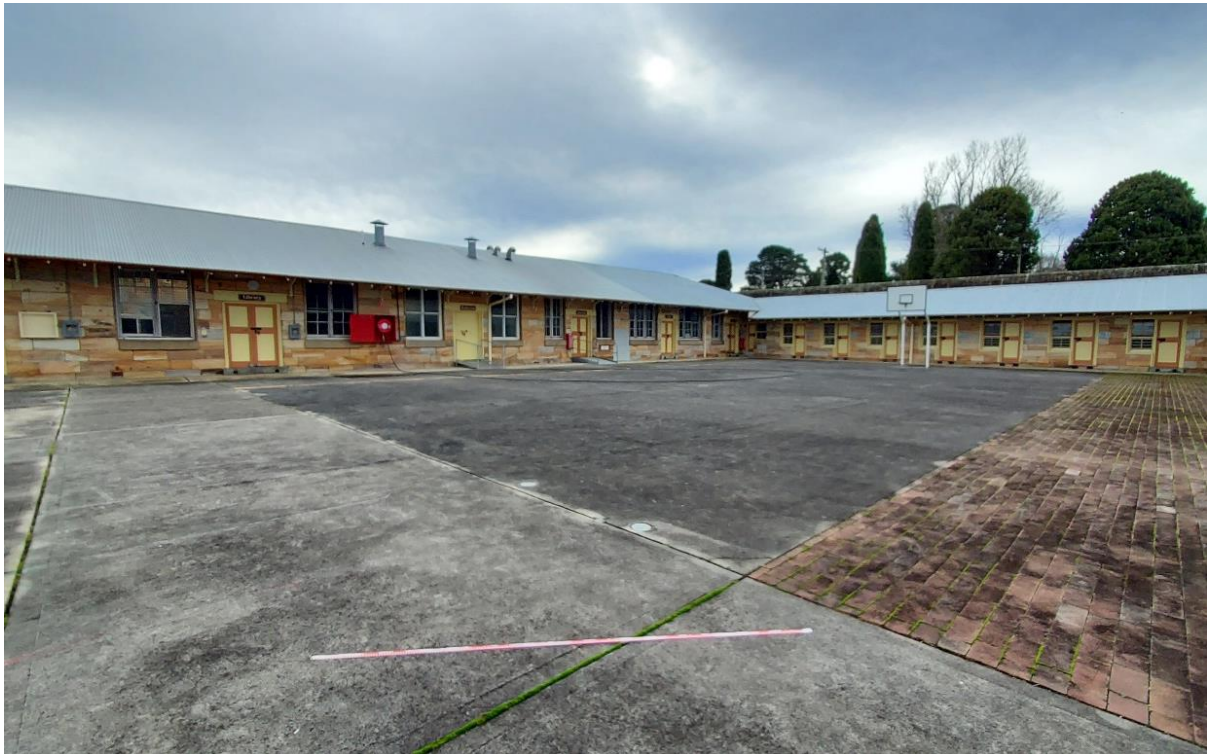
Figure 7.8 Northwest-facing view of courtyard (2 m scale).
