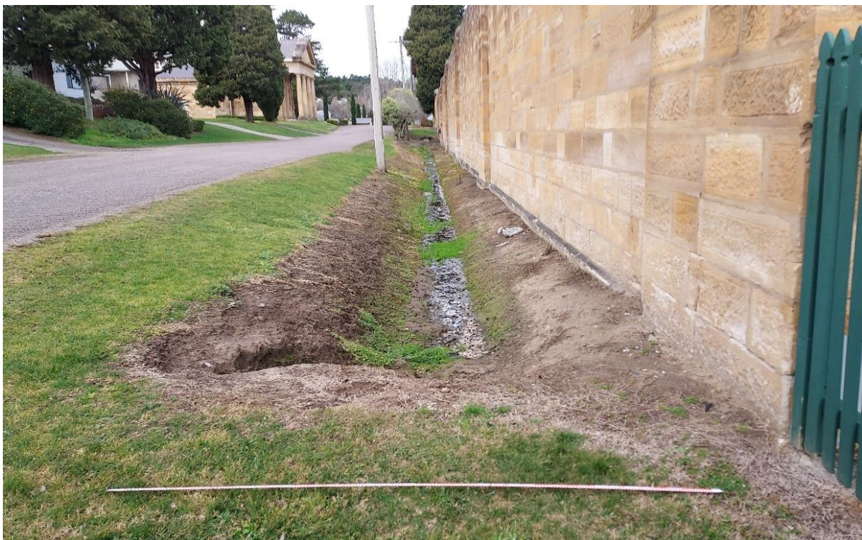
Figure 7.17 East-facing view of drainage channel and slope (2 m scale).
