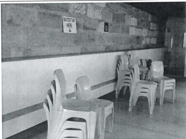
Photo No: J145125-BCC001-Photo013 Result: SMF - Positive Building/Level: 004 Visitors Facility-Ground Level Room/Location: Visitors Room-Western Side in Wall Feature/Material: Pipework Insulation-Insulation Material
