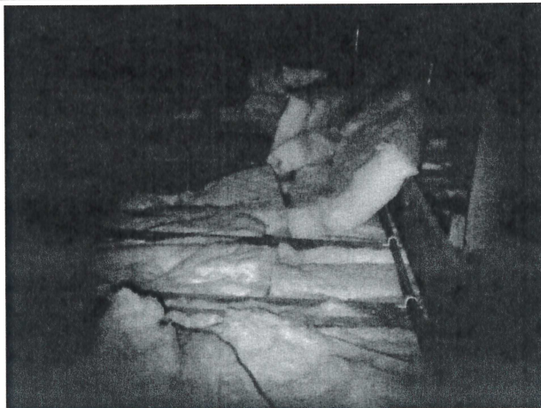
Photo No: J145125-BCC001-Photo036 Result: SMF - Positive Building/Level: 013 Kitchen/Dining/Activities-Ground Level Room/Location: Ceiling Space-Throughout Feature/Material: Pipework Insulation-Insulation Material
