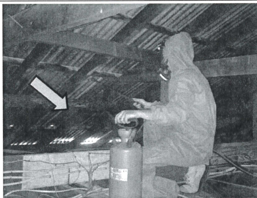
Photo 8. Block D, C & Sally Port, Ceiling space, Diluted PVA solution been applied following removal works.
