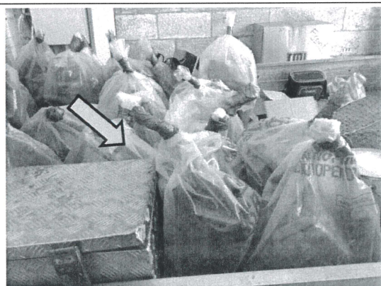
Photo 9. Asbestos waste material bagged in 200 µm thick plastic waste bags for removal from site.
