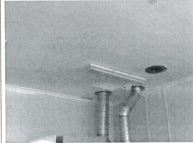
Photo No: J145125-BCC001-Photo032 Result: Asbestos - Previously Sampled Positive Building/Level: 013 Kitchen/Dining/Activities-Ground Level Room/Location: Laundry-Throughout Feature/Material: Ceiling-Fibre Cement Sheetting
