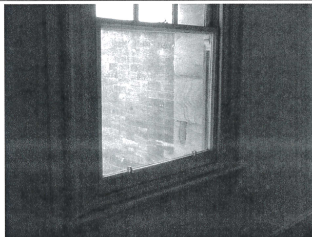
Photo No: J145125-BCC001-Photo072 Result: Lead (Paint) - Previously Sampled Positive Building/Level: 018 Oberon House-Level One Room/Location: Throughout-Windows Feature/Material: Window Frame-Lower Paint System/s
