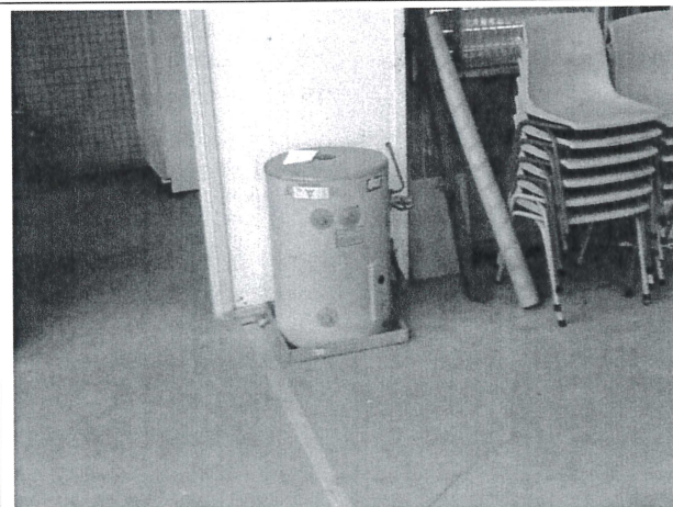
Photo No: J145125-BCC001-Photo040 Result: SMF - Presumed Positive Building/Level: 016 Industries Building-Ground Level Room/Location: Main Workshop-West Feature/Material: Hot Water Heater-Insulation Material
