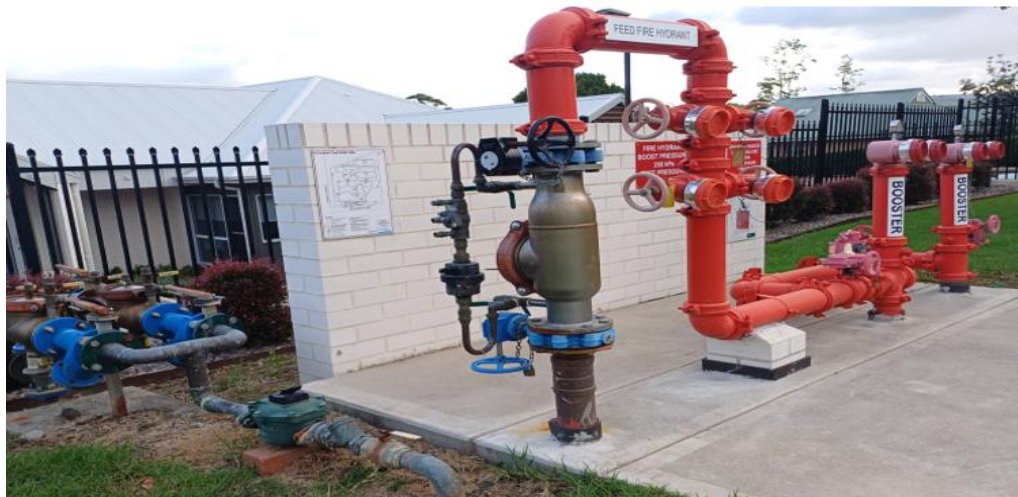
Image 17 typically exposed pumps and meters to potential 'interference' and damage - Harris
