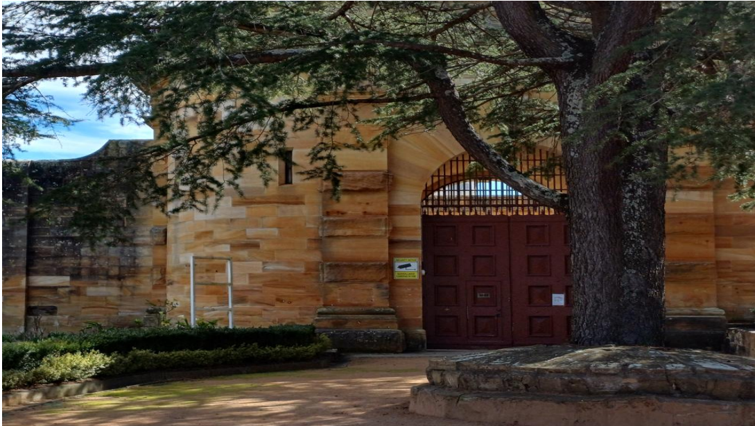
Image 2 one of two 'original' entrances to the Berrima Gaol - Harris
