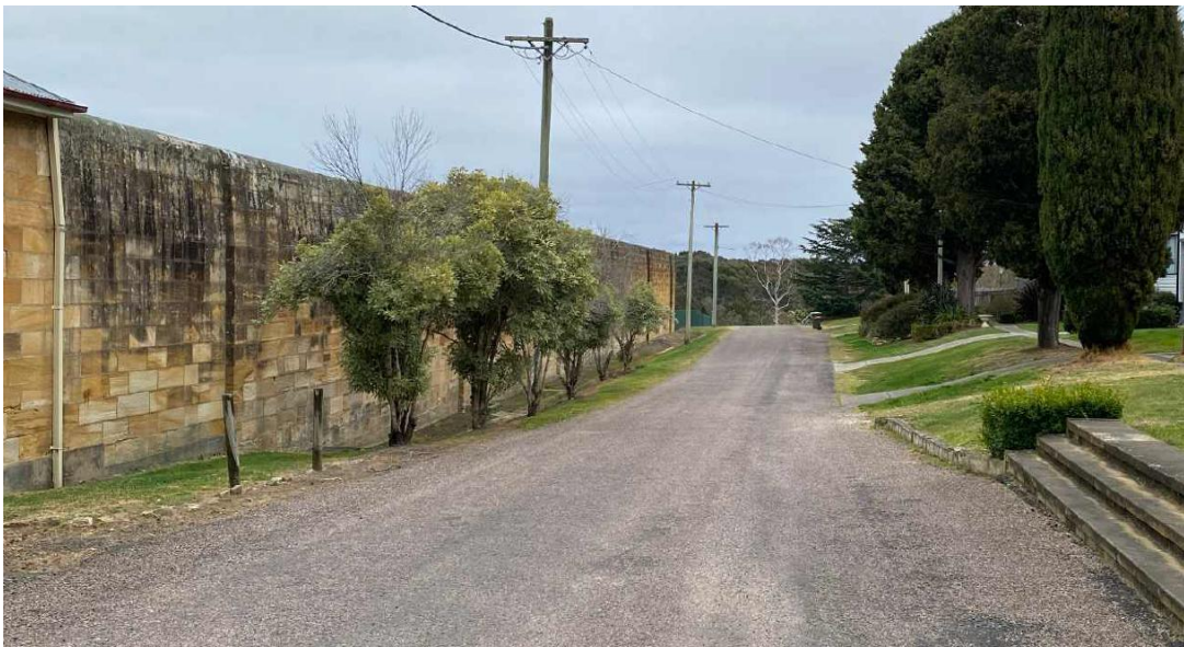
Image 6 the northern Gaol wall fronting Wilshire Street - Turner
