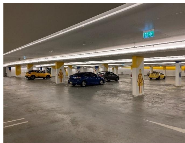
Images 24 and 25 continuation of recommended 'no dark gaps' basement overhead and wall washed lighting to promote proximate-distant object clarity for maximum surveillance - Harris
