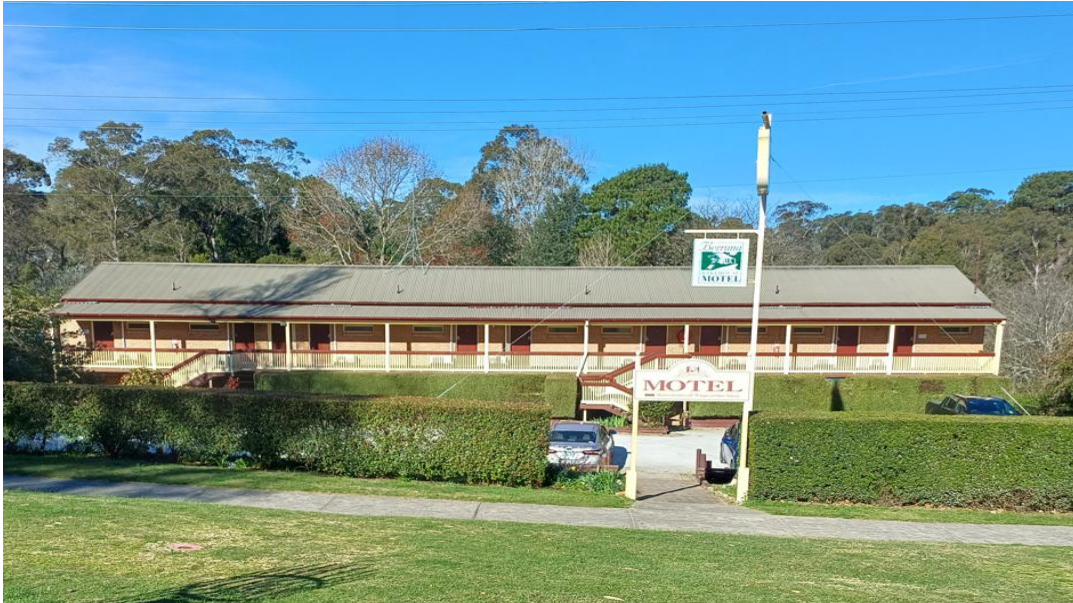
Image 7 attractive main street (Argyle Street) motel accommodation - Harris
