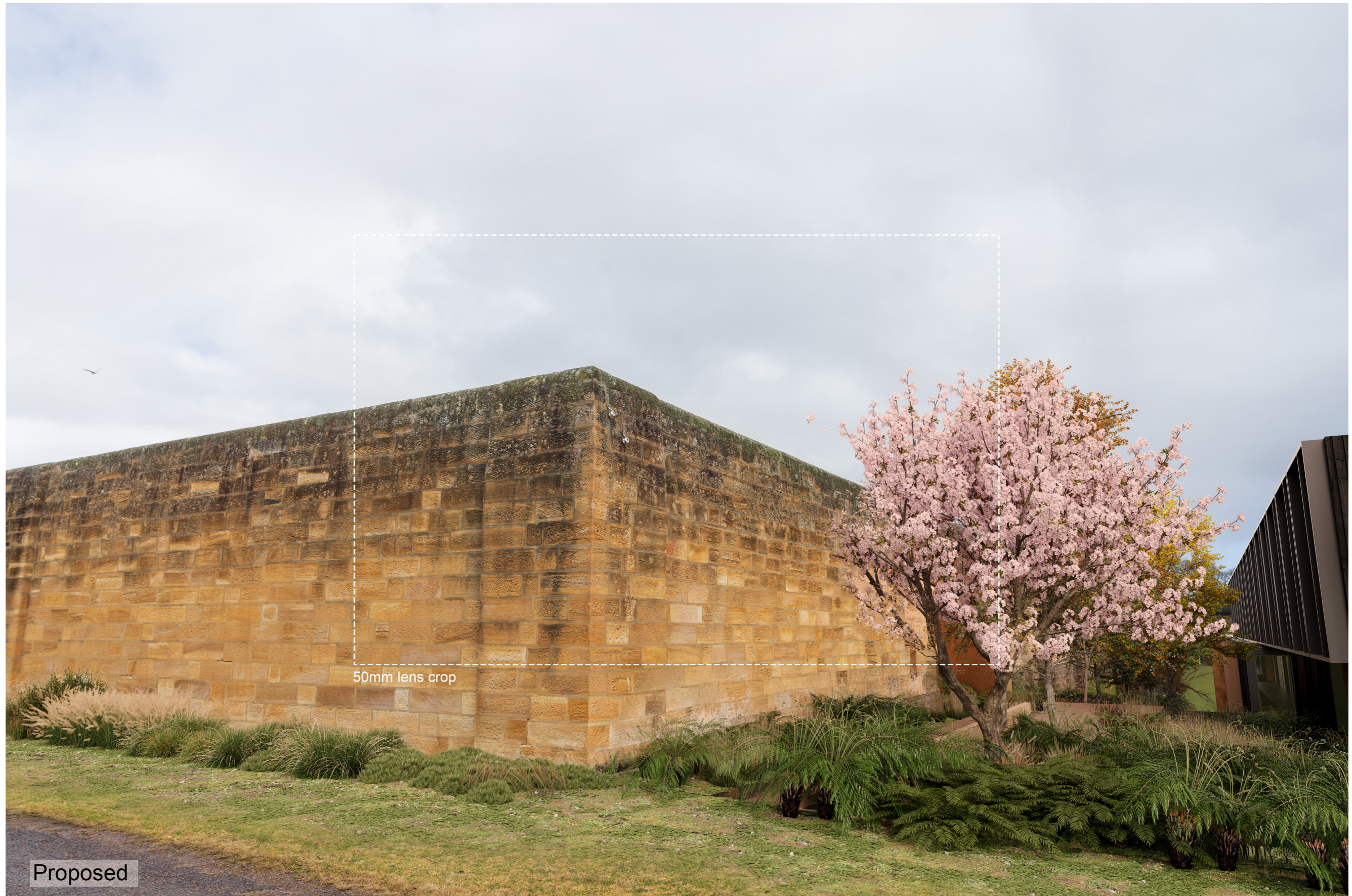
Figure 24. Viewpoint 3: Gaol Wall and western annexe (Wilshire Street) - proposed view Source: Virtual Ideas
