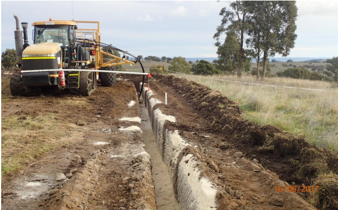
Figure 4-18: Laying underground transmission line within the road network
