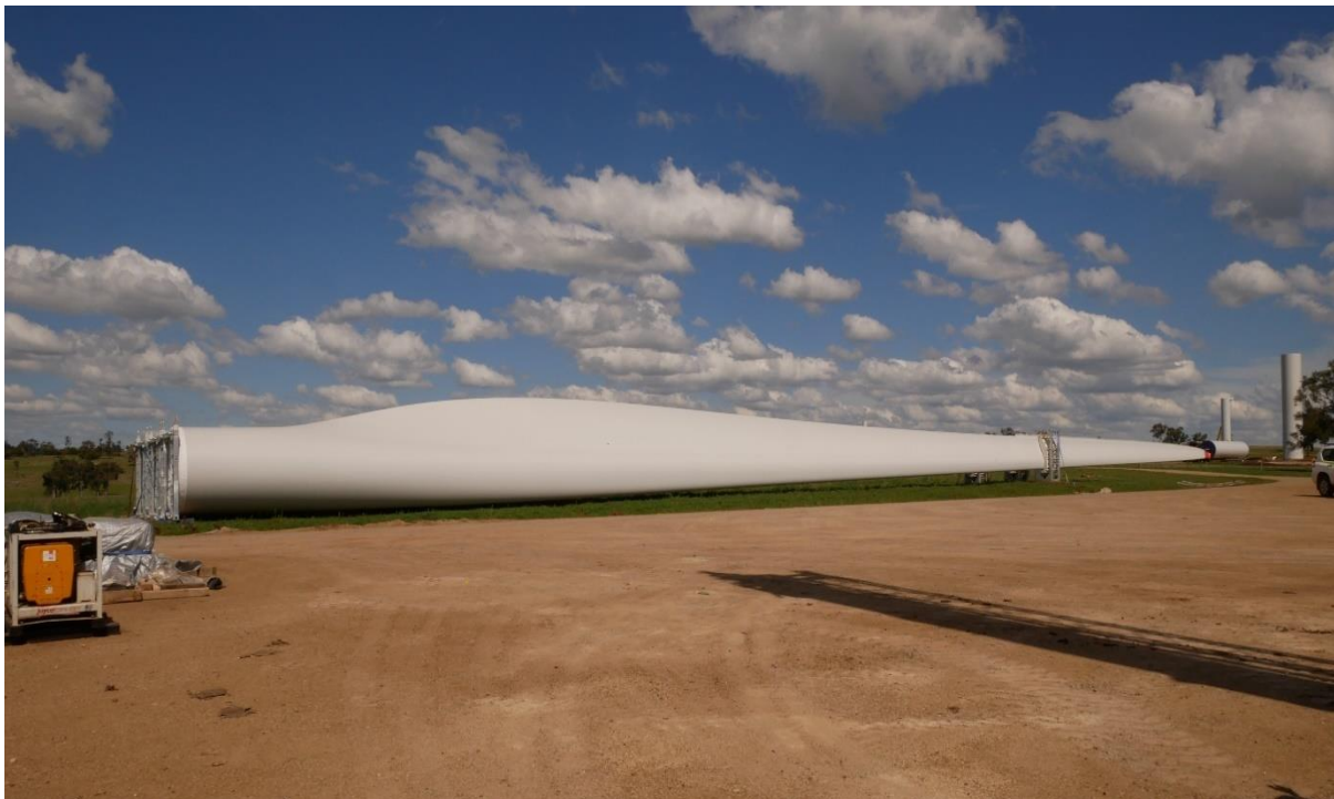
Figure 4-10: A single piece blade approximately 62 m long at Sapphire Wind Farm
