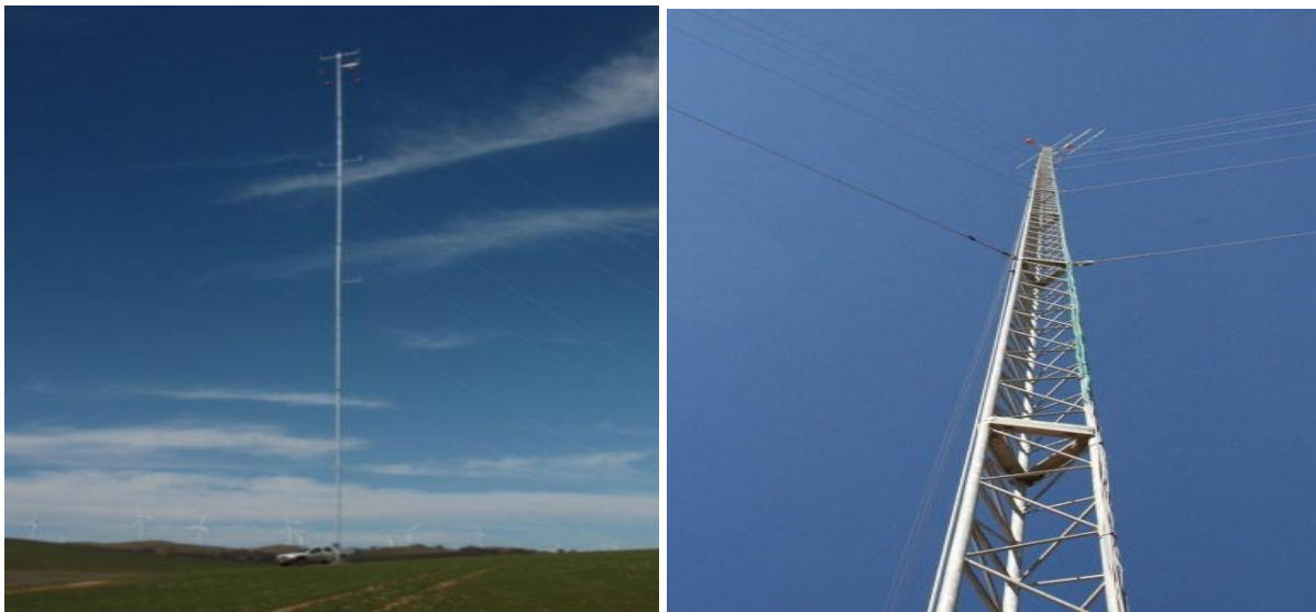
Figure 4-19: Tubular (left) and lattice (right) wind monitoring masts
