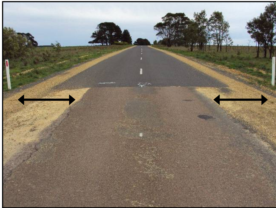
Figure 5.2: Typical unsealed increase in width of (public) road
