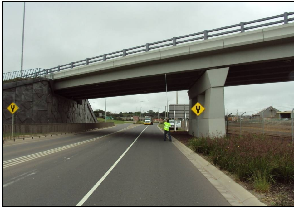
Figure 5.3: Identification of bridge underpass height risk
