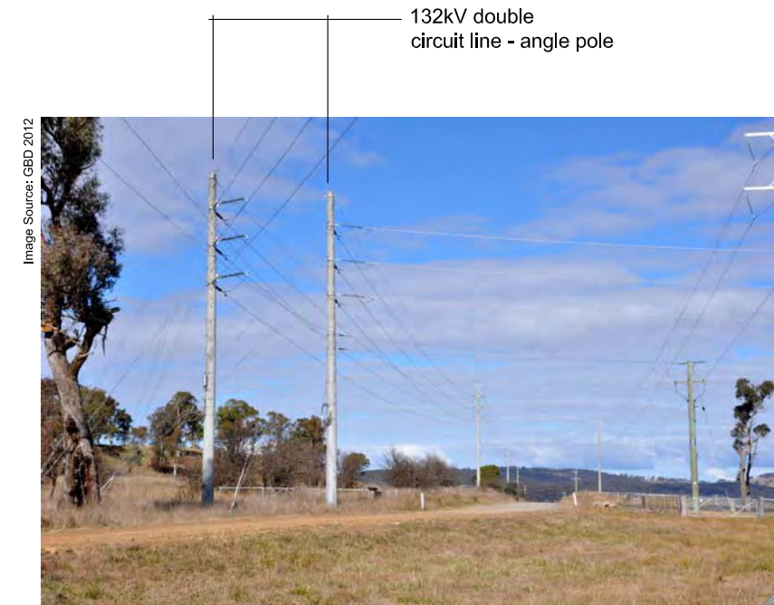
Double circuit 132kV transmission line (angle pole structure) at road crossing
