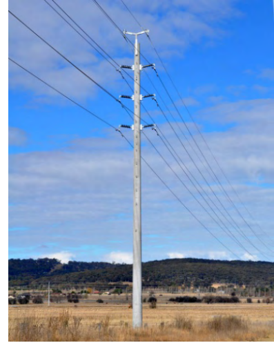
Plate 8 – Typical illustration of a 132 kV double circuit powerline
