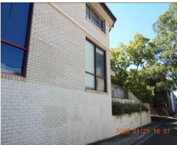
Figure 289 - General condition of external wall
