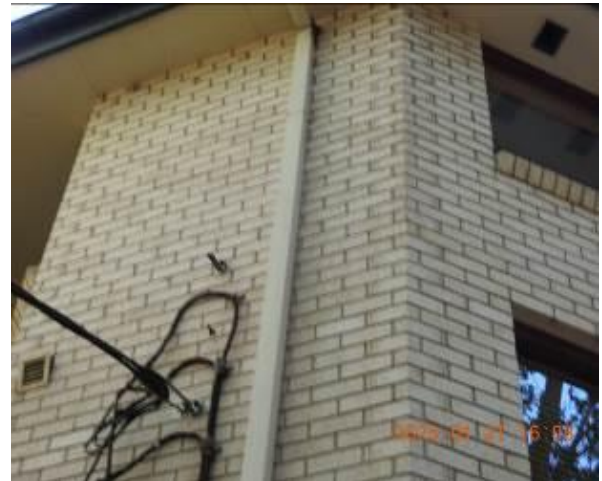
Figure 314 - General condition of external wall
