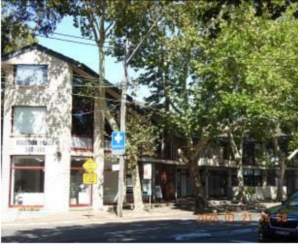
Figure 207 - General condition of external wall
