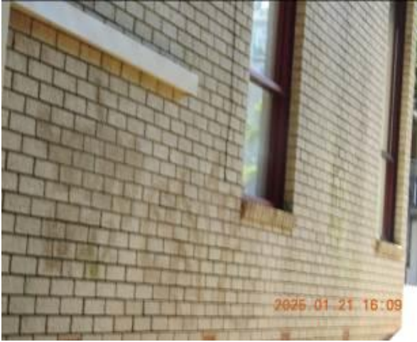
Figure 327 - General condition of external wall
