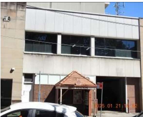
Figure 181 - General condition of external wall
