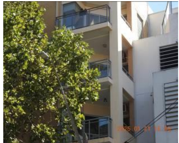
Figure 73 - General condition of external wall
