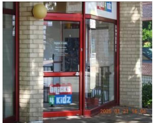
Figure 254 - General condition of external wall
