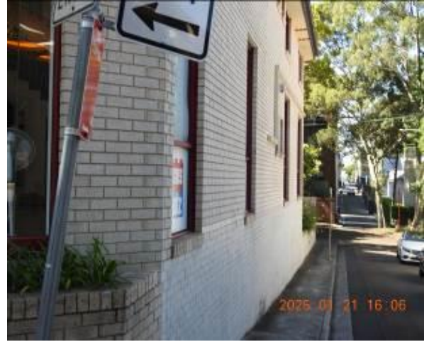
Figure 280 - General condition of external wall
