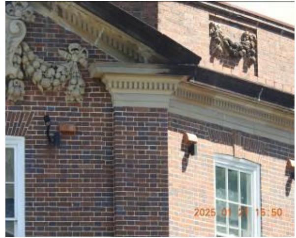
Figure 154 - General condition of external wall
