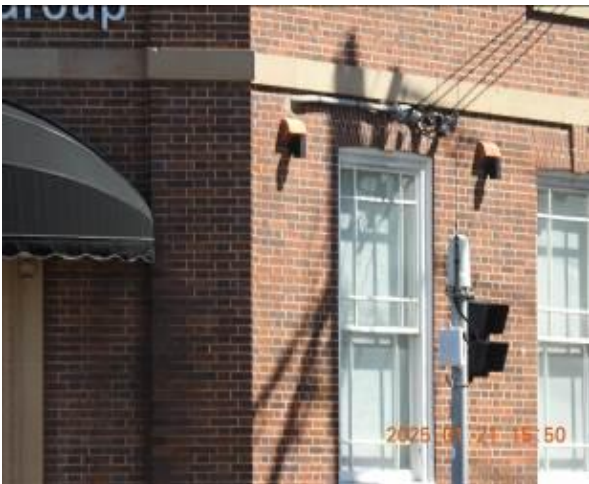
Figure 161 - General condition of external wall
