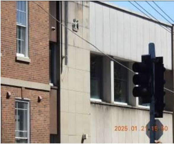
Figure 165 - General condition of external wall
