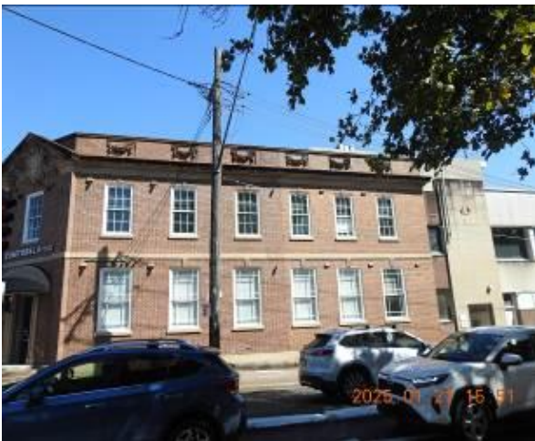
Figure 167 - General condition of external wall
