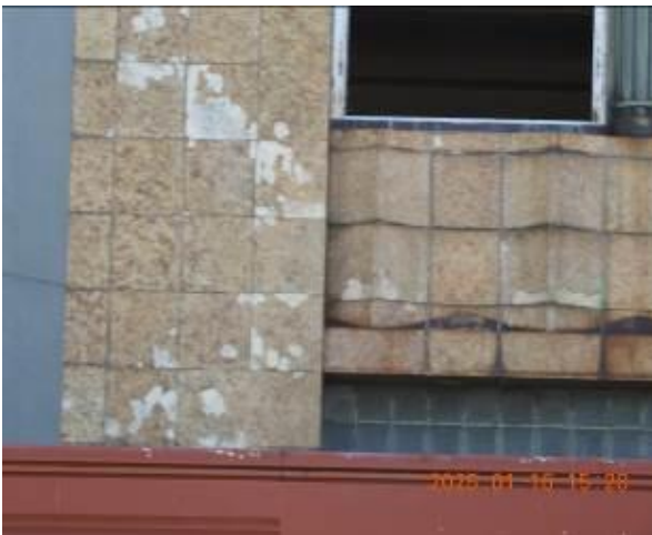
Figure 129 - General condition of external wall
