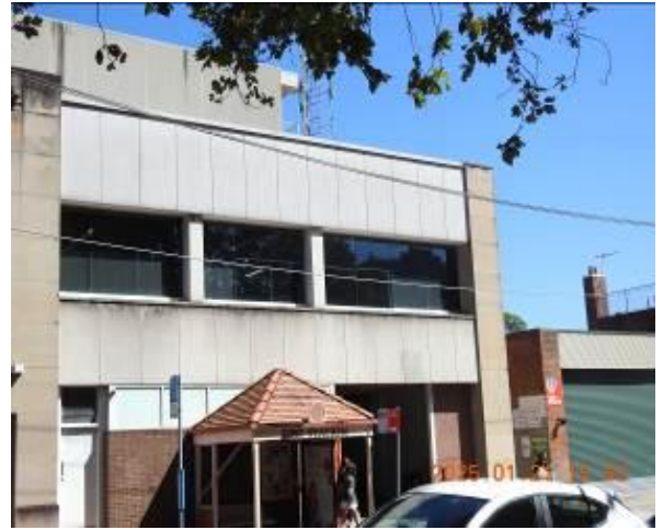
Figure 178 - General condition of external wall
