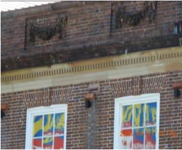
Figure 147 - General condition of external wall
