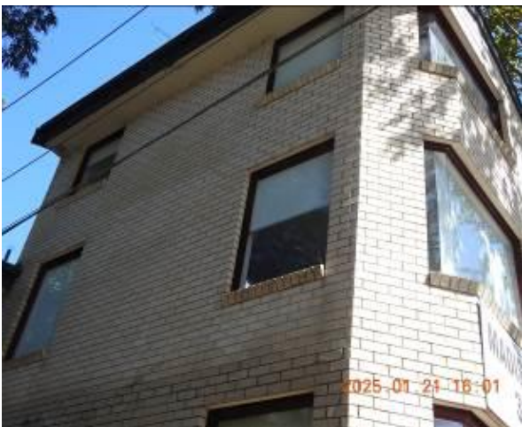
Figure 217 - General condition of external wall
