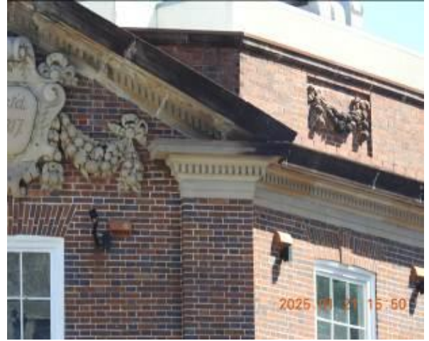
Figure 160 - General condition of external wall
