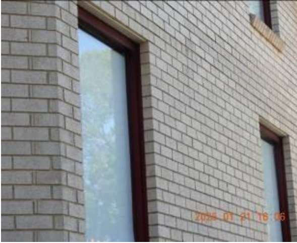
Figure 279 - General condition of external wall
