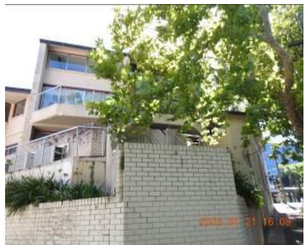
Figure 308 - General condition of external wall
