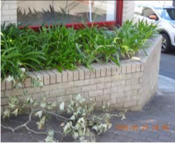
Figure 273 - General condition of retaining wall
