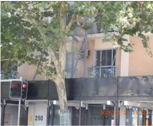
Figure 78 - General condition of external wall
