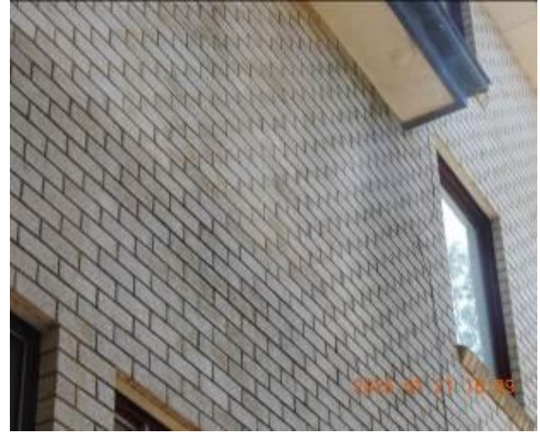
Figure 328 - General condition of external wall
