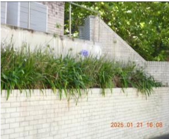
Figure 305 - General condition of external wall
