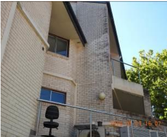
Figure 295 - General condition of external wall
