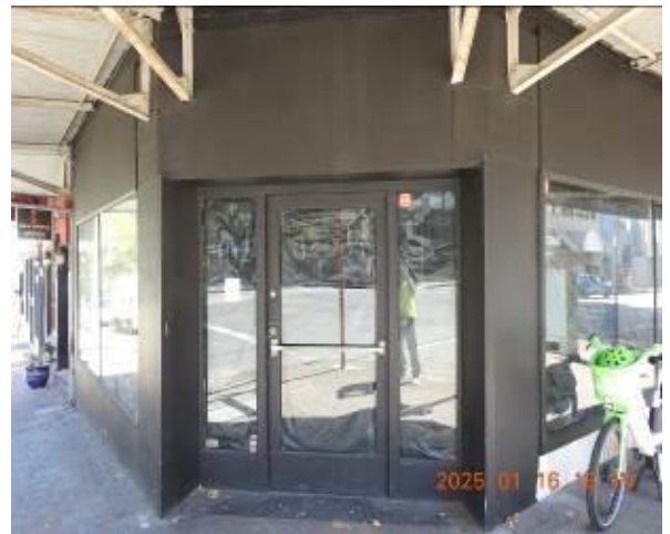
Figure 50 - General condition of external wall
