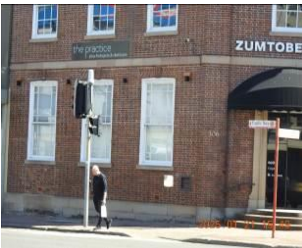
Figure 139 - General condition of external wall
