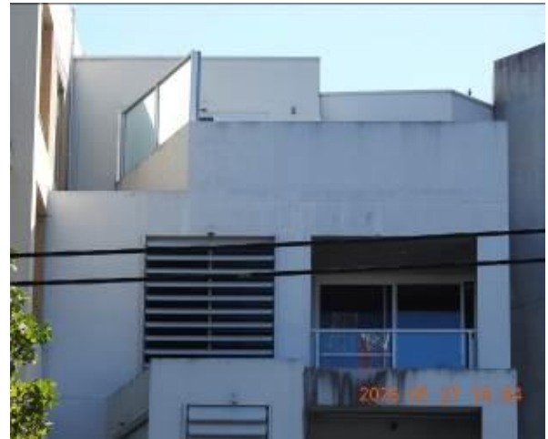
Figure 103 - General condition of external wall
