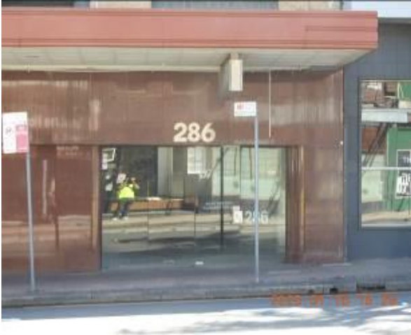
Figure 133 - General condition of external wall
