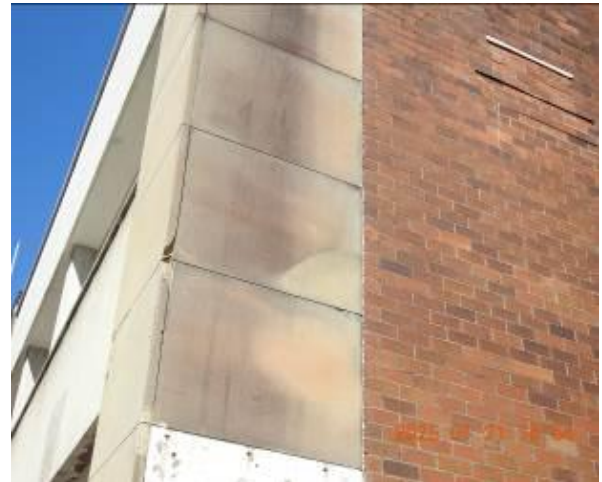
Figure 204 - General condition of external wall
