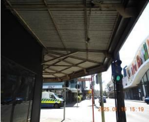
Figure 53 - General condition of awning
