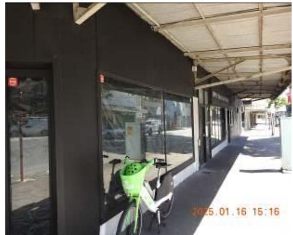
Figure 38 - General condition of external wall
