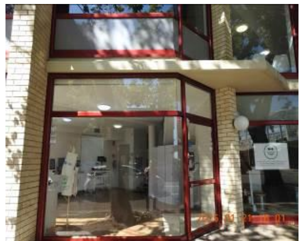
Figure 224 - General condition of external wall
