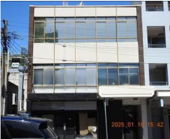
Figure 33 - General condition of external wall
