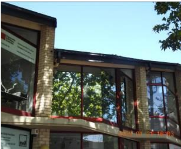
Figure 245 - General condition of external wall
