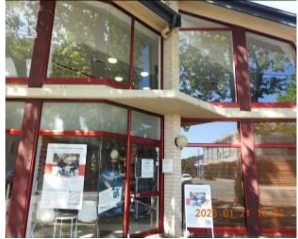
Figure 232 - General condition of external wall
