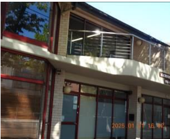
Figure 235 - General condition of external wall
