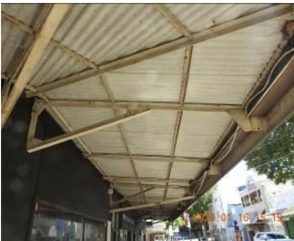
Figure 51 - General condition of awning
