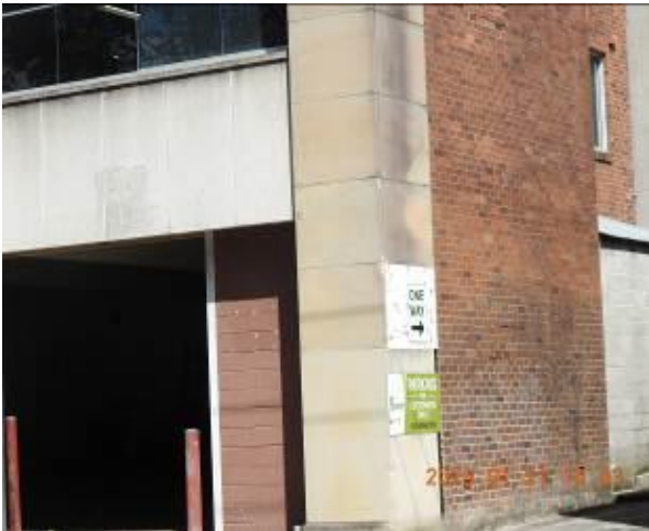
Figure 185 - General condition of external wall
