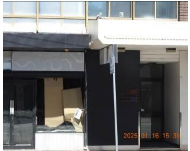
Figure 12 - General condition of external wall
