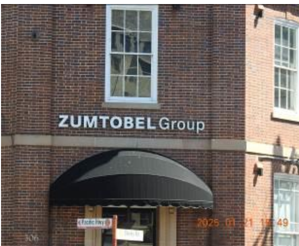
Figure 151 - General condition of external wall
