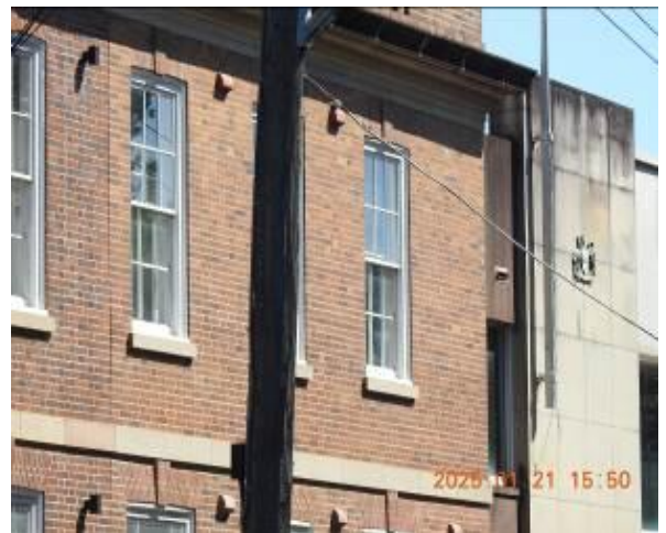
Figure 164 - General condition of external wall
