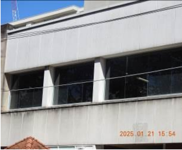
Figure 195 - General condition of external wall
