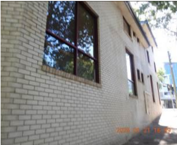
Figure 317 - General condition of external wall
