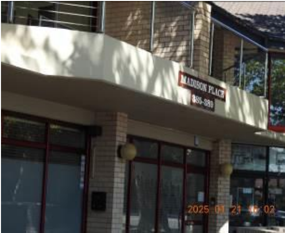
Figure 237 - General condition of external wall
