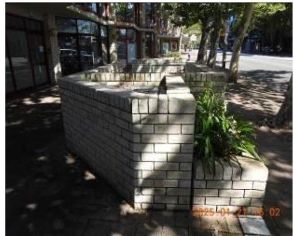
Figure 240 - General condition of external wall
