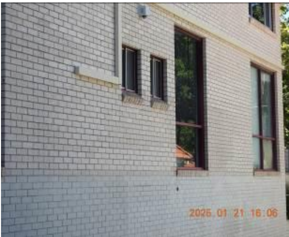
Figure 287 - General condition of external wall
