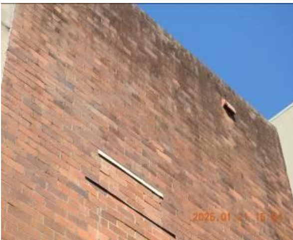
Figure 199 - General condition of external wall
