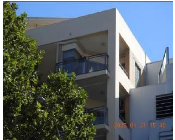
Figure 79 - General condition of external wall
