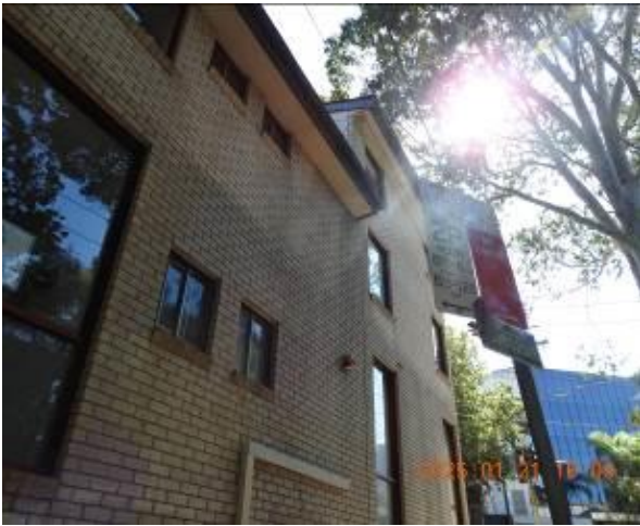
Figure 323 - General condition of external wall
