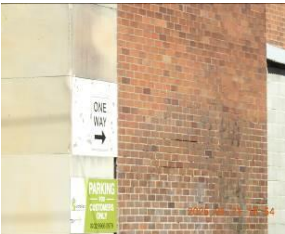
Figure 193 - General condition of external wall
