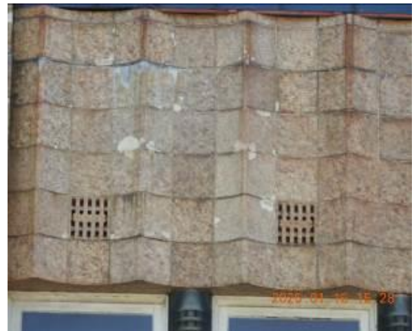
Figure 130 - General condition of external wall
