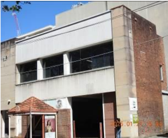
Figure 197 - General condition of external wall
