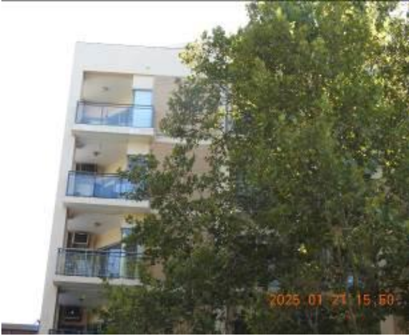
Figure 88 - General condition of external wall
