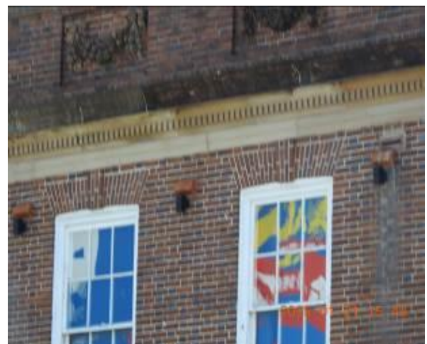
Figure 146 - General condition of external wall
