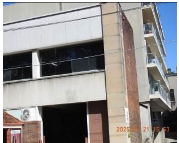
Figure 182 - General condition of external wall
