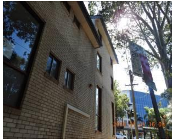
Figure 324 - General condition of external wall
