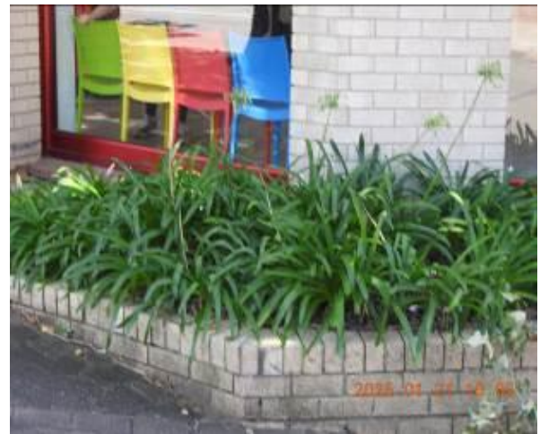
Figure 270 - General condition of retaining wall
