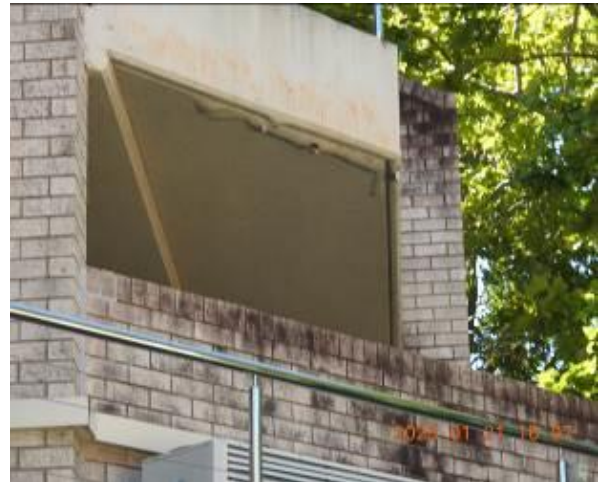
Figure 300 - General condition of external wall
