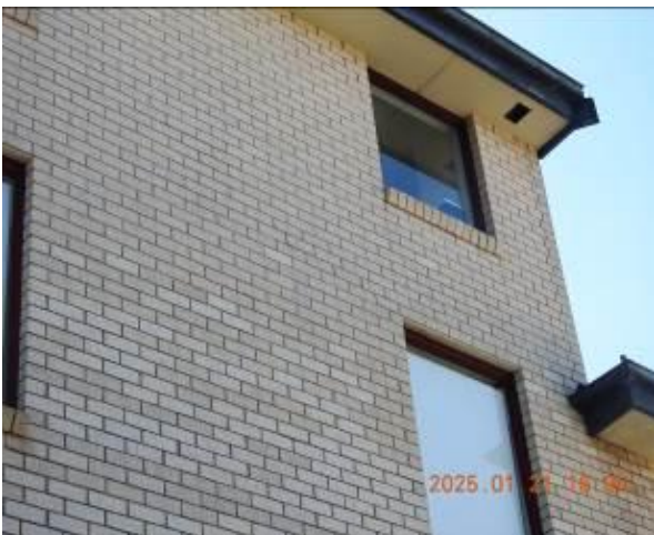
Figure 283 - General condition of external wall
