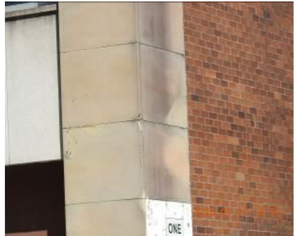
Figure 186 - General condition of external wall
