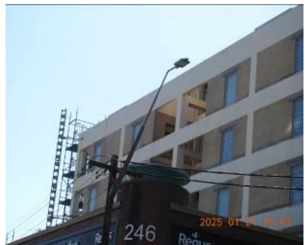
Figure 99 - General condition of external wall
