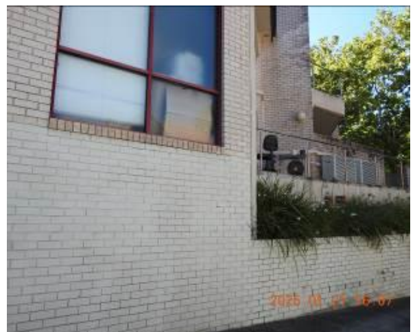
Figure 290 - General condition of external wall
