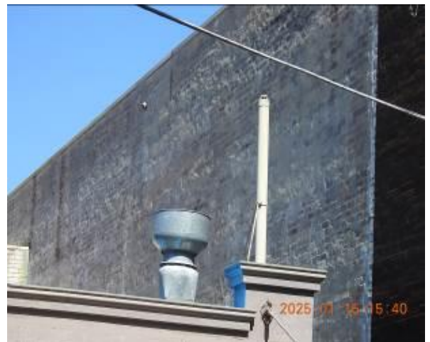
Figure 24 - General condition of external wall
