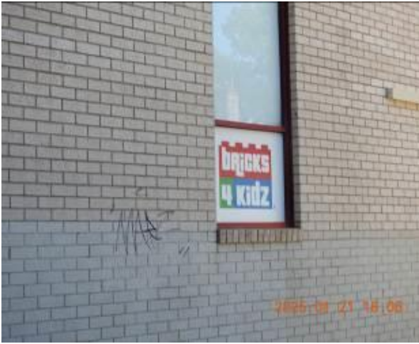
Figure 285 - General condition of external wall
