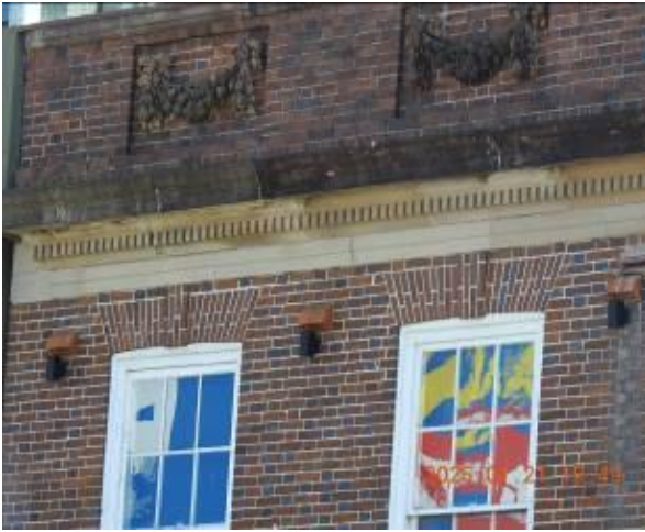
Figure 141 - General condition of external wall
