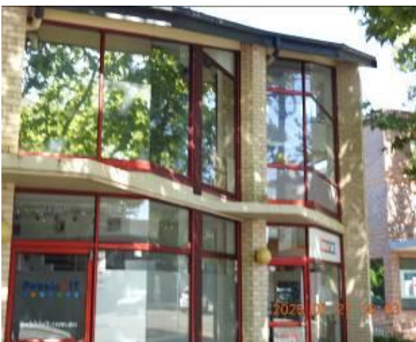
Figure 247 - General condition of external wall
