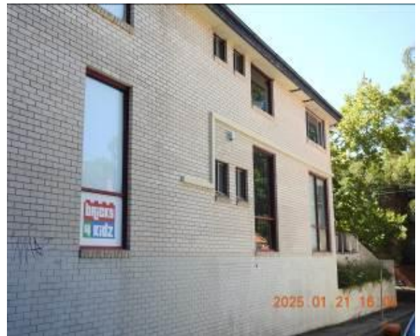
Figure 288 - General condition of external wall
