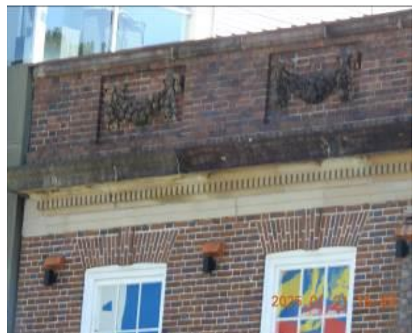
Figure 140 - General condition of external wall
