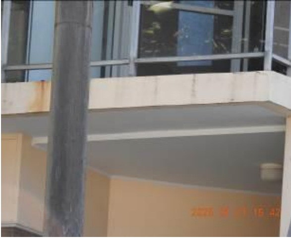
Figure 118 - General condition of external wall
