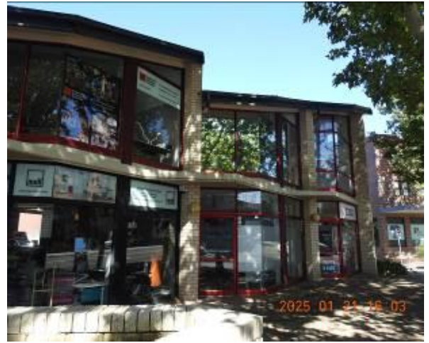
Figure 244 - General condition of external wall
