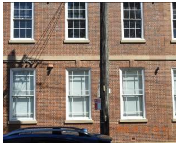
Figure 170 - General condition of external wall
