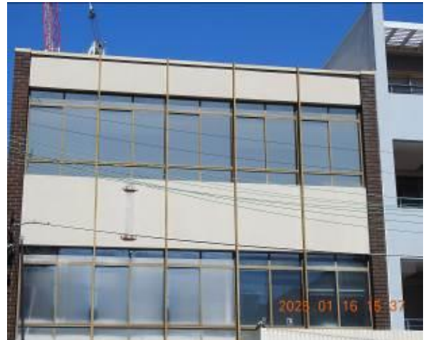
Figure 4 - General condition of external wall
