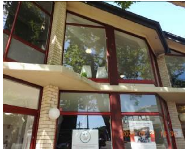
Figure 228 - General condition of external wall
