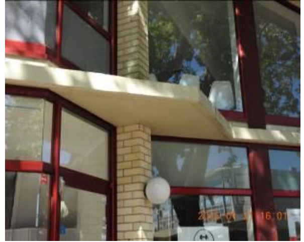
Figure 226 - General condition of external wall
