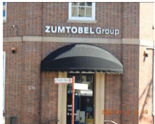
Figure 152 - General condition of external wall
