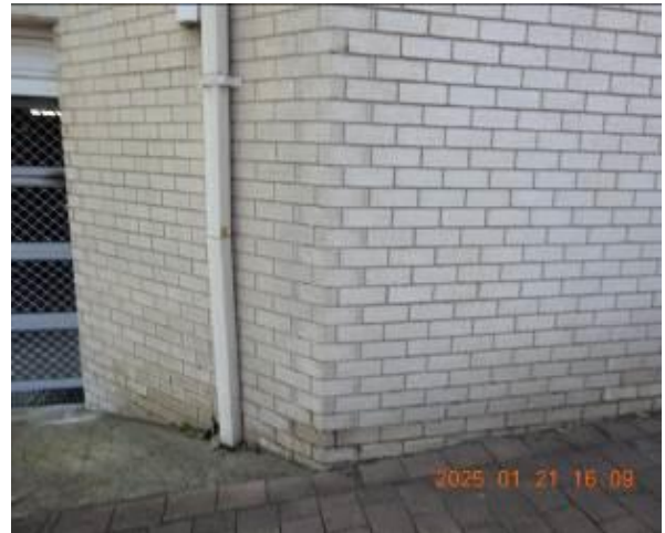
Figure 318 - General condition of external wall
