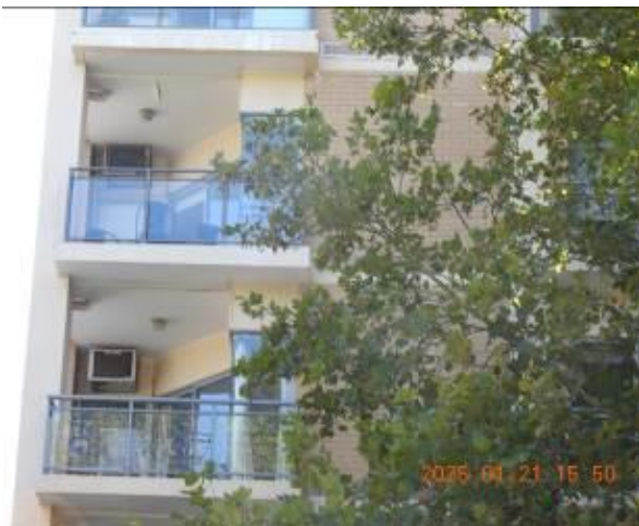
Figure 90 - General condition of external wall
