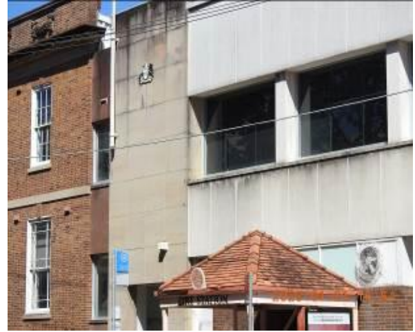
Figure 196 - General condition of external wall
