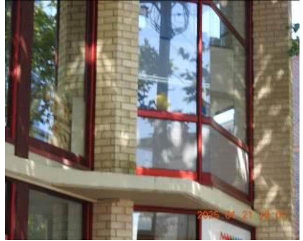
Figure 250 - General condition of external wall
