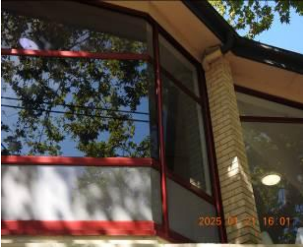
Figure 225 - General condition of external wall
