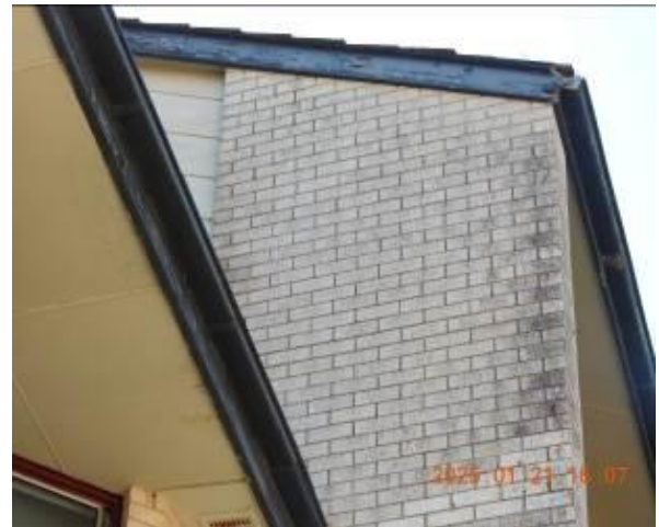
Figure 296 - General condition of external wall
