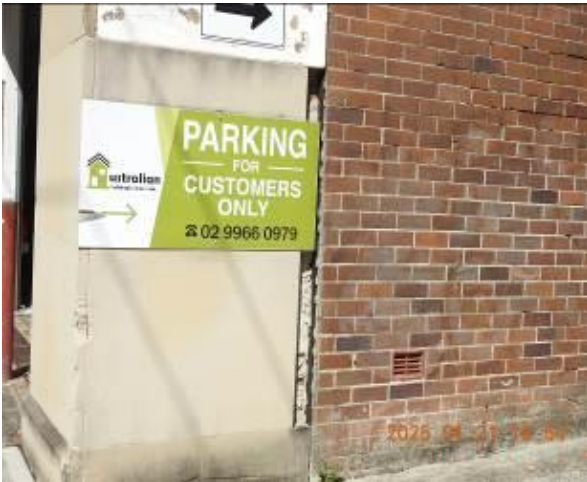
Figure 203 - General condition of external wall
