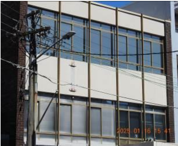
Figure 27 - General condition of external wall
