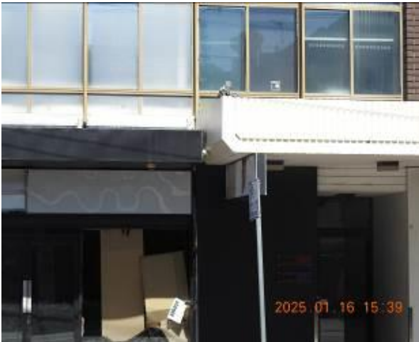
Figure 11 - General condition of external wall
