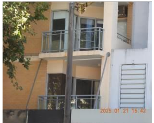
Figure 81 - General condition of external wall
