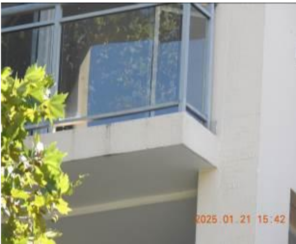
Figure 120 - General condition of external wall
