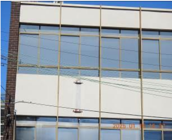
Figure 3 - General condition of external wall
