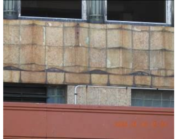
Figure 128 - General condition of external wall
