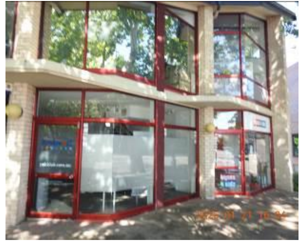
Figure 256 - General condition of external wall
