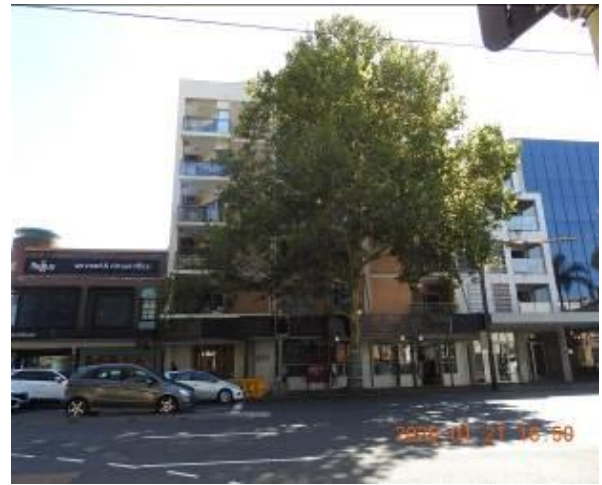
Figure 85 - General condition of external wall
