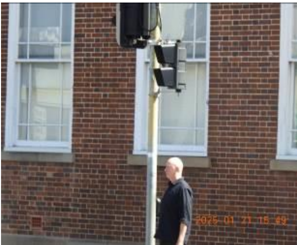
Figure 143 - General condition of external wall
