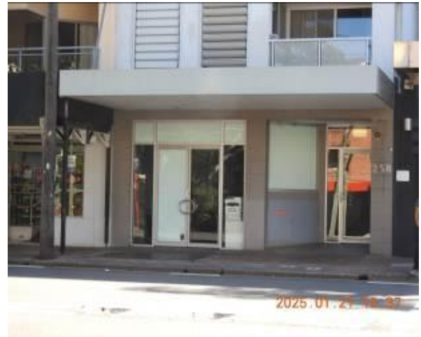
Figure 109 - General condition of external wall
