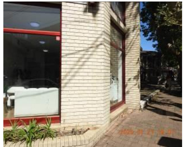
Figure 222 - General condition of external wall
