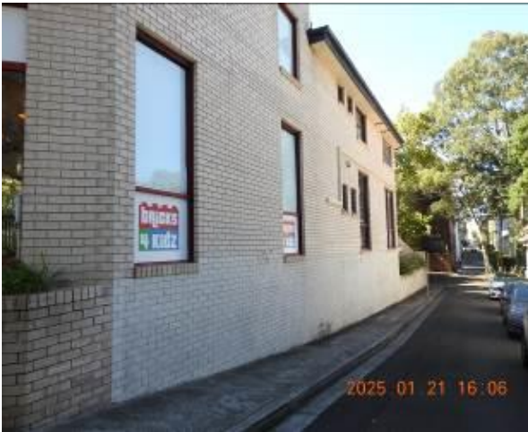
Figure 281 - General condition of external wall
