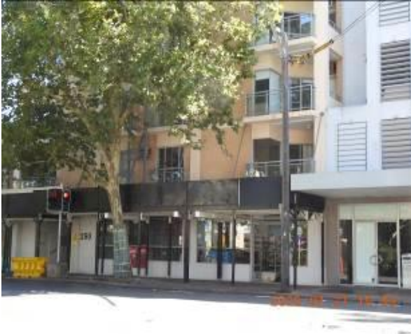
Figure 70 - General condition of external wall
