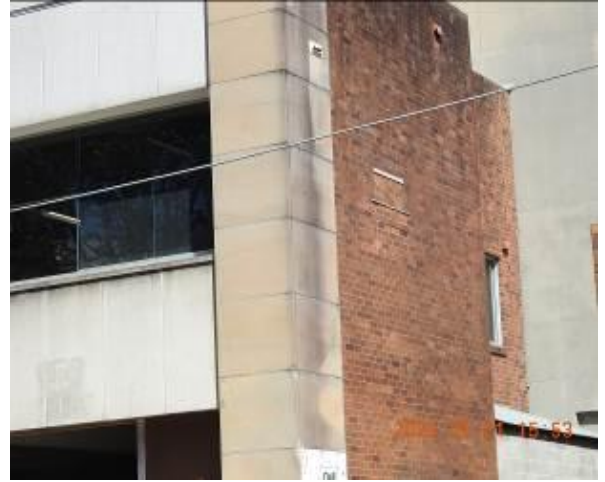
Figure 184 - General condition of external wall
