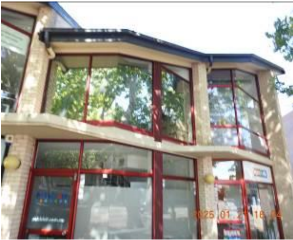
Figure 257 - General condition of external wall
