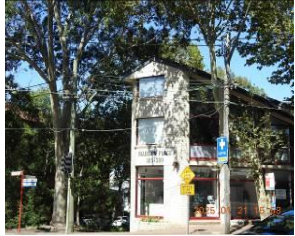
Figure 208 - General condition of external wall
