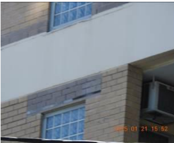
Figure 96 - General condition of external wall
