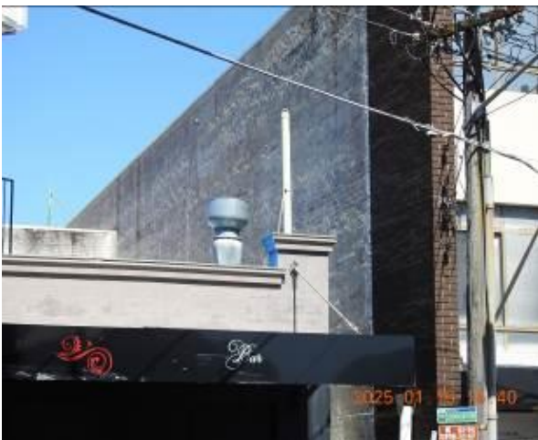
Figure 23 - General condition of external wall
