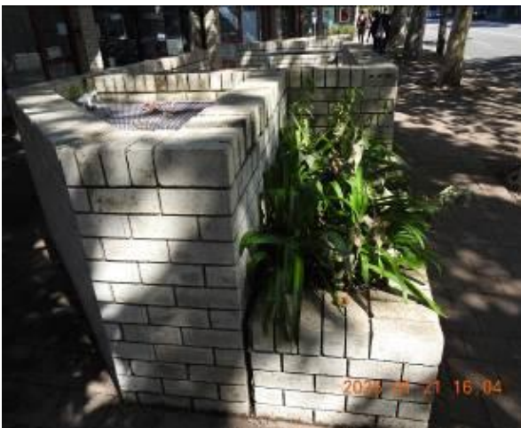
Figure 265 - General condition of retaining wall
