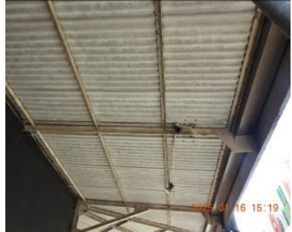
Figure 54 - General condition of awning
