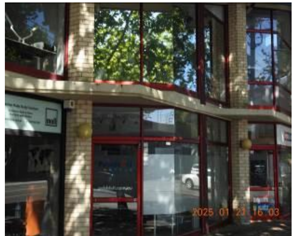
Figure 246 - General condition of external wall
