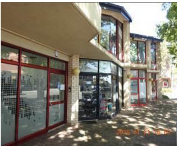
Figure 241 - General condition of external wall
