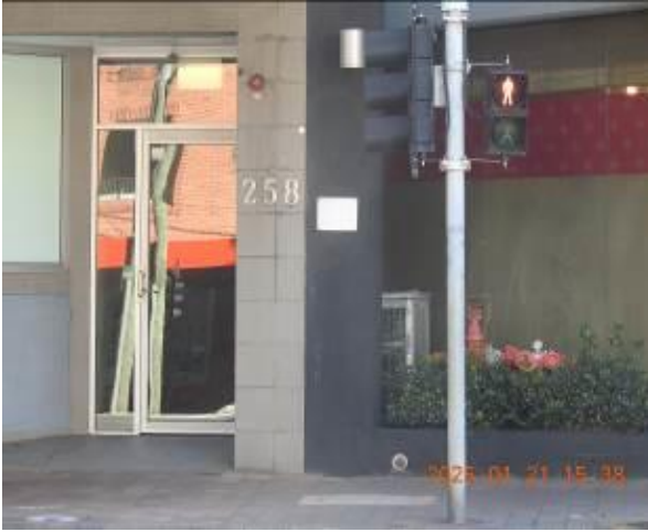
Figure 112 - General condition of external wall
