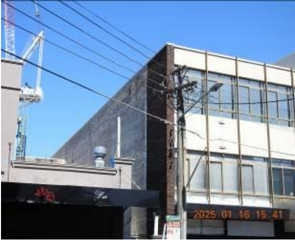
Figure 31 - General condition of external wall
