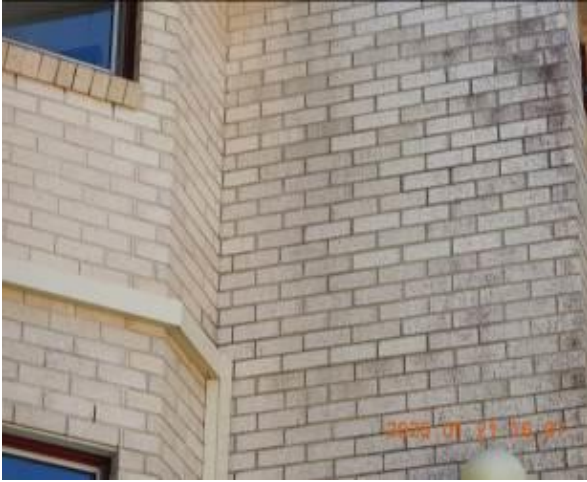
Figure 297 - General condition of external wall
