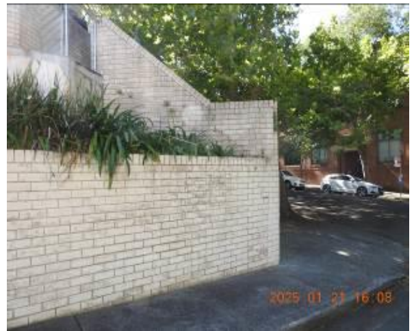
Figure 306 - General condition of external wall
