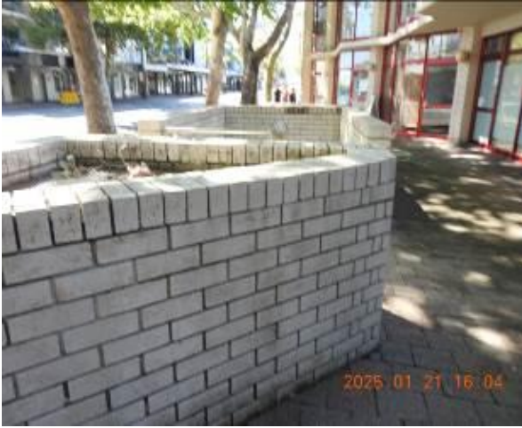
Figure 261 - General condition of retaining wall
