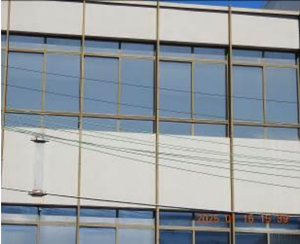
Figure 13 - General condition of external wall
