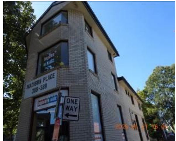
Figure 276 - General condition of external wall
