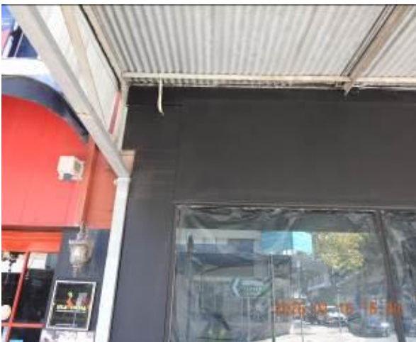
Figure 57 - General condition of awning
