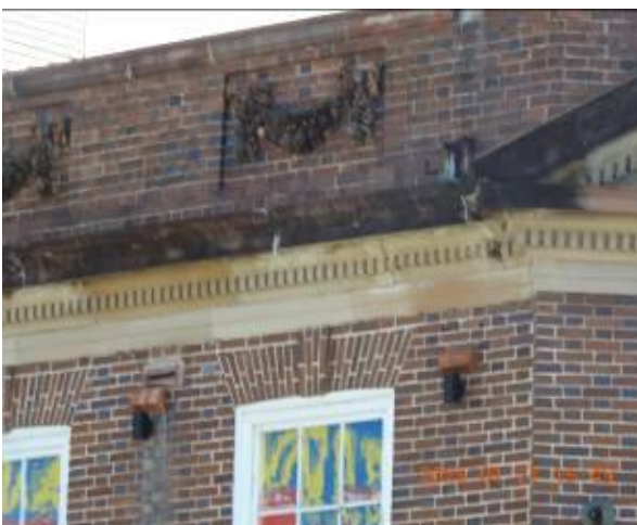
Figure 145 - General condition of external wall
