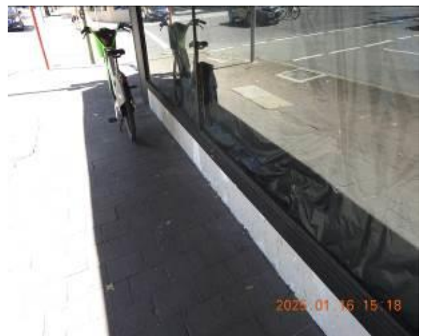
Figure 46 - General condition of external wall
