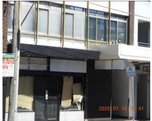
Figure 28 - General condition of external wall
