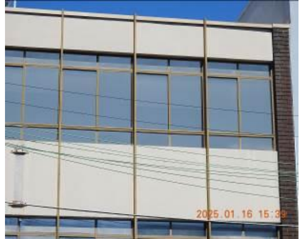
Figure 14 - General condition of external wall
