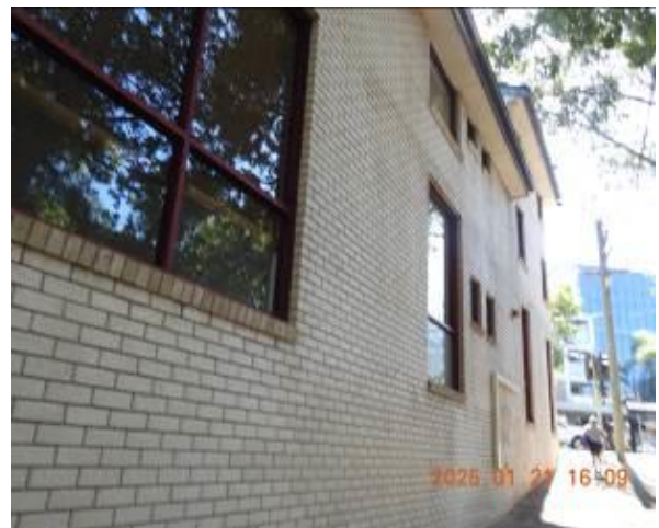
Figure 320 - General condition of external wall
