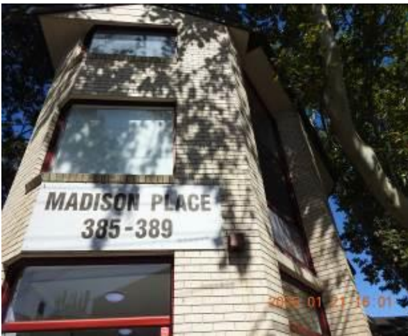
Figure 221 - General condition of external wall
