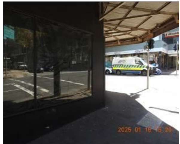
Figure 56 - General condition of external wall
