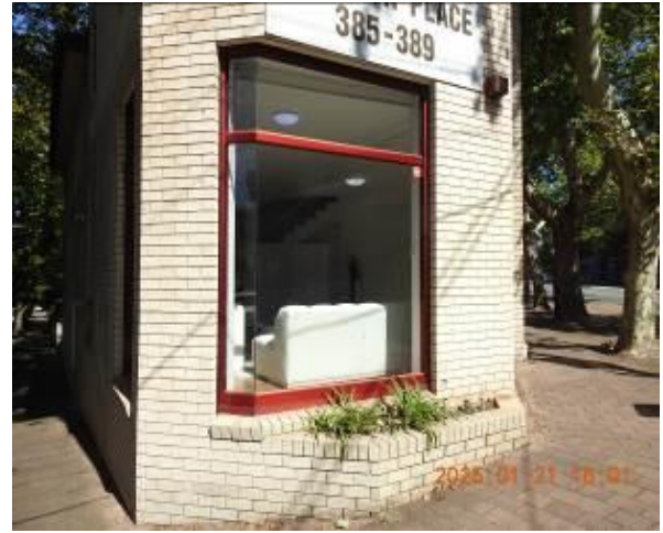
Figure 220 - General condition of external wall
