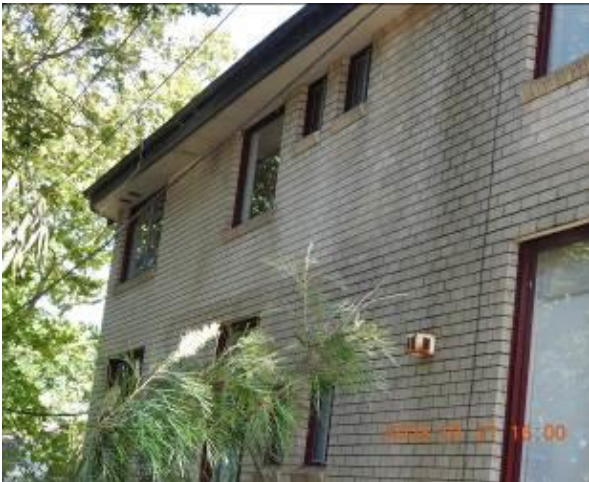
Figure 215 - General condition of external wall
