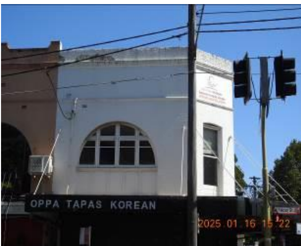
Figure 63 - - General condition of external wall
