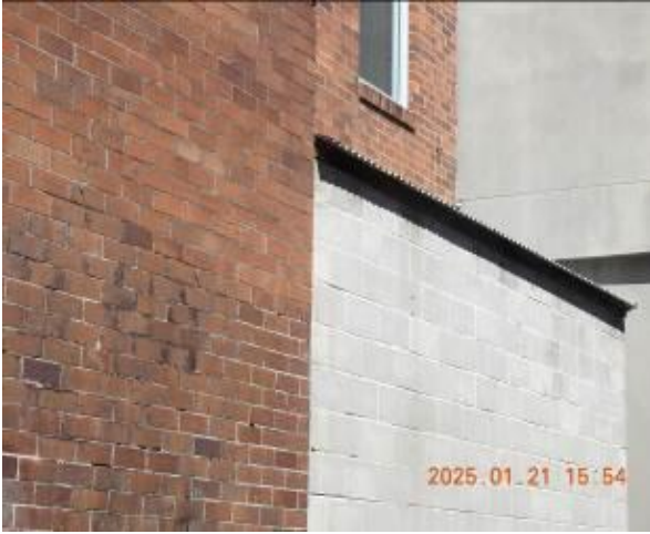
Figure 201 - General condition of external wall
