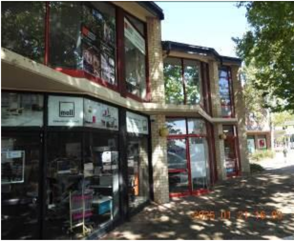
Figure 243 - General condition of external wall
