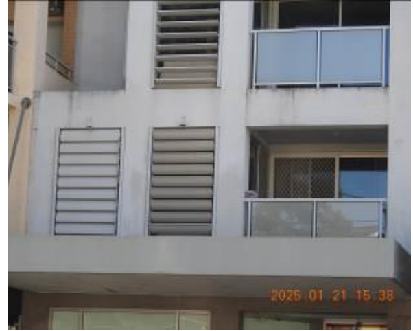
Figure 113 - General condition of external wall
