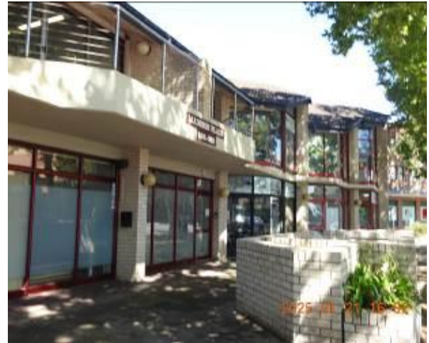
Figure 238 - General condition of external wall
