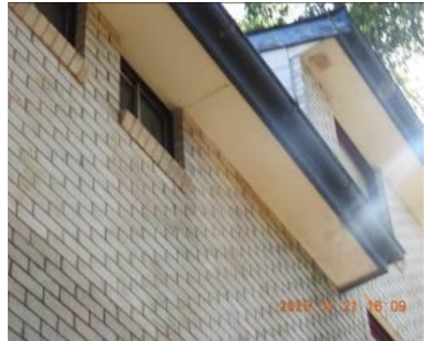
Figure 330 - General condition of external wall
