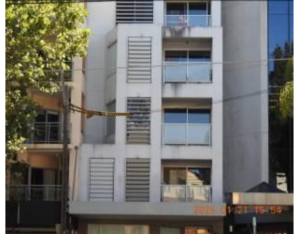
Figure 101 - General condition of external wall
