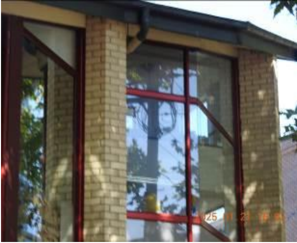
Figure 249 - General condition of external wall
