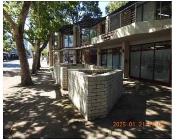
Figure 258 - General condition of external wall
