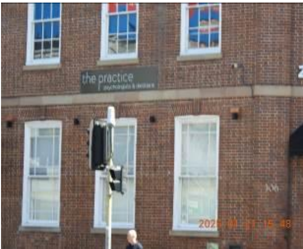
Figure 137 - General condition of external wall
