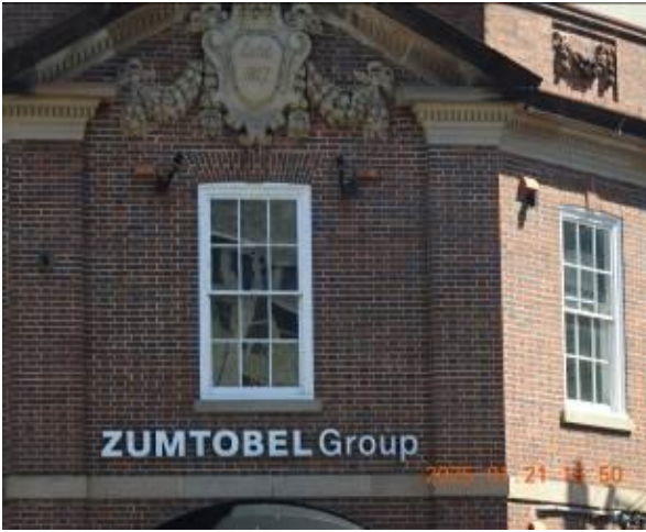
Figure 153 - General condition of external wall
