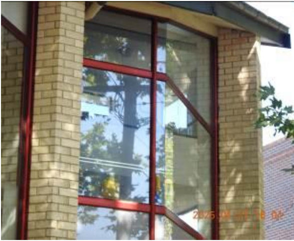
Figure 255 - General condition of external wall
