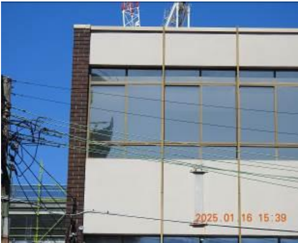
Figure 15 - General condition of external wall
