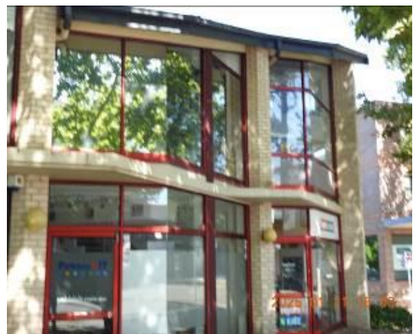
Figure 248 - General condition of external wall
