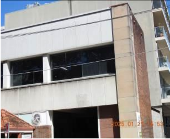
Figure 183 - General condition of external wall
