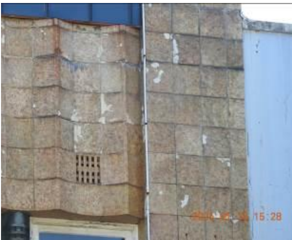
Figure 131 - General condition of external wall
