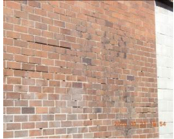
Figure 202 - General condition of external wall
