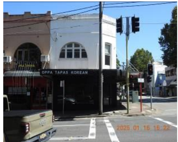
Figure 62 - General condition of external wall
