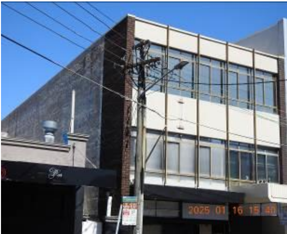
Figure 17 - General condition of external wall
