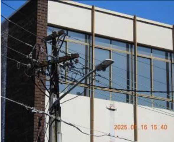
Figure 19 - General condition of external wall
