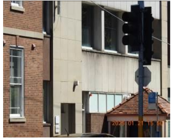
Figure 166 - General condition of external wall
