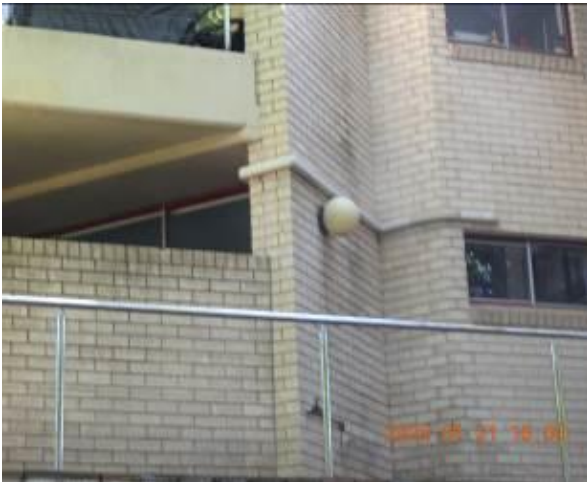
Figure 311 - General condition of external wall
