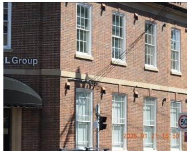
Figure 158 - General condition of external wall
