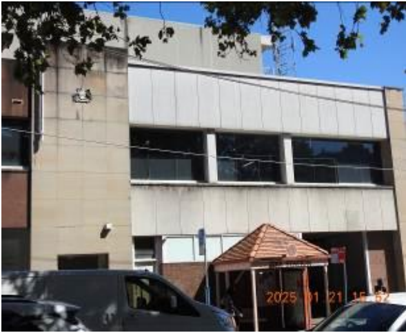
Figure 177 - General condition of external wall
