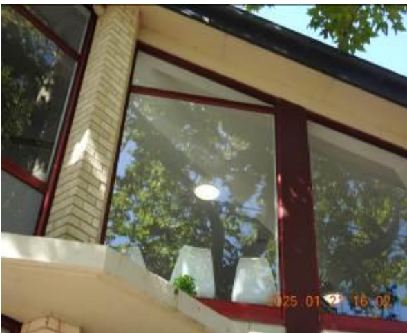
Figure 229 - General condition of external wall
