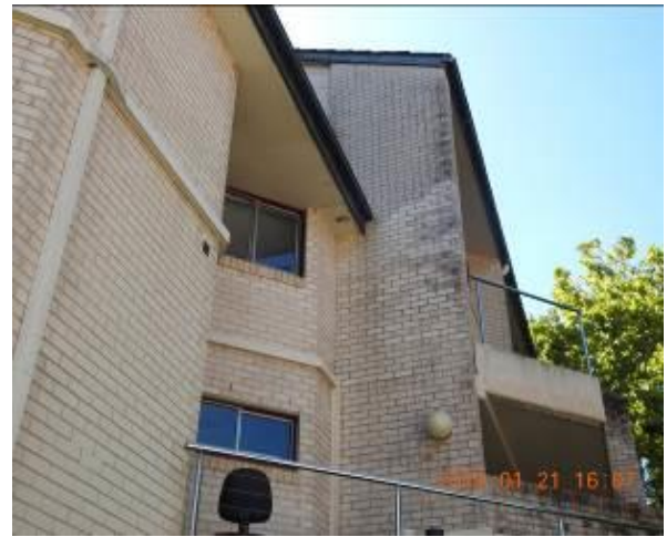
Figure 294 - General condition of external wall
