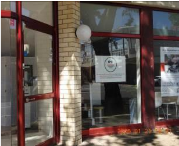
Figure 227 - General condition of external wall
