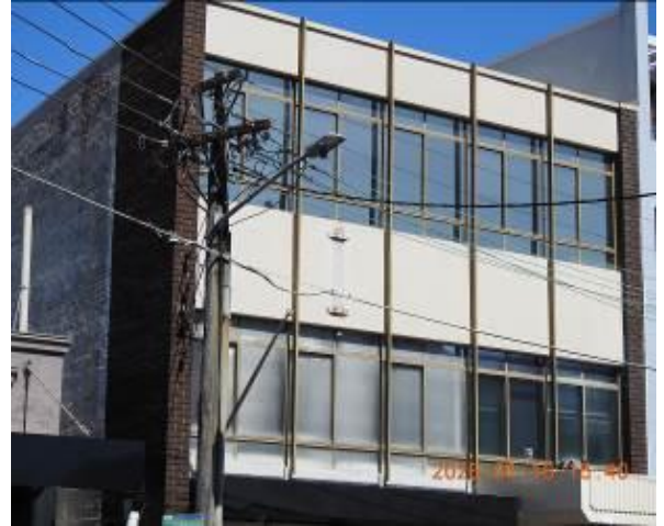
Figure 20 - General condition of external wall
