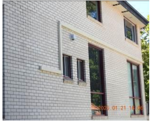
Figure 286 - General condition of external wall
