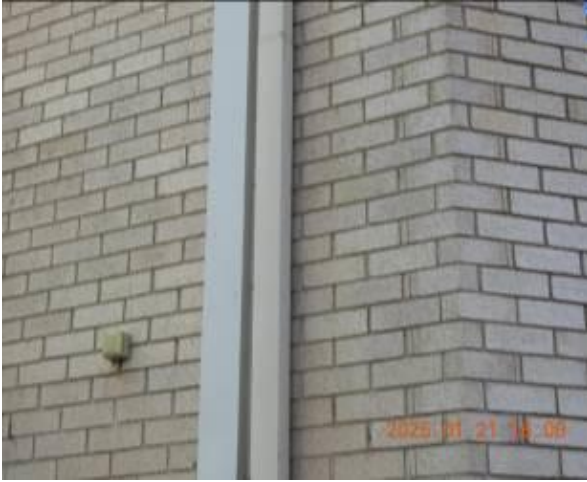
Figure 315 - General condition of external wall
