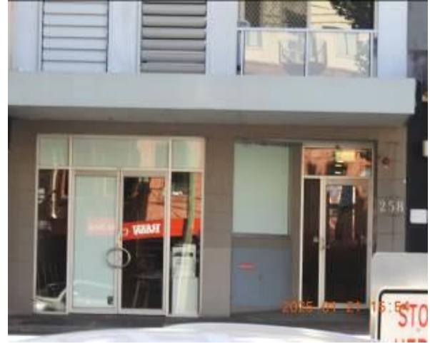
Figure 107 - General condition of external wall
