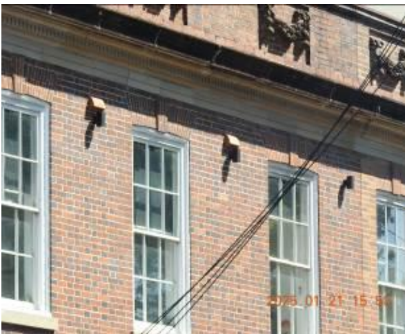
Figure 157 - General condition of external wall
