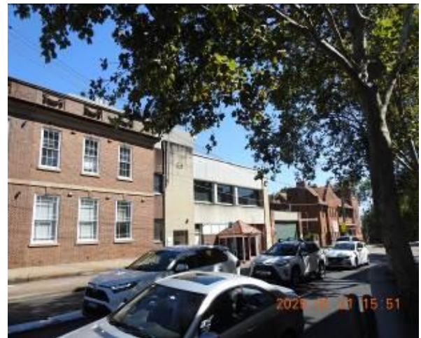
Figure 168 - General condition of external wall
