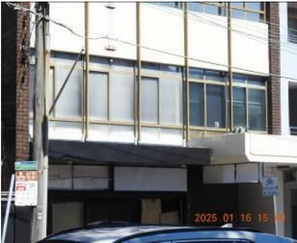
Figure 21 - General condition of external wall
