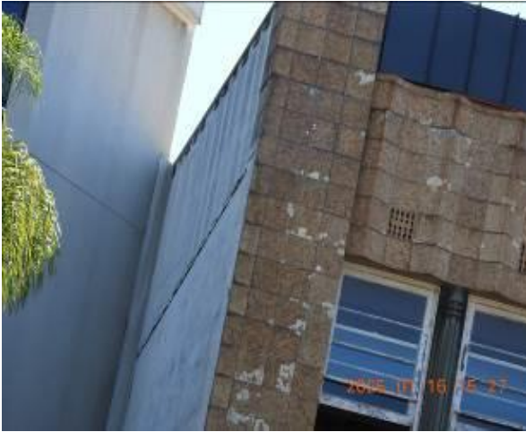
Figure 123 - General condition of external wall
