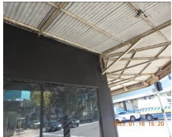
Figure 58 - General condition of awning
