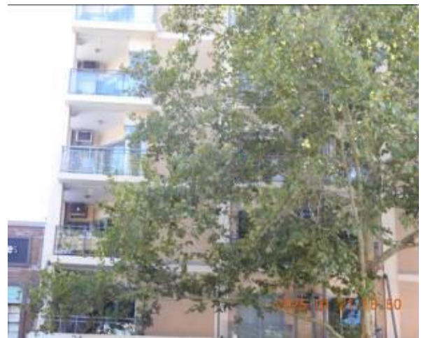
Figure 87 - General condition of external wall
