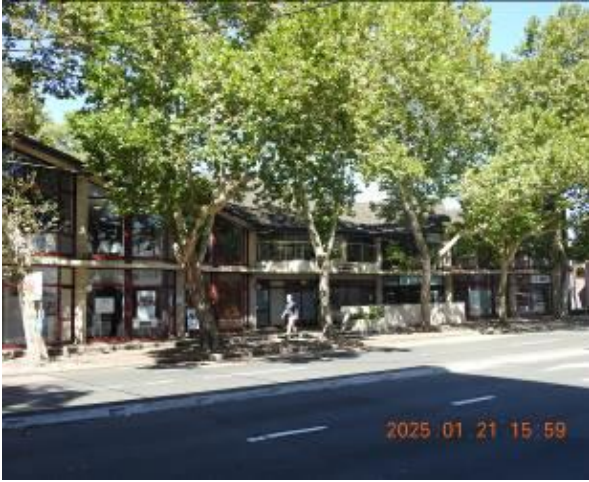
Figure 213 - General condition of external wall
