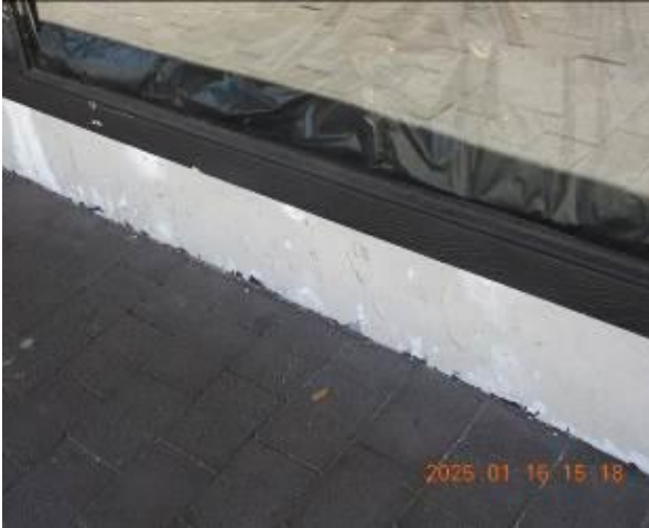
Figure 47 - General condition of external wall
