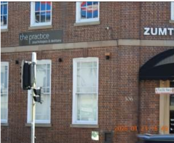
Figure 149 - General condition of external wall
