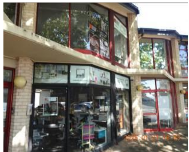
Figure 242 - General condition of external wall
