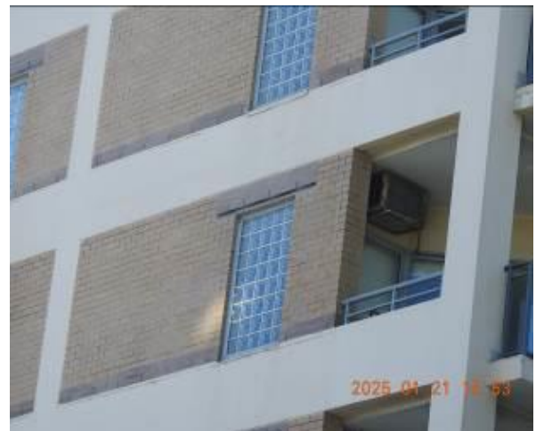
Figure 97 - General condition of external wall
