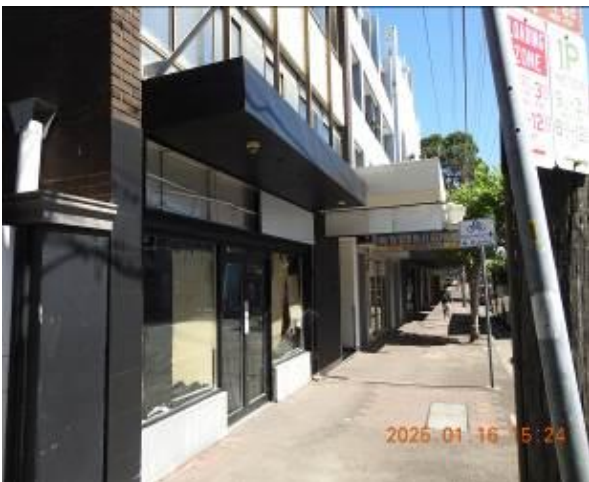
Figure 69 - - General condition of external wall
