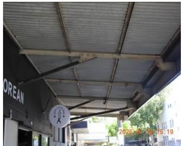
Figure 52 - General condition of awning
