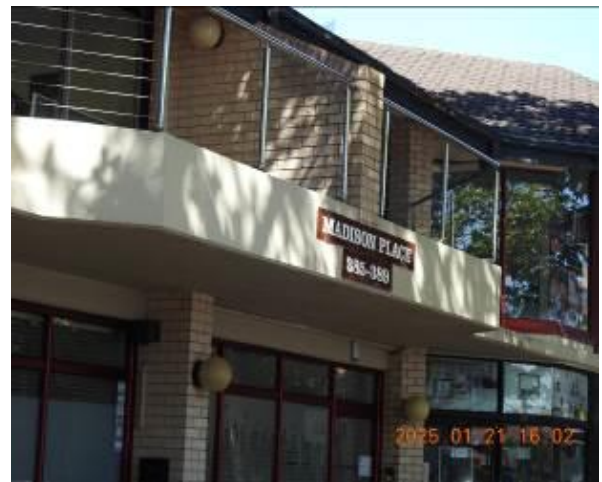
Figure 236 - General condition of external wall
