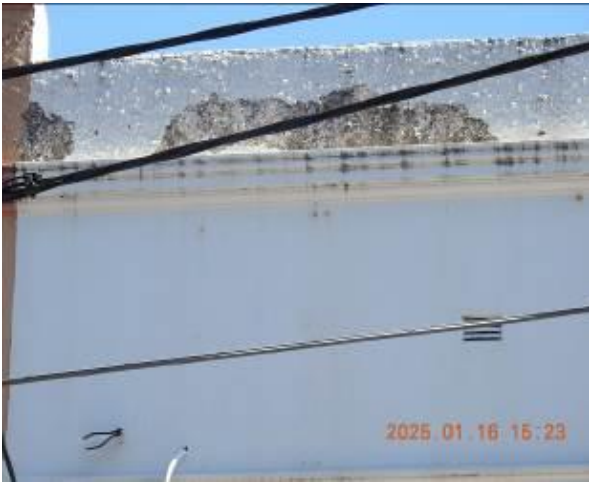
Figure 67 - - General condition of external wall
