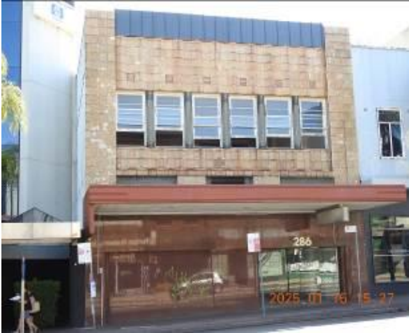
Figure 121 – The following images displays the general condition of 286 Pacific Highway
