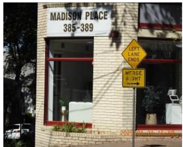
Figure 212 - General condition of external wall
