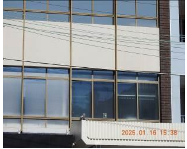
Figure 8 - General condition of external wall
