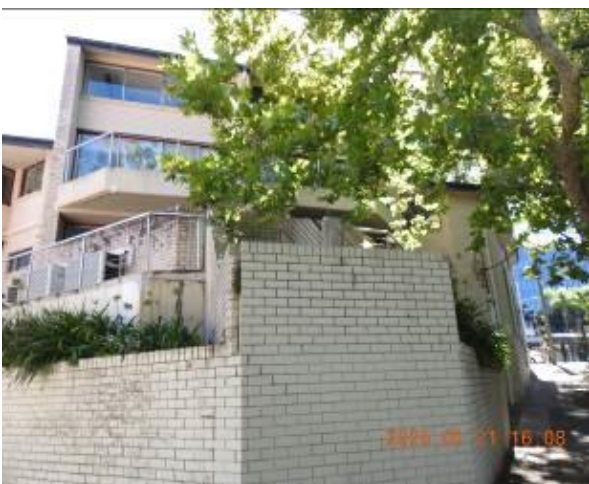
Figure 307 - General condition of external wall
