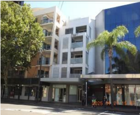
Figure 108 - General condition of external wall
