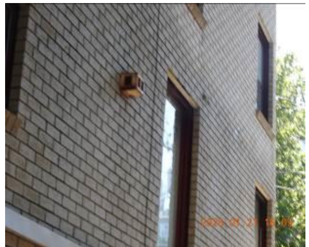
Figure 326 - General condition of external wall
