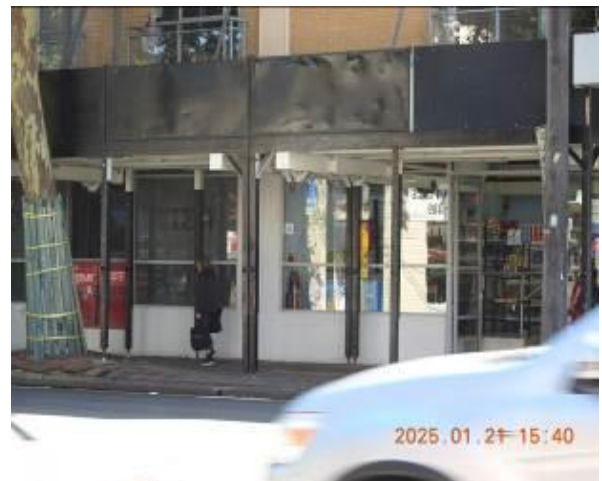
Figure 75 - General condition of external wall
