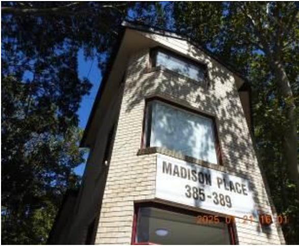
Figure 219 - General condition of external wall
