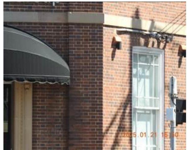
Figure 156 - General condition of external wall
