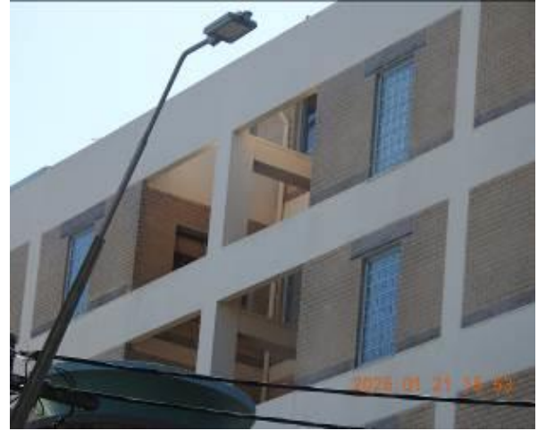
Figure 83 - General condition of external wall
