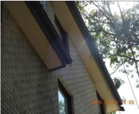
Figure 329 - General condition of external wall
