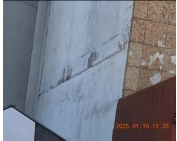
Figure 124 - General condition of external wall
