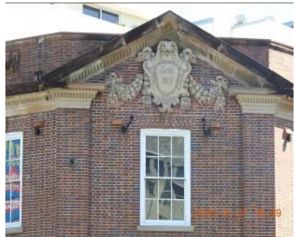
Figure 150 - General condition of external wall
