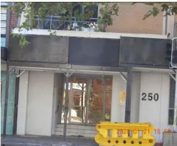
Figure 92 - General condition of external wall
