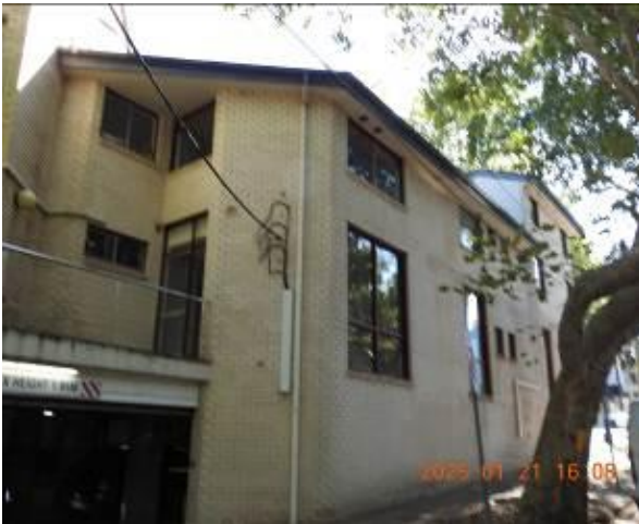
Figure 313 - General condition of external wall
