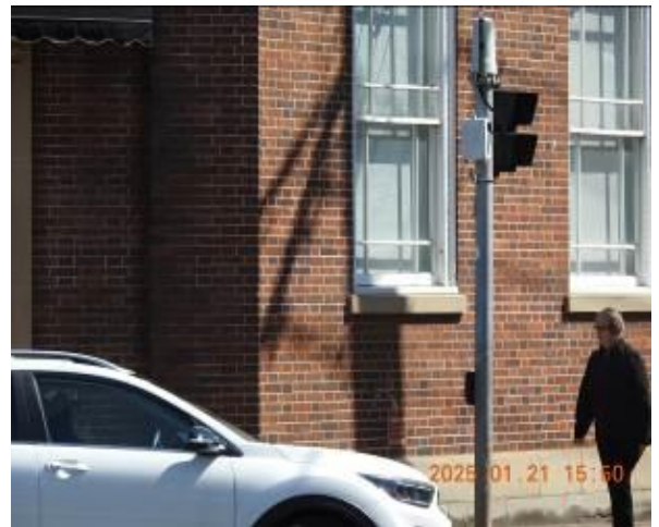
Figure 162 - General condition of external wall
