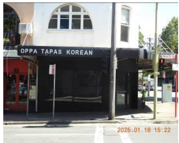
Figure 64 - - General condition of external wall
