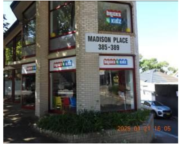
Figure 268 - General condition of external wall
