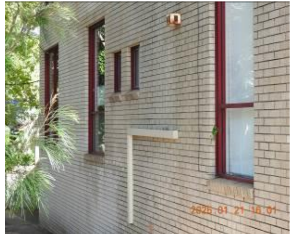
Figure 216 - General condition of external wall
