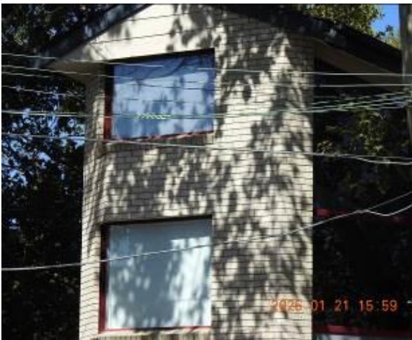
Figure 209 - General condition of external wall
