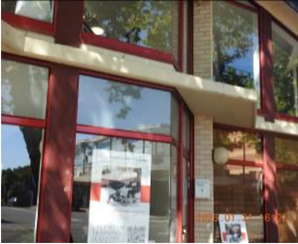
Figure 231 - General condition of external wall
