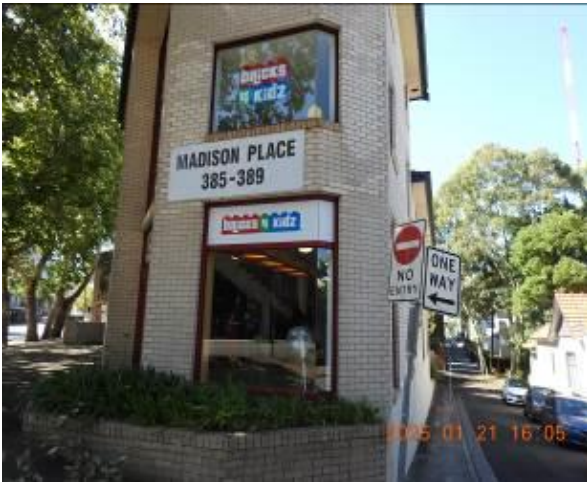
Figure 275 - General condition of external wall
