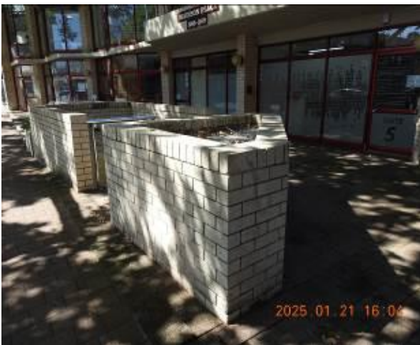
Figure 259 - General condition of retaining wall
