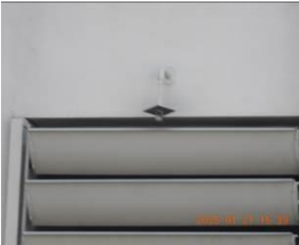
Figure 114 - General condition of external wall
