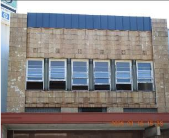
Figure 127 - General condition of external wall
