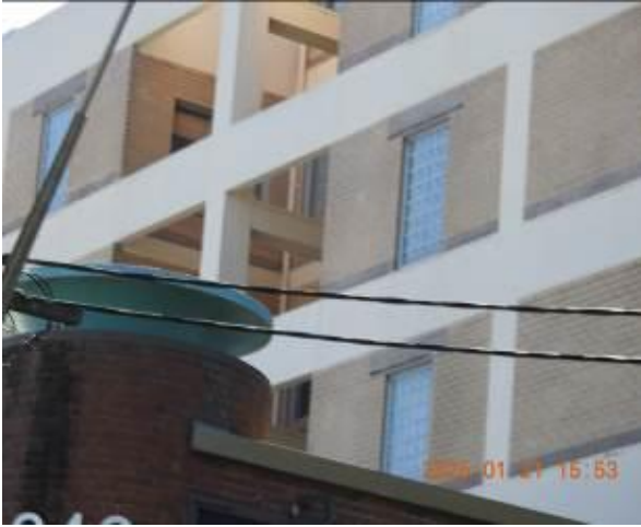
Figure 82 - General condition of external wall
