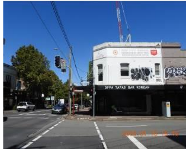
Figure 36 - General condition of external wall
