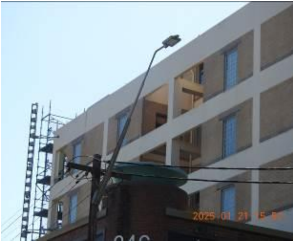
Figure 94 - General condition of external wall
