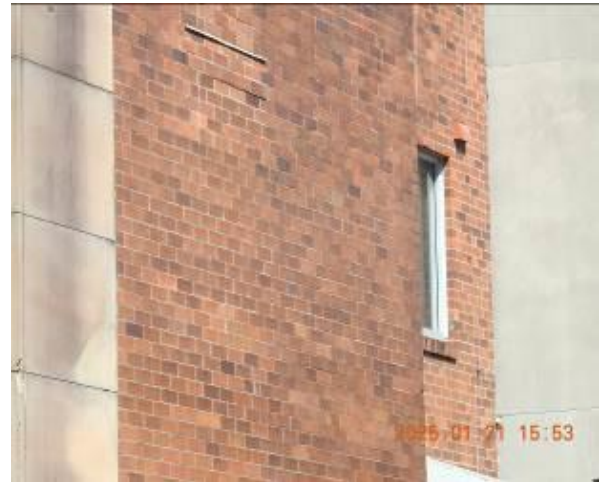
Figure 192 - General condition of external wall
