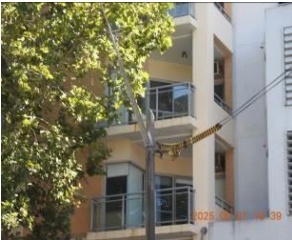
Figure 72 - General condition of external wall
