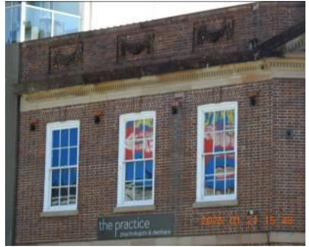
Figure 136 - General condition of external wall
