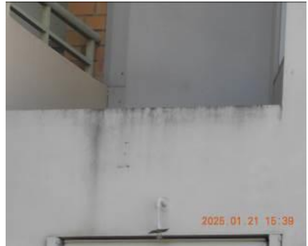
Figure 115 - General condition of external wall
