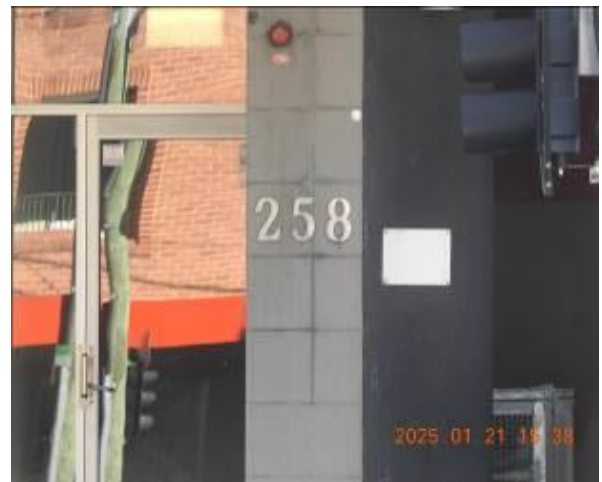
Figure 111 - General condition of external wall
