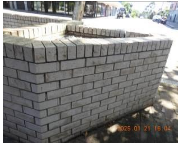
Figure 264 - General condition of external wall
