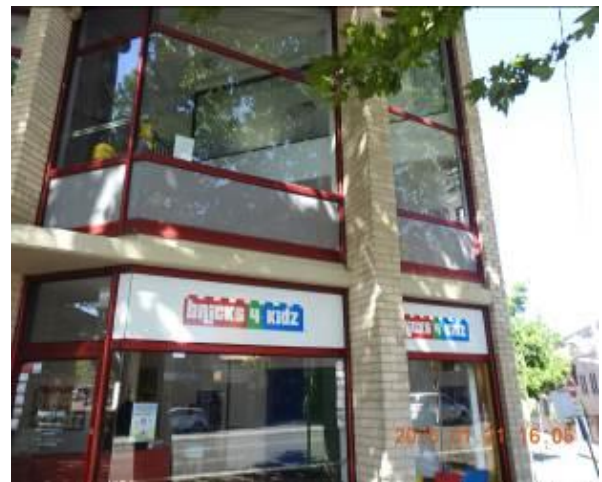
Figure 266 - General condition of external wall
