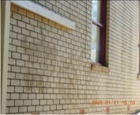
Figure 333 - General condition of external wall
