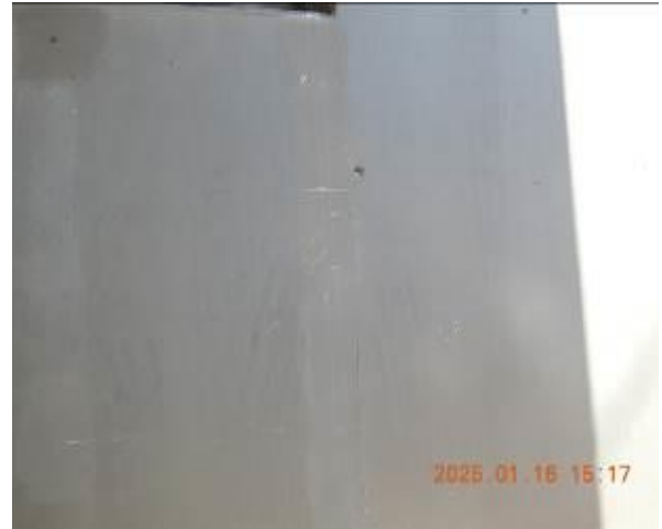
Figure 42 - General condition of external wall
