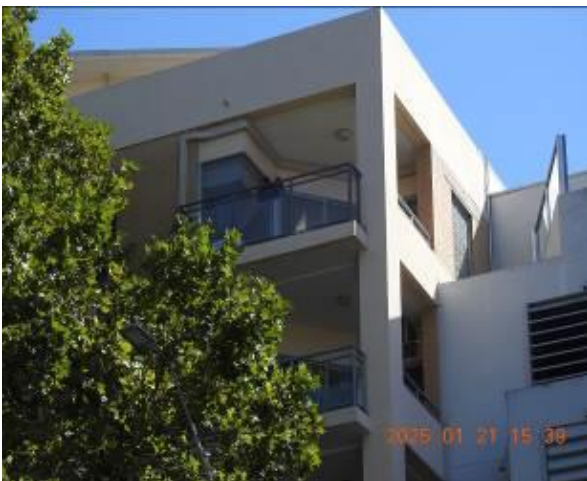
Figure 74 - General condition of external wall
