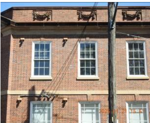
Figure 169 - General condition of external wall
