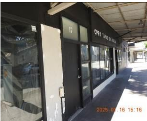
Figure 39 - General condition of external wall
