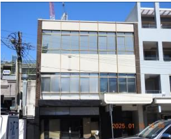
Figure 5 - General condition of external wall
