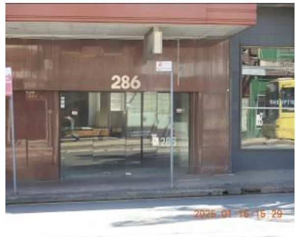
Figure 132 - General condition of external wall
