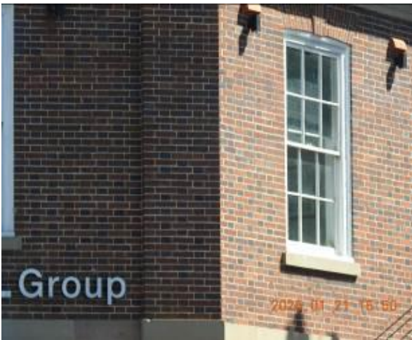
Figure 155 - General condition of external wall
