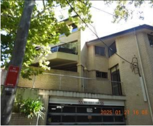
Figure 309 - General condition of external wall
