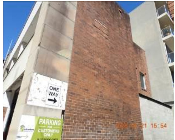
Figure 198 - General condition of external wall
