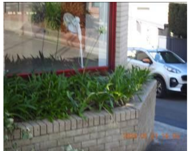
Figure 272 - General condition of retaining wall
