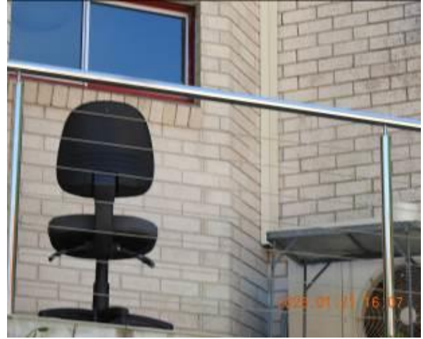
Figure 298 - General condition of external wall
