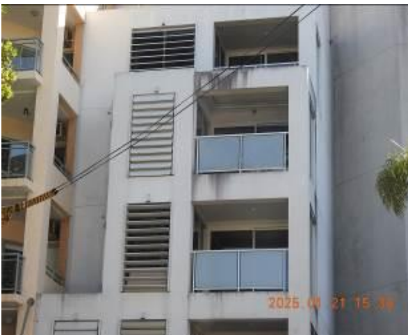
Figure 116 - General condition of external wall
