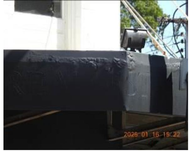
Figure 66 - - General condition of external wall
