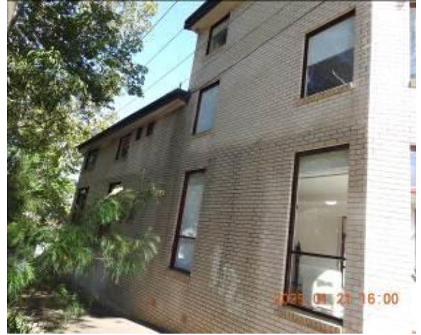
Figure 214 - General condition of external wall
