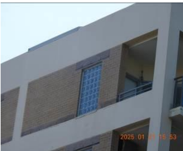
Figure 98 - General condition of external wall
