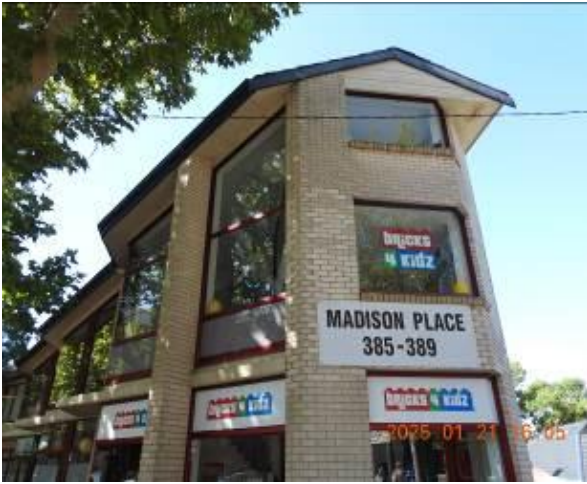
Figure 267 - General condition of external wall
