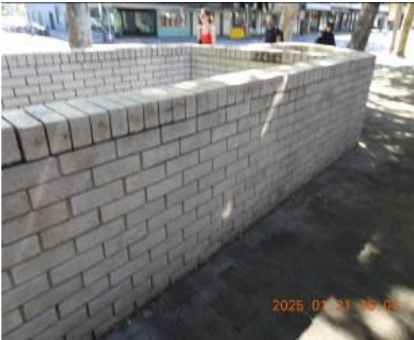
Figure 263 - General condition of external wall
