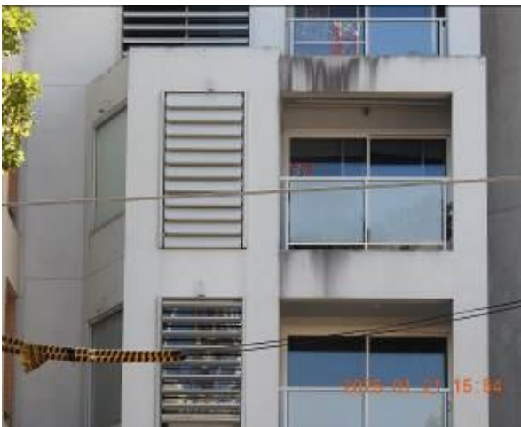
Figure 104 - General condition of external wall
