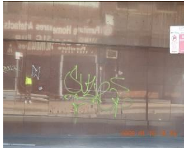
Figure 126 - General condition of external wall
