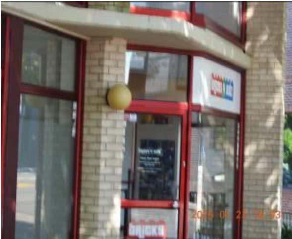
Figure 251 - General condition of external wall
