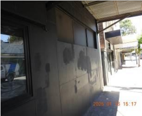
Figure 41 - General condition of external wall
