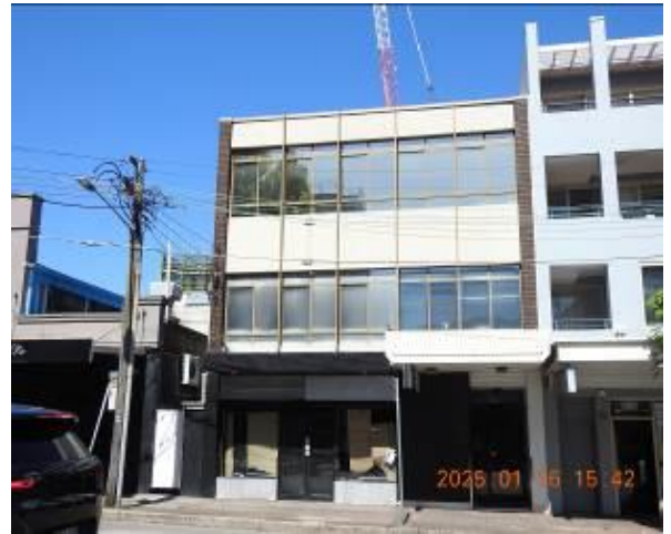
Figure 34 - General condition of external wall
