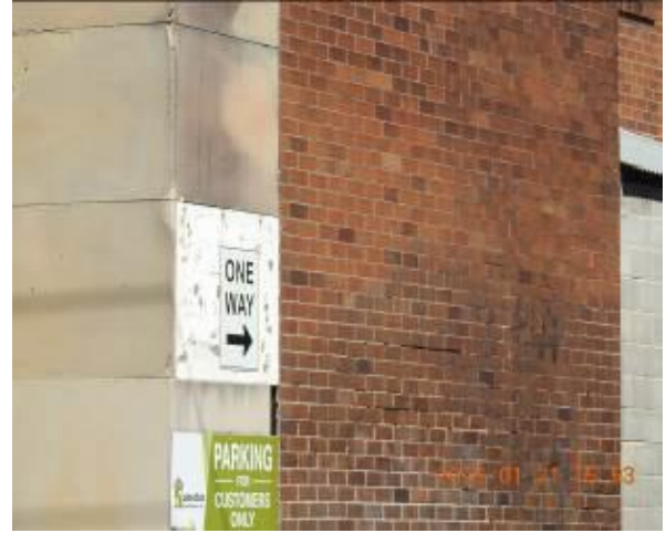
Figure 190 - General condition of external wall
