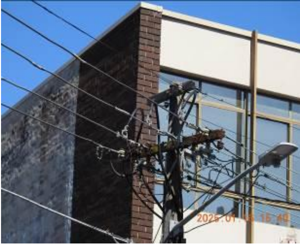
Figure 25 - General condition of external wall
