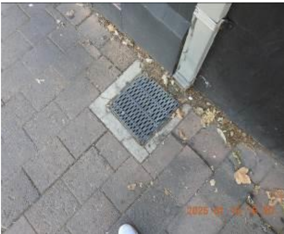
Figure 61 - General condition of service pit
