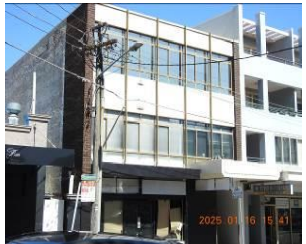
Figure 30 - General condition of external wall
