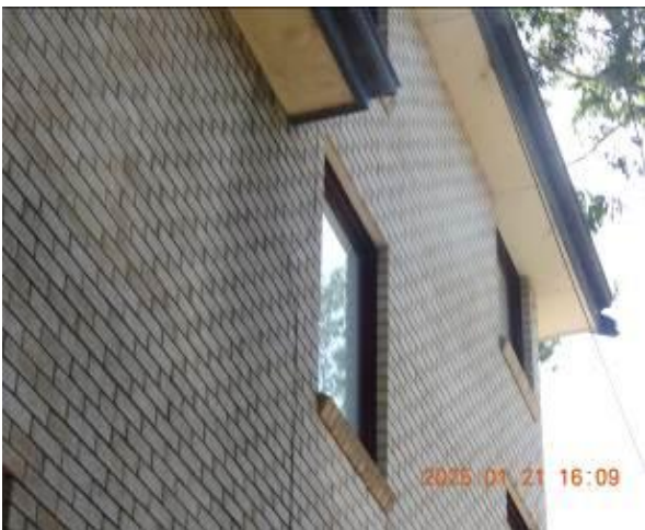
Figure 325 - General condition of external wall
