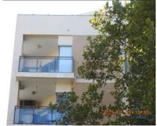
Figure 89 - General condition of external wall
