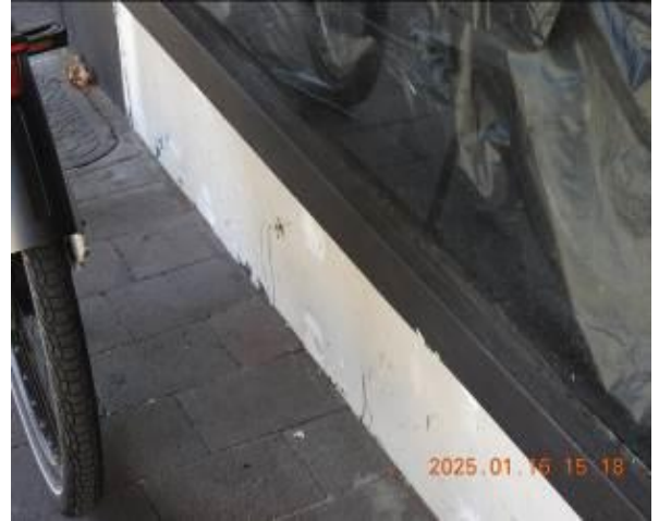
Figure 48 - General condition of external wall
