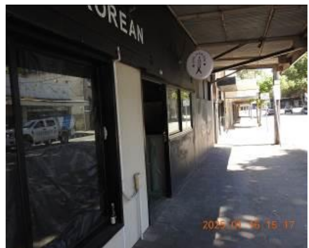
Figure 40 - General condition of external wall
