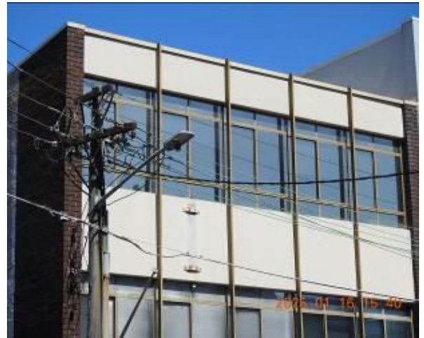
Figure 22 - General condition of external wall
