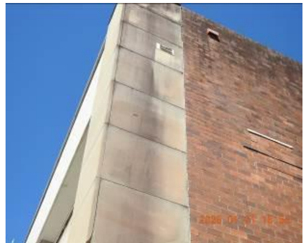
Figure 206 - General condition of external wall
