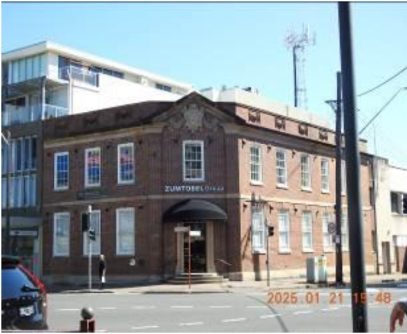
Figure 135 - General condition of external wall
