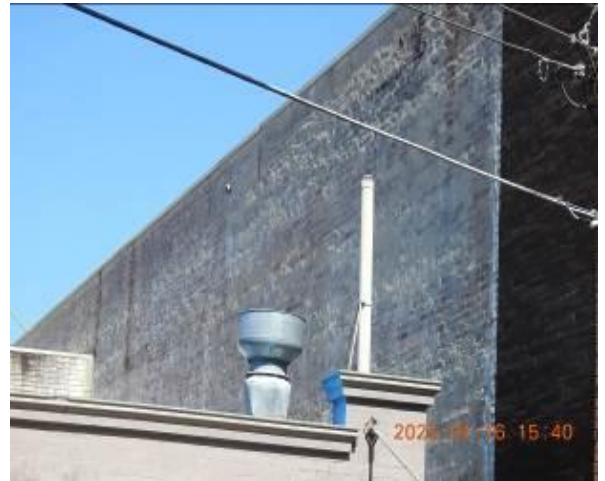
Figure 18 - General condition of external wall
