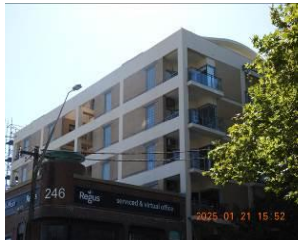
Figure 93 - General condition of external wall
