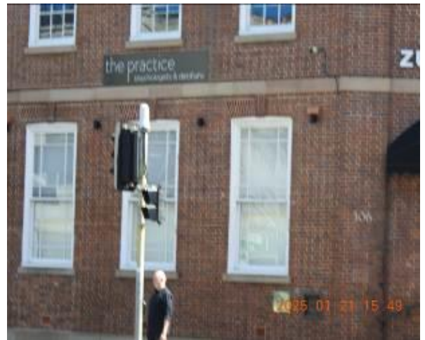
Figure 138 - General condition of external wall
