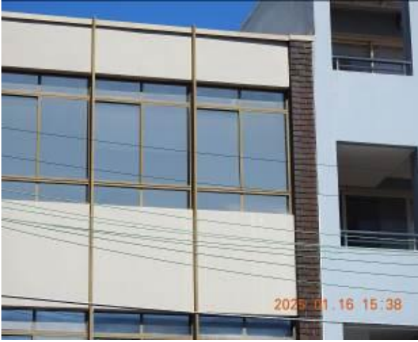
Figure 7 - General condition of external wall
