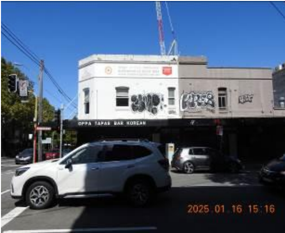
Figure 35 – The Following images displays the general condition of 17 Alexander Street
