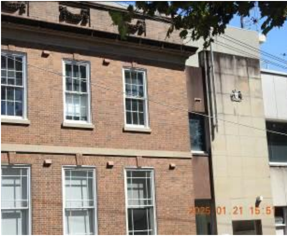
Figure 171 - General condition of external wall
