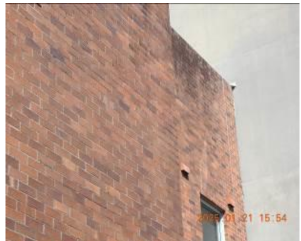
Figure 200 - General condition of external wall
