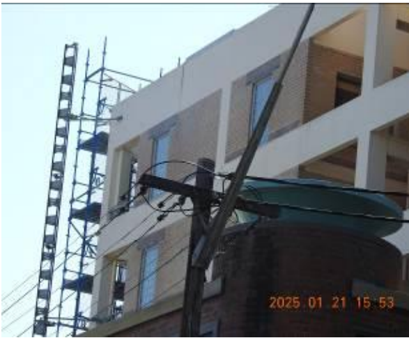
Figure 84 - General condition of external wall
