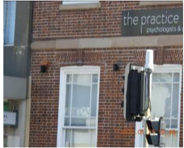
Figure 142 - General condition of external wall
