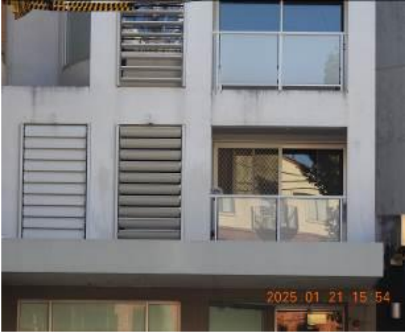
Figure 106 - General condition of external wall
