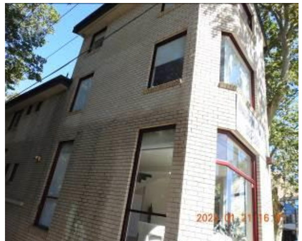
Figure 218 - General condition of external wall
