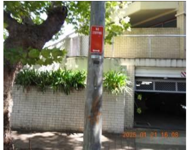
Figure 312 - General condition of external wall
