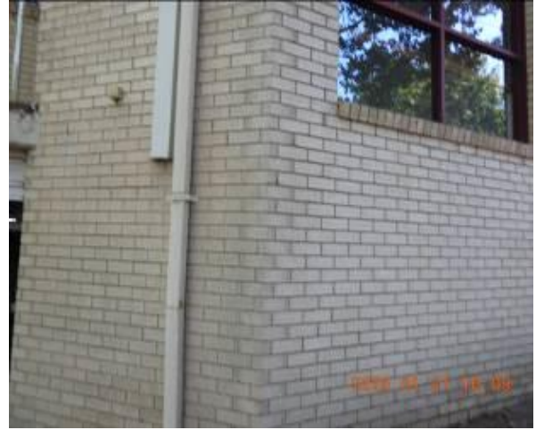
Figure 316 - General condition of external wall
