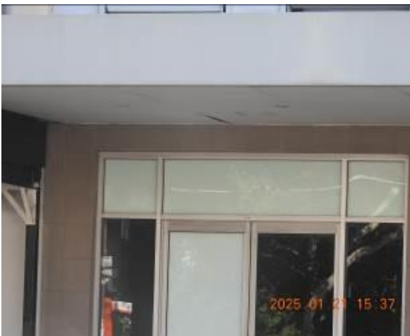
Figure 110 - General condition of external wall
