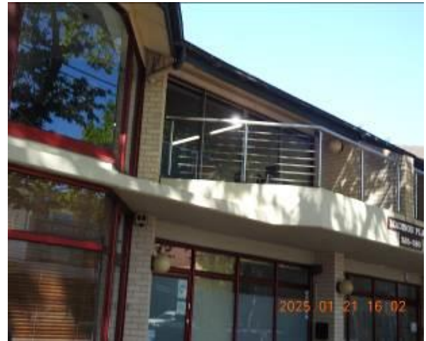
Figure 234 - General condition of external wall
