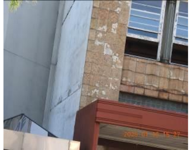
Figure 122 - General condition of external wall
