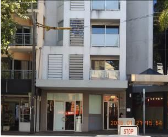
Figure 100 - General condition of external wall
