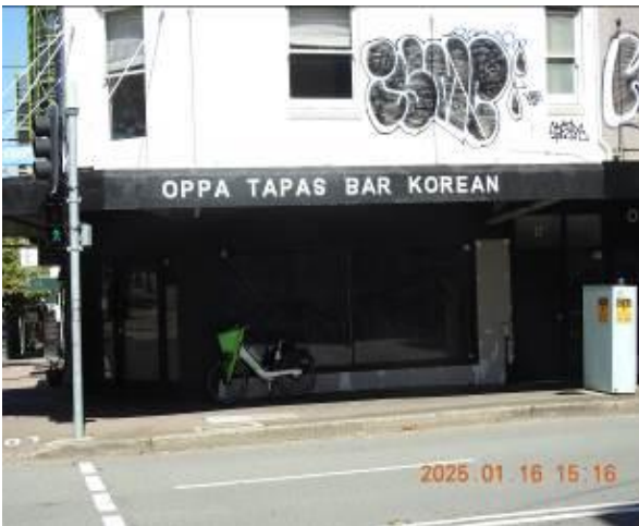
Figure 37 - General condition of external wall
