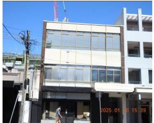
Figure 16 - General condition of external wall
