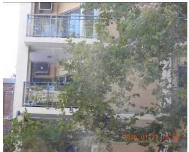
Figure 91 - General condition of external wall
