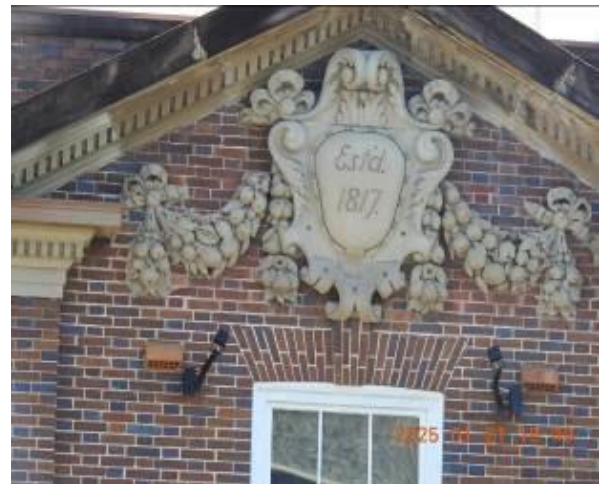
Figure 144 - General condition of external wall
