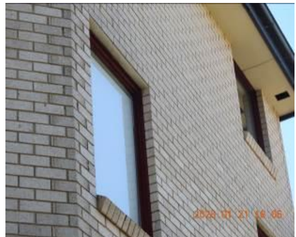
Figure 278 - General condition of external wall
