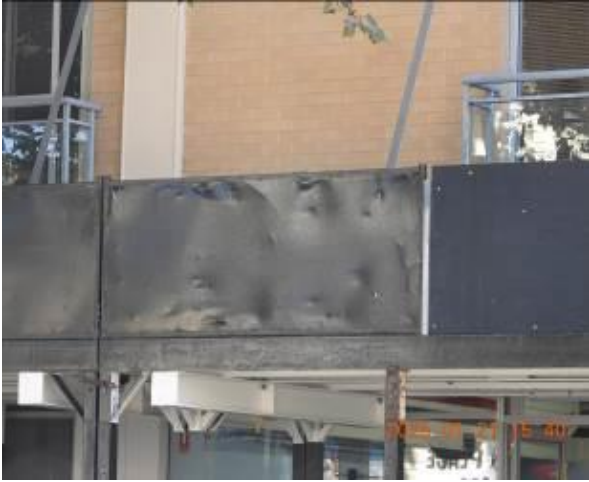
Figure 76 - General condition of external wall
