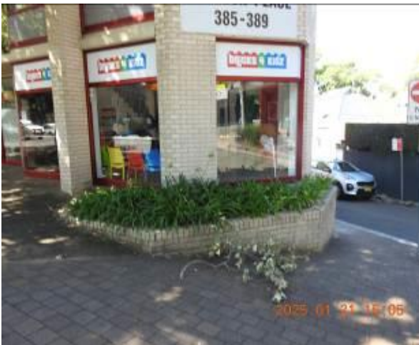
Figure 269 - General condition of retaining wall
