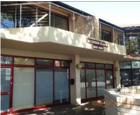
Figure 239 - General condition of external wall
