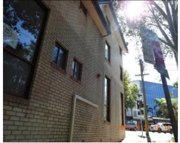
Figure 334 - General condition of external wall
