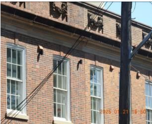
Figure 163 - General condition of external wall
