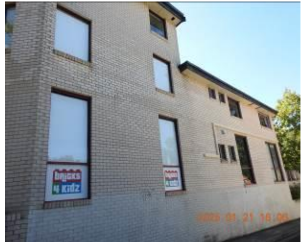
Figure 282 - General condition of external wall
