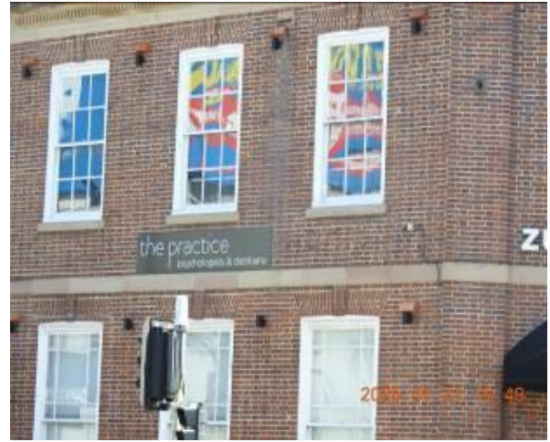
Figure 148 - General condition of external wall
