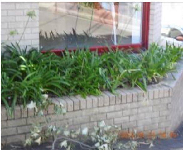
Figure 271 - General condition of retaining wall
