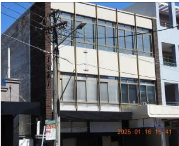
Figure 29 - General condition of external wall
