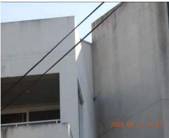
Figure 80 - General condition of external wall
