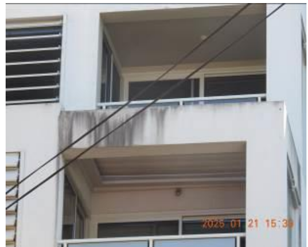
Figure 117 - General condition of external wall
