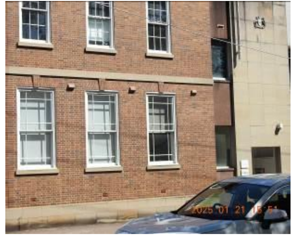
Figure 172 - General condition of external wall
