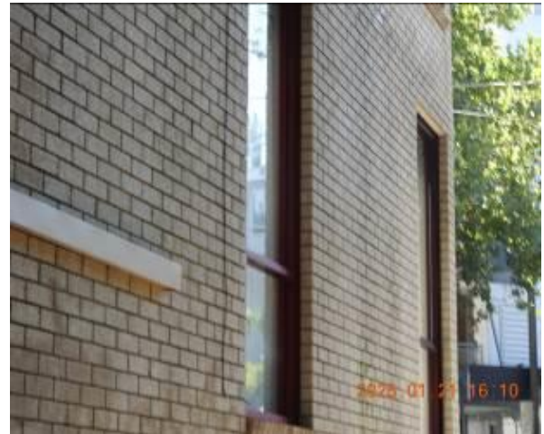
Figure 332 - General condition of external wall
