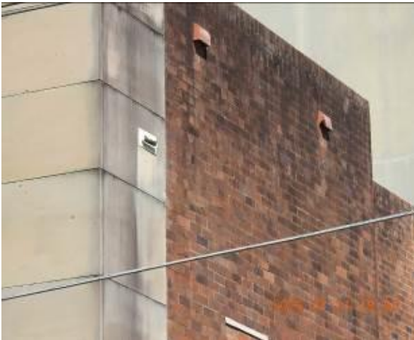
Figure 191 - General condition of external wall
