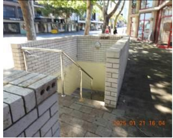
Figure 262 - General condition of external wall
