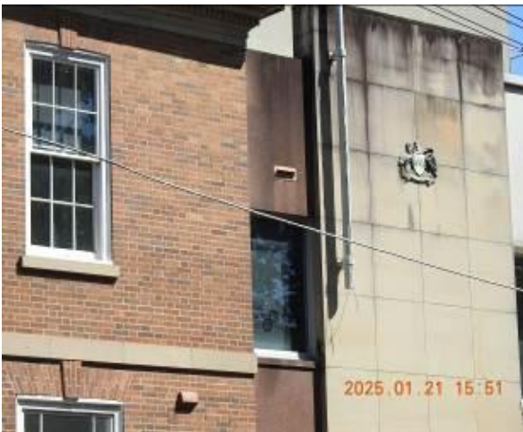
Figure 173 - General condition of external wall
