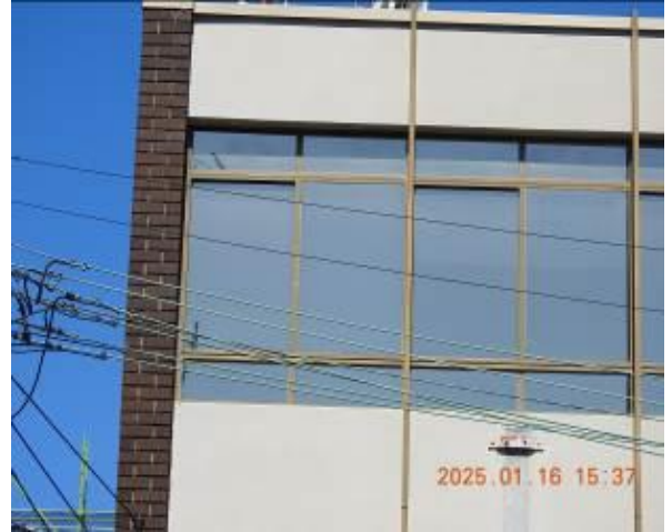
Figure 2 - General condition of external wall
