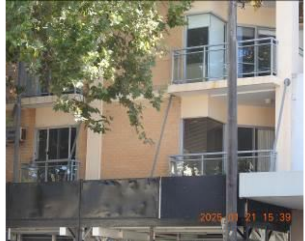
Figure 71 - General condition of external wall
