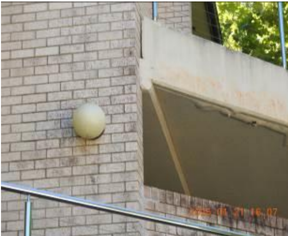
Figure 299 - General condition of external wall
