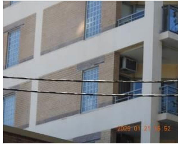
Figure 95 - General condition of external wall
