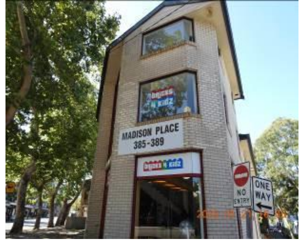
Figure 274 - General condition of external wall
