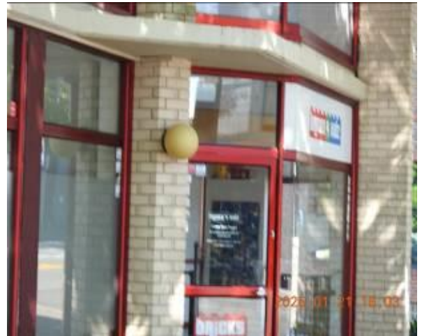
Figure 252 - General condition of external wall
