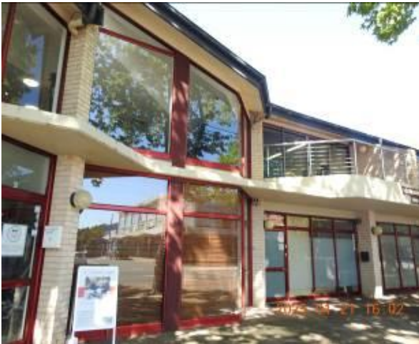
Figure 233 - General condition of external wall
