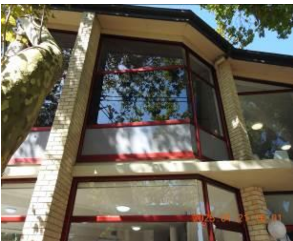
Figure 223 - General condition of external wall
