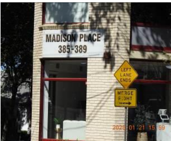
Figure 211 - General condition of external wall
