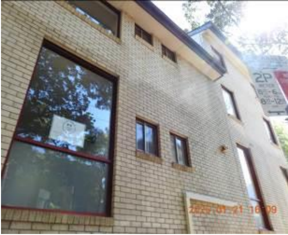
Figure 321 - General condition of external wall
