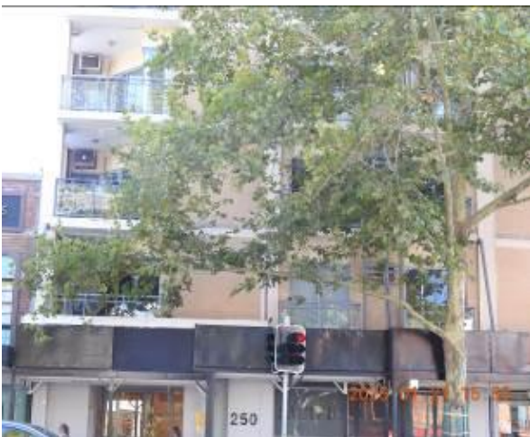
Figure 86 - General condition of external wall
