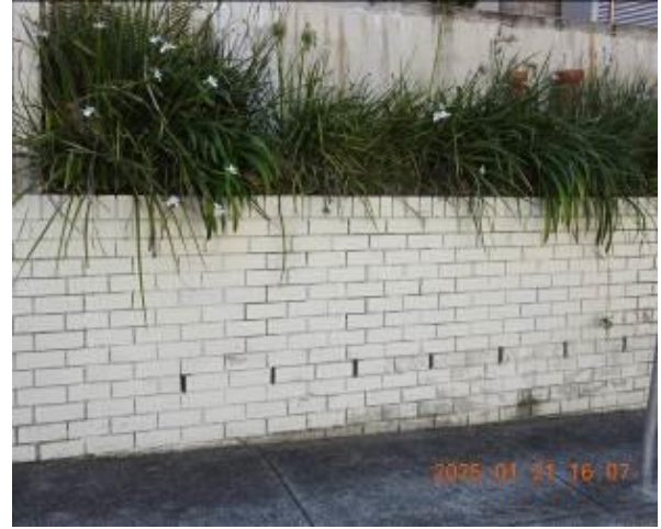
Figure 292 - General condition of retaining wall
