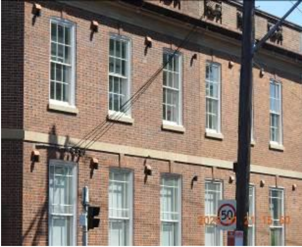
Figure 159 - General condition of external wall
