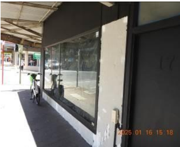
Figure 43 - General condition of external wall
