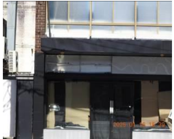
Figure 10 - General condition of external wall
