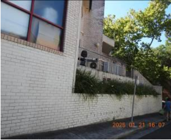
Figure 291 - General condition of external wall
