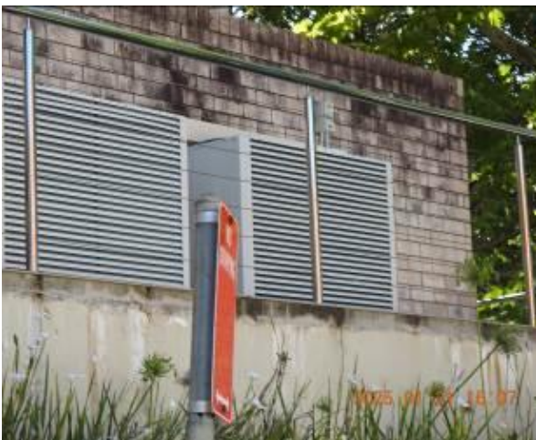
Figure 301 - General condition of external wall
