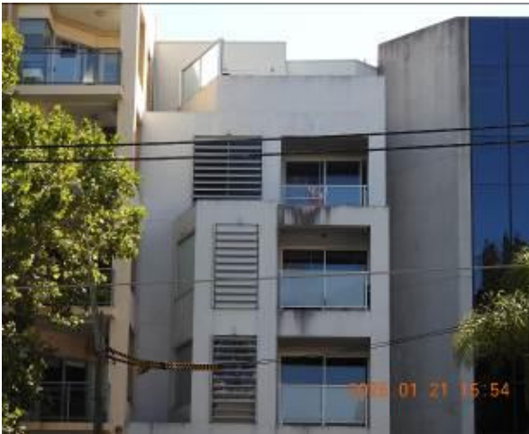
Figure 102 - General condition of external wall
