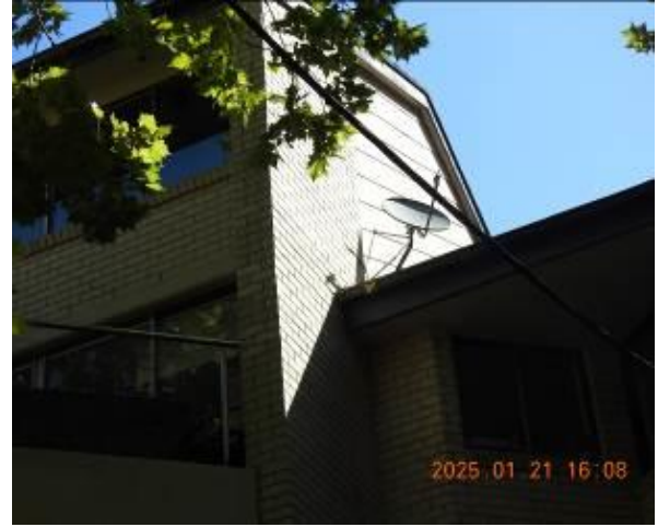
Figure 310 - General condition of external wall
