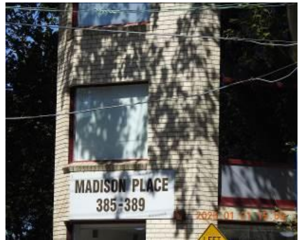
Figure 210 - General condition of external wall
