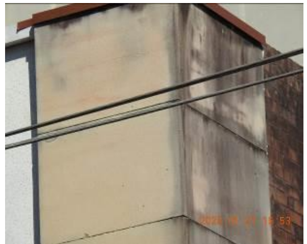
Figure 188 - General condition of external wall
