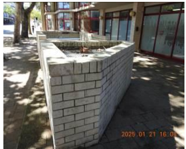
Figure 260 - General condition of retaining wall
