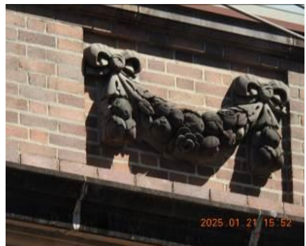
Figure 176 - General condition of external wall
