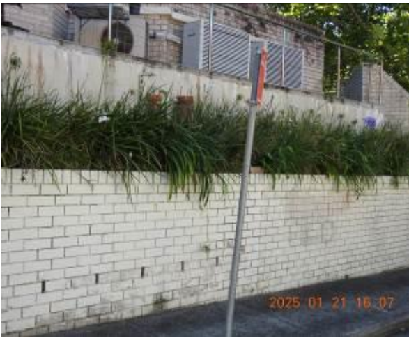
Figure 293 - General condition of external wall
