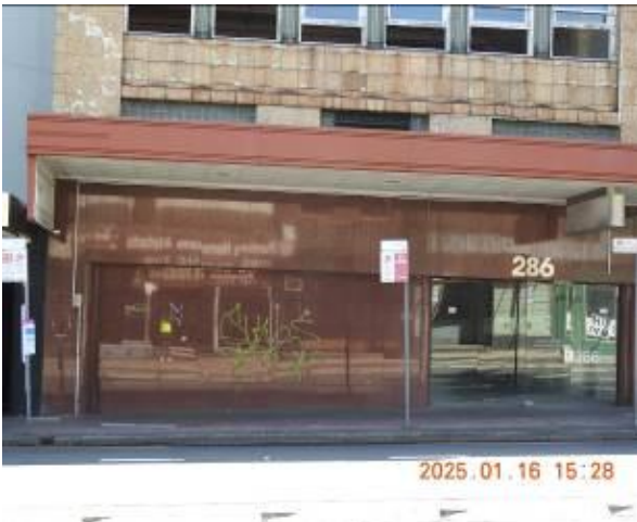
Figure 125 - General condition of external wall
