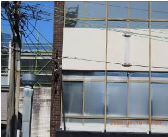
Figure 9 - General condition of external wall
