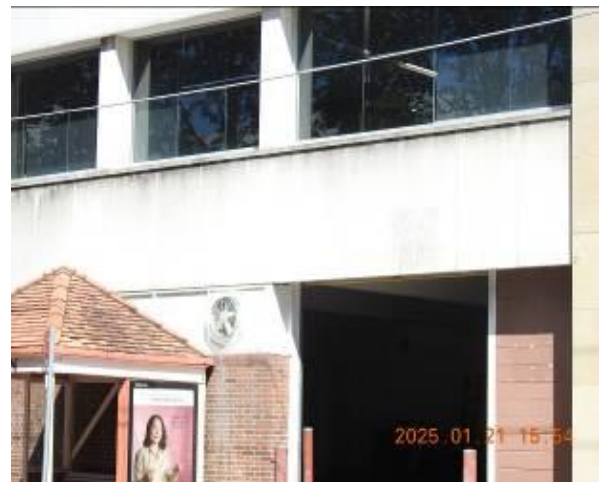
Figure 194 - General condition of external wall
