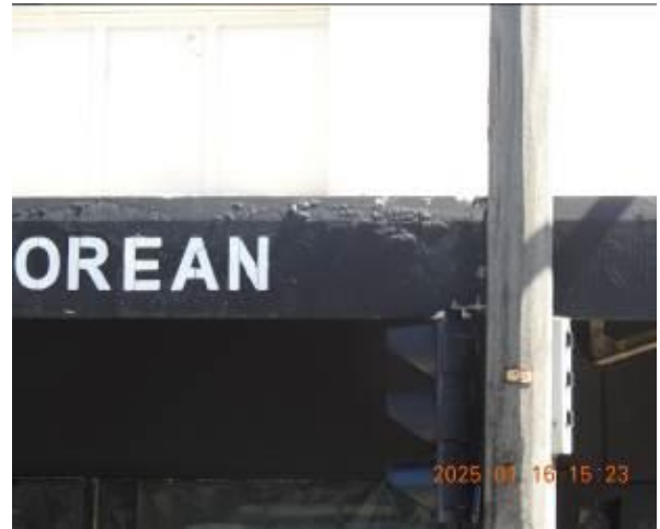
Figure 68 - - General condition of external wall
