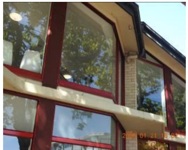
Figure 230 - General condition of external wall
