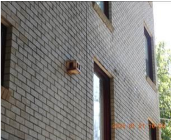
Figure 331 - General condition of external wall
