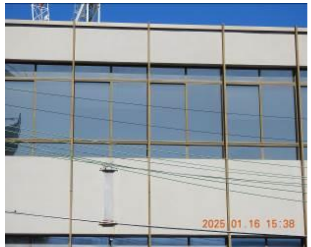
Figure 6 - General condition of external wall
