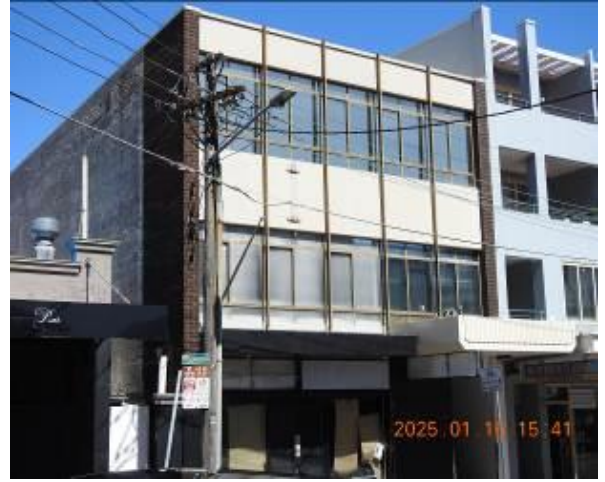
Figure 32 - General condition of external wall
