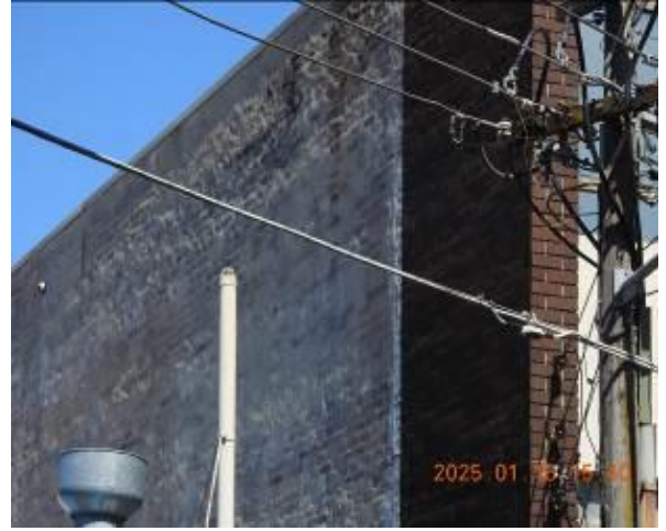
Figure 26 - General condition of external wall
