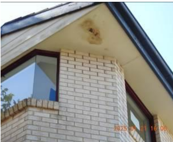
Figure 277 - General condition of external wall
