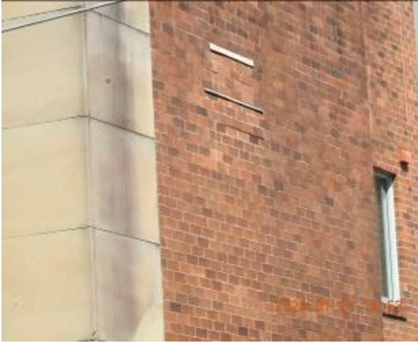
Figure 189 - General condition of external wall
