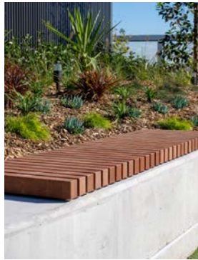
SW: In situ concrete class 2 with timber seating battens and led light strip
