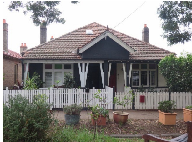
Figure 75 - Nos. 30 and 32 Hayberry Street, is a semi-detached contributory item within the HCA, located opposite a heritage item, and looks at an existing high rise development in the distance on the Pacific Highway.
