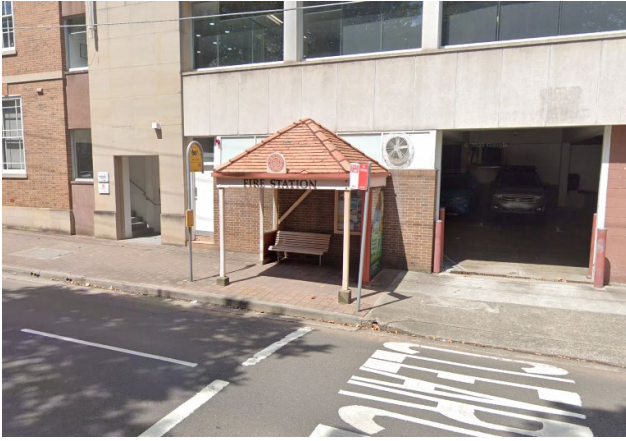
Figure 64 - North Sydney Bus Shelters , Various throughout the North Sydney LGA, item: #I0407.
