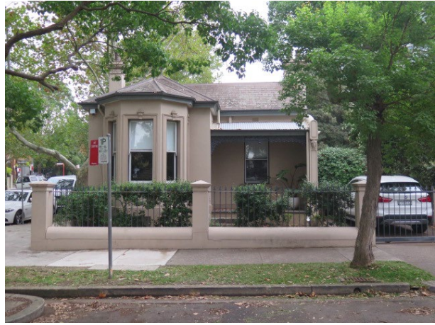
Figure 77 - House at 18 David Street, is a heritage item within the Holtermann Estate C HCA.
