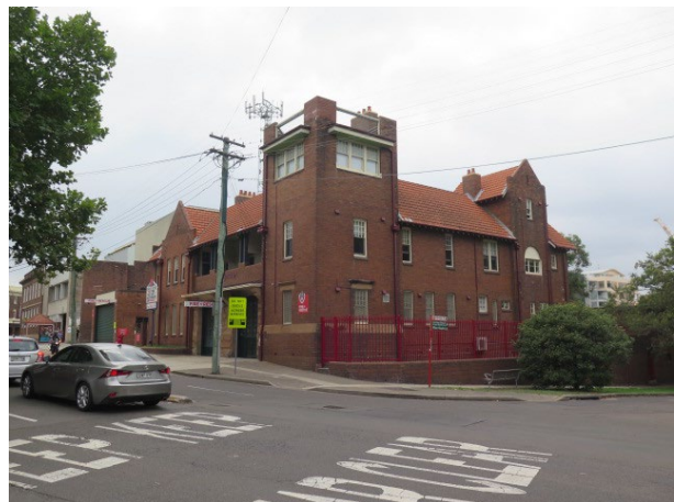
Figure 15 - Crows Nest Fire Station, located at 99 Shirley Road, is a heritage item located west of the subject site. Views looking east to the heritage item are likely to have the proposed development in the background.
