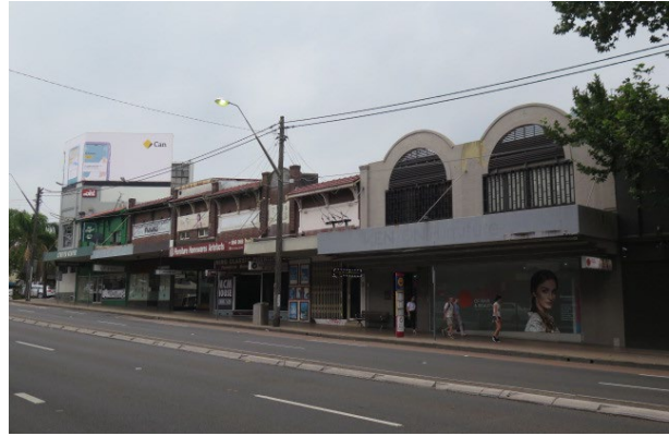
Figure 20 - Subject site with view of two storey, commercial buildings located on the eastern side of the Pacific Highway – Nos 407, 409-419 and 423.
