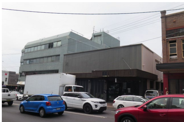
Figure 23 - Subject site (Falcon Street) with view of two-storey and four storey, commercial buildings located on the southern side of the Falcon Street. No 9-11 Falcon Street (right) and 15 Falcon Street (left)
