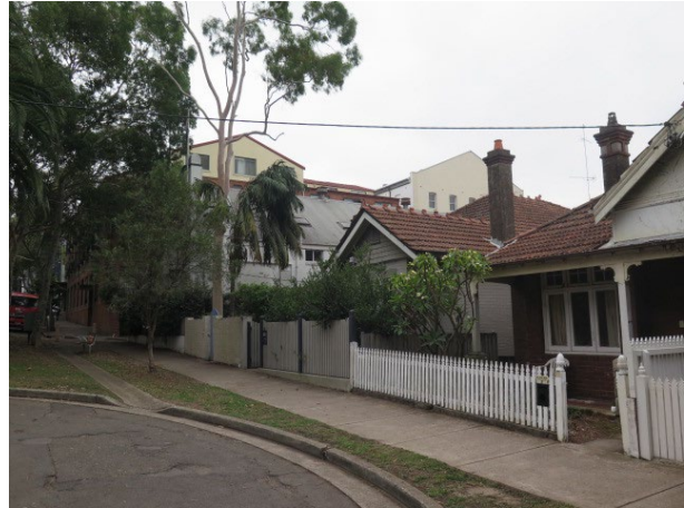
Figure 73 - Views looking northwest from in front of 22 Hayberry Street looking towards the side elevation of the former hall, a heritage item. There are likely to be distant views to the proposed development visible above the roof tops.
