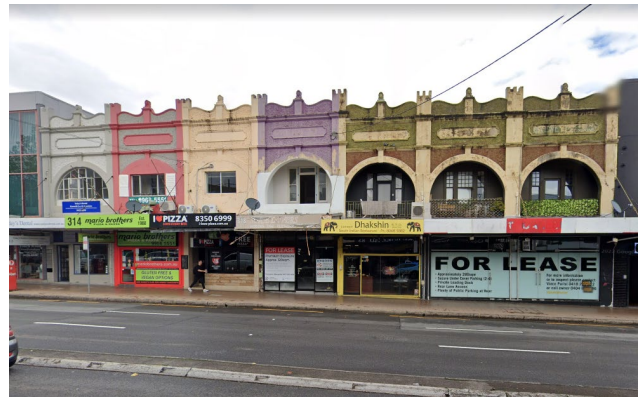
Figure 59 - Shop Group , 312-322 Pacific Highway, items: #I0153, #I0154, #I0155, #I0156, #I0157, #I0158.
