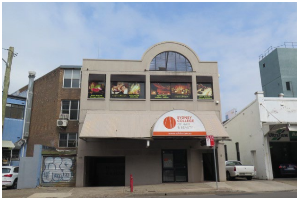
Figure 27 - View to No 6 Alexander Street (centre), a two storey, late-20th century commercial building. Rear vehicular access to buildings addressing Pacific Highway provided off this street.
