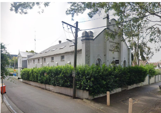
Figure 62 - Former Hall , 14 Hayberry Street, Crows Nest, item: #I0144.
