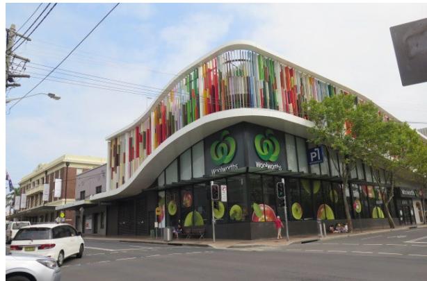
Figure 13 - Woolworths store located on the corner of Alexander and Falcon Streets, opposite and north of the subject site.
