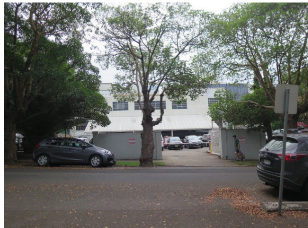
Figure 9 - View from Sinclair Street to the rear of the Former North Shore Gas Co Office. The proposed development is likely to be visible above the roof tops. Views to the proposed development will be screened by street plantings.
