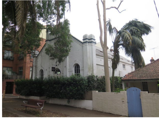
Figure 69 - Former Hall, located at 14 Hayberry Street, Crows Nest, is a heritage item located east of the subject site within the Holtermann Estate C HCA. The proposed development may be visible in the background when viewing the heritage item from the east on the lower gradient of Hayberry Street within the HCA.
