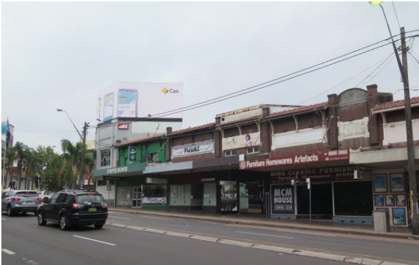
Figure 21 - Subject site (Pacific Highway) with view of two storey, commercial buildings located on the eastern side of the Pacific Highway – Nos 409-419 and 423.
