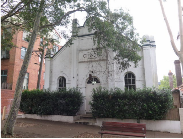
Figure 68 - Former Hall, located at 14 Hayberry Street, Crows Nest, is a heritage item located east of the subject site within the Holtermann Estate C HCA.
