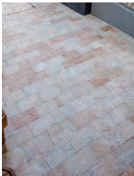
P2: Paving to Council Standards
