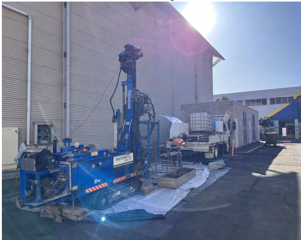
Photo 12 - Typical Drill Rig Set-Up Overlaying a Tarp
