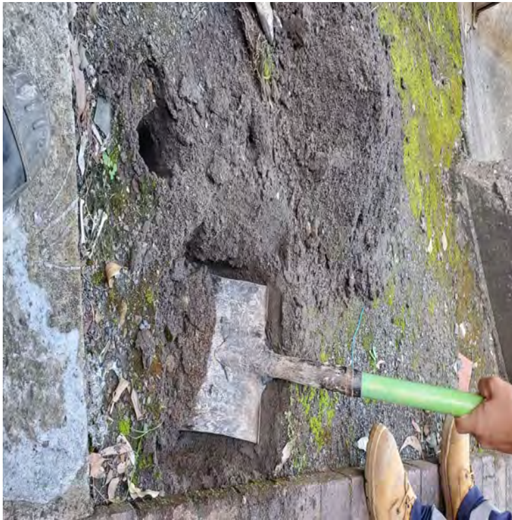
Photo 9 - Excavating the surface of BH08 prior to using the hand auger
