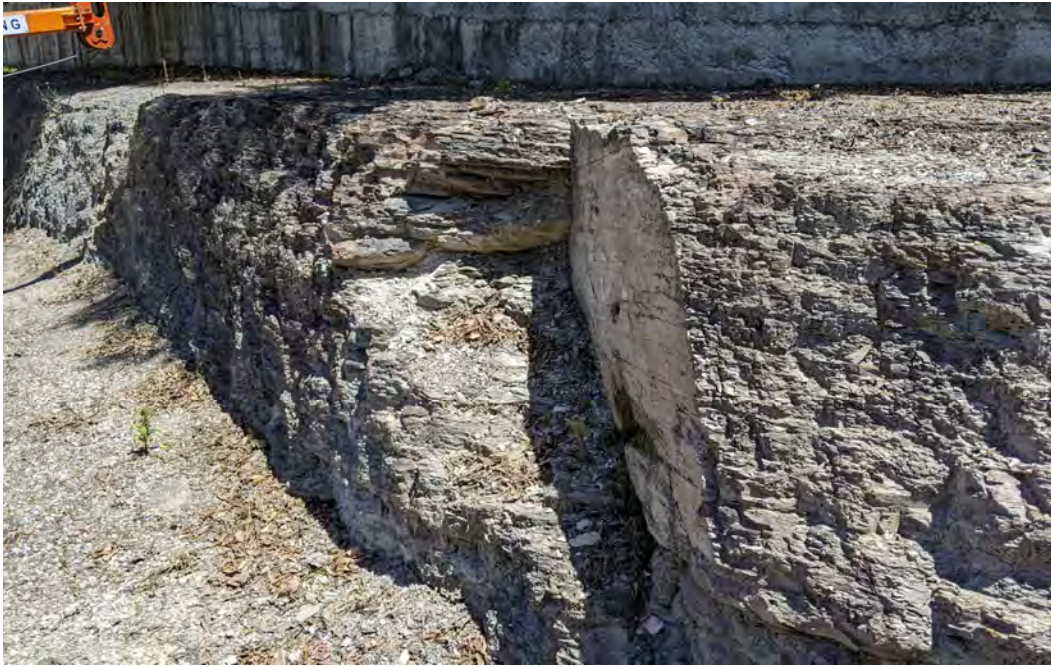
Photo 5 - Joint observed in rock cutting along south-west boundary of the site
