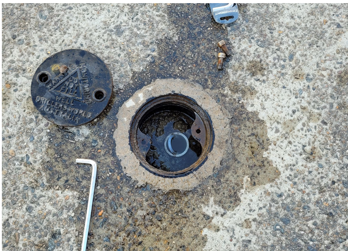
Photo 4 - Condition of BH12 on 26 July 2023 following removal of PVC Cap
