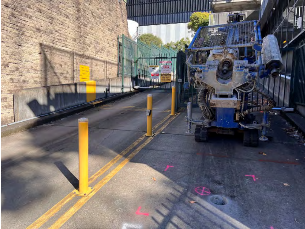
Photo 13 - Drilling Conditions on a Ramp for BH10
