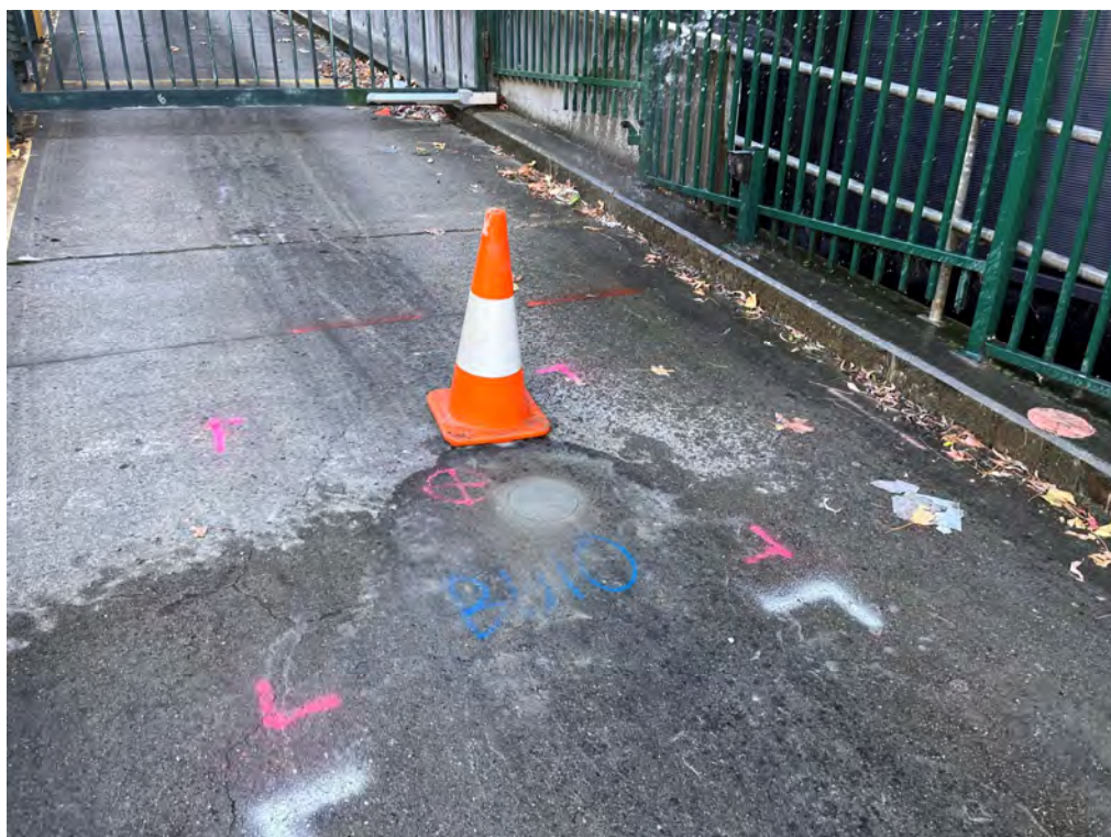
Photo 16 - Reinstated hole at BH10
