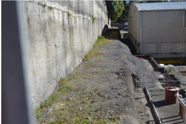
Figure 13. View to north from multi-story car park at number 8 Lanceley Road. Original sandstone has been cut and covered with formed and poured in-situ concrete (left) and shotcrete (at centre).
