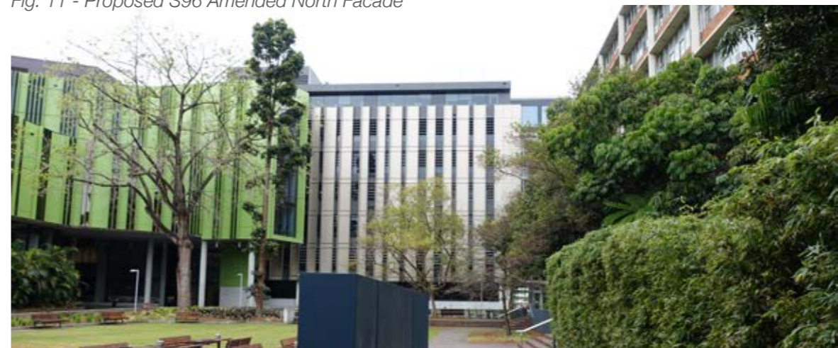
Fig. 12 - Existing adjacent buildings (Lowy Centre, left, and Wallace Wurth) - Vertical articulation
