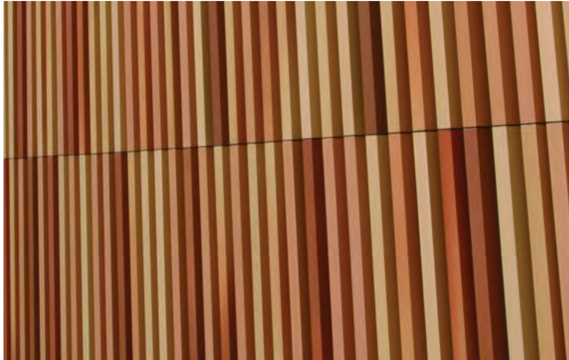
Vertical coloured terracotta blades (Facade B)
