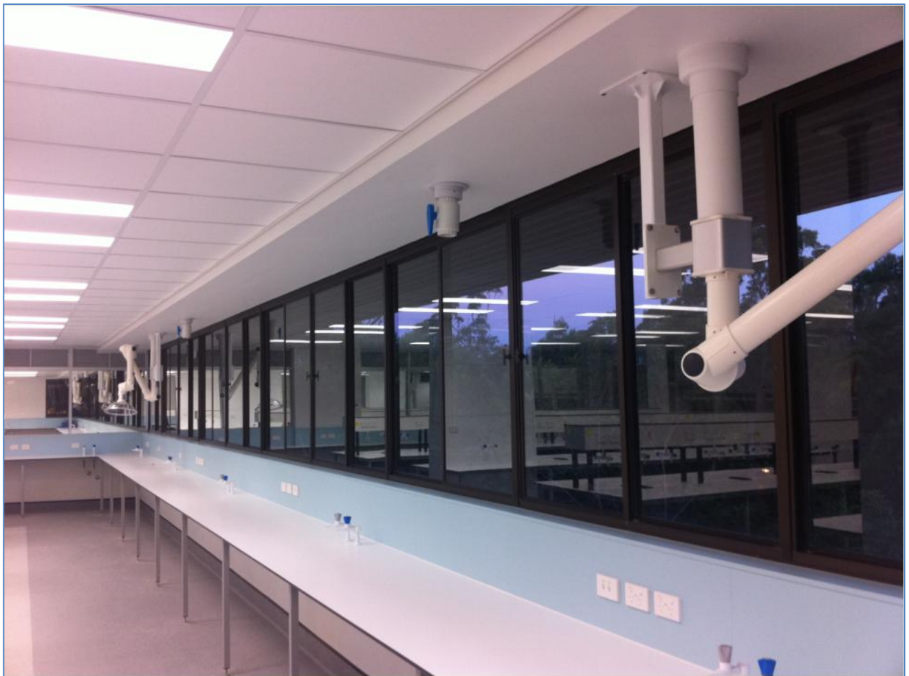
Figure 3 - Proposed BSC fumigation exhaust point arrangement
