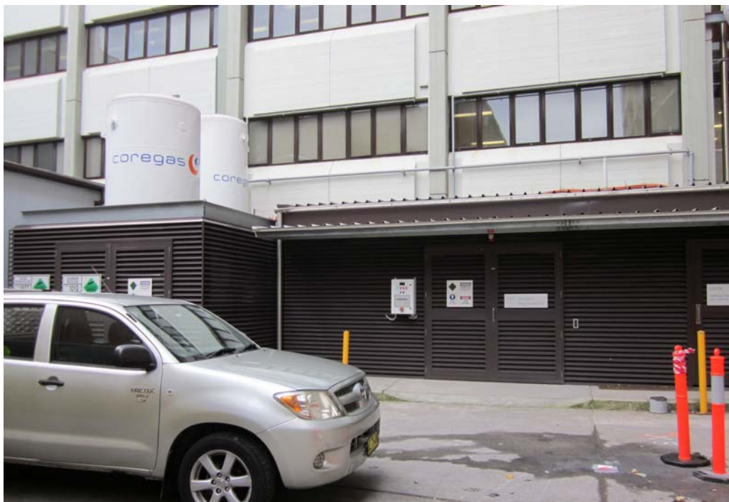
Photo 3 – Dangerous goods stored to the west of the Biomedical Theatres.
