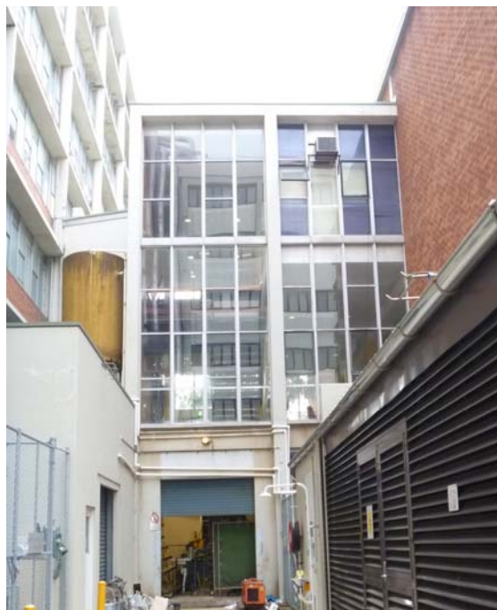
Photo 6 – Biological hazard waste, chemical waste and general waste storage area located at the rear of the Biomedical Theatres.
