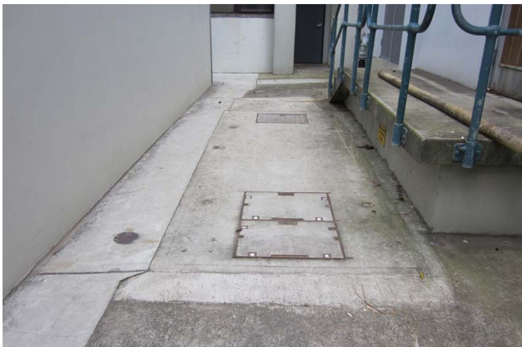
Photo 4 – Liquid trade waste tank observed between the BEES Work Area and Substation No. 6.
