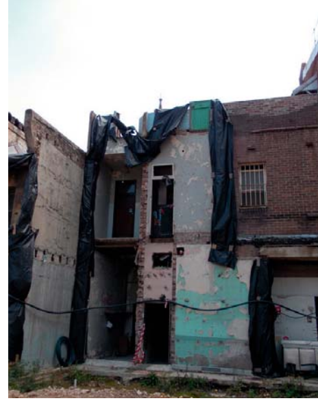
View of the demolished staircase to the Australian Hotel
