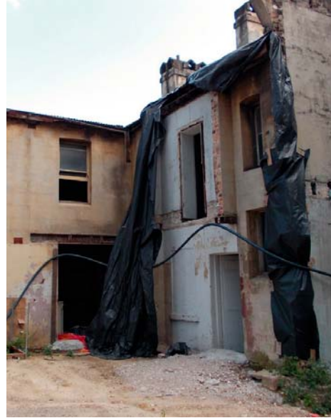
View the demolished extension to one of the Terraces
