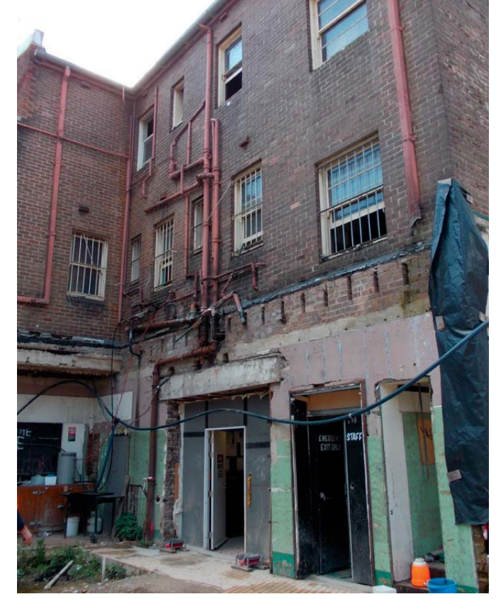
View of the rear of the Australian Hotel
