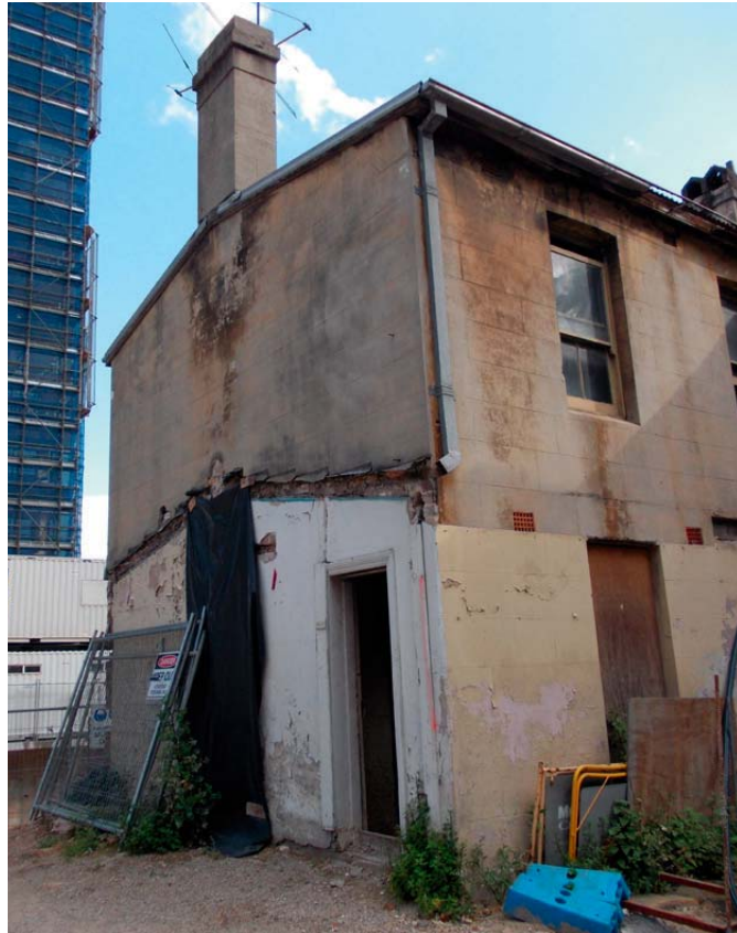
View of the rear of the historical Terraces
