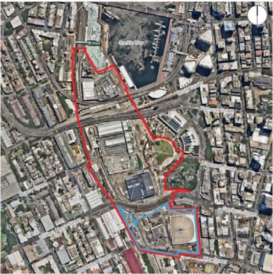
Figure 1 – Aerial Photograph of the SICEEP Site
