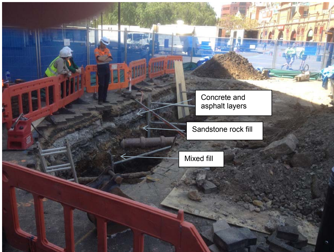
Photograph 1: Archaeological Excavation at approximate R2-5 location
