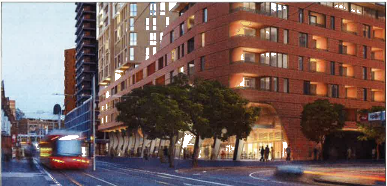
Figure 4: View towards the south east corner of the podium and the undercroft/colonnade fronting the light rail corridor / Hay Street (Source: applicant's EIS)
