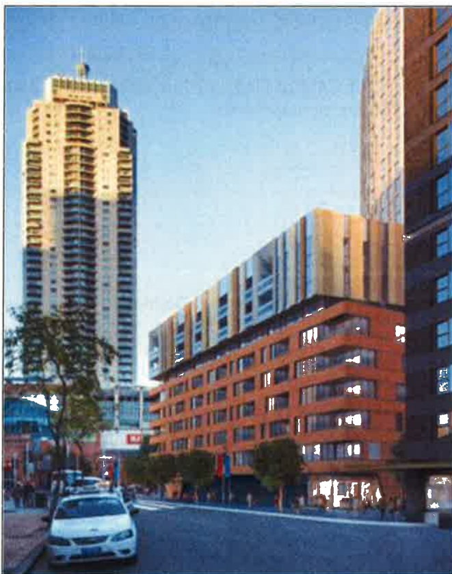
Figure 6: View south along Harbour Street (Source: applicant's EIS)
