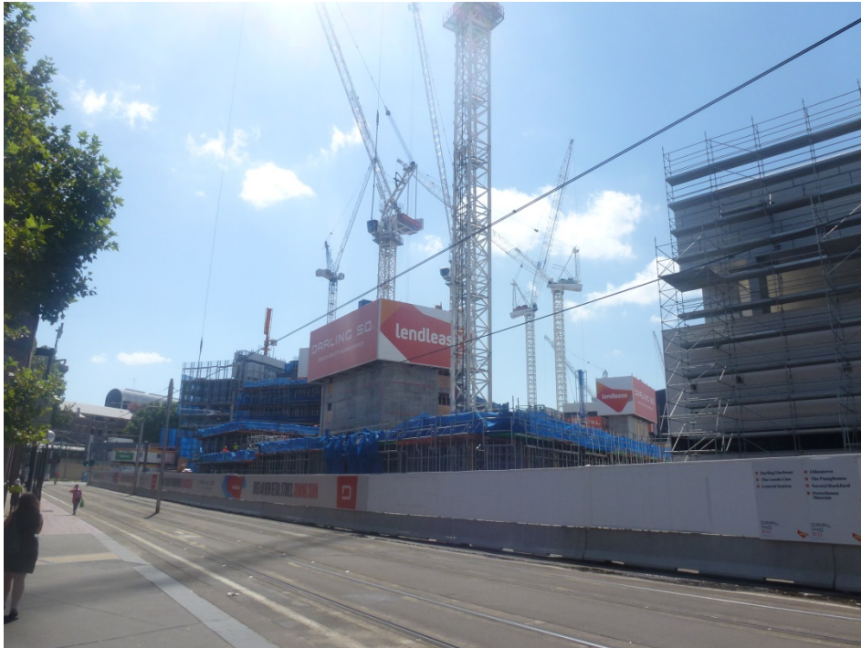
Figure 19 – South West Plot under construction
