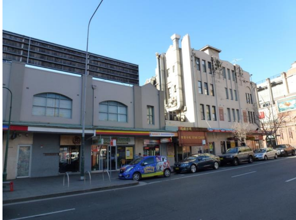
Figure 15 – Harbour Street retail and restaurant buildings
