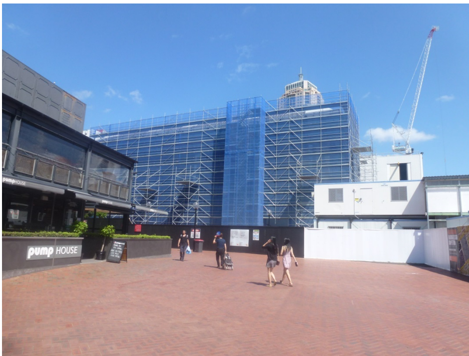
Figure 14 – Northern Public plaza in front of the SEC
