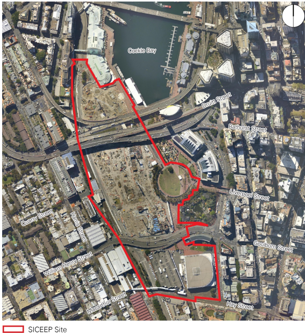
Figure 1 – Aerial Photograph of the SICEEP Site
