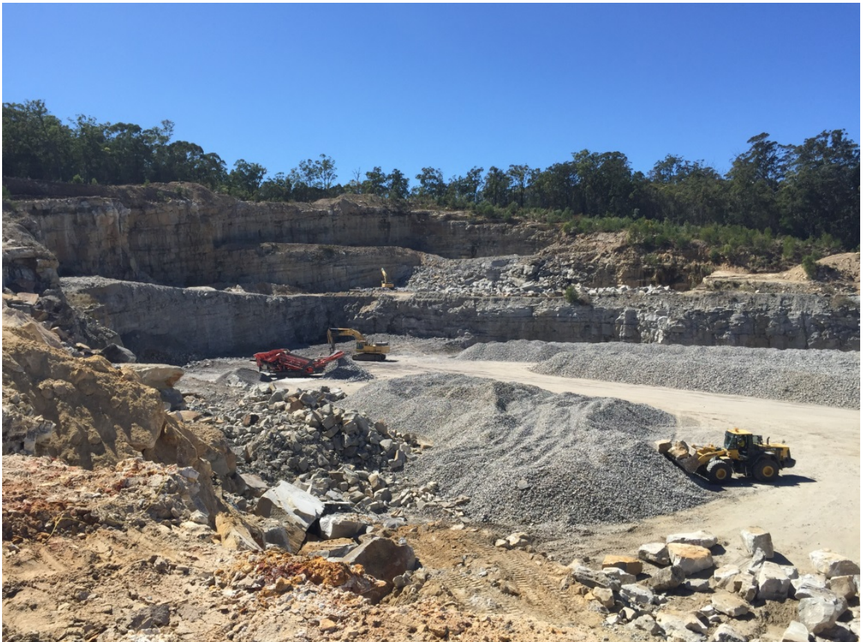
Photo 1: View of the quarry from the western cut face. Benches are spaced at around 10 m in height and the base of the quarry at around 44 m AHD. The dip of the sandstone beds to the north west, the left of the image is clearly visible.
