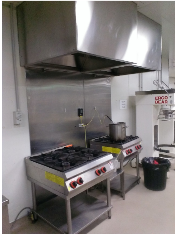
Figure A - 1: Gas stoves with overhead extraction system
