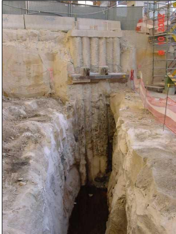
Plate 7.1 Photograph showing main gas holder annulus, secant pile wall and upper waler beam and ground anchors (Source: Lend Lease)
