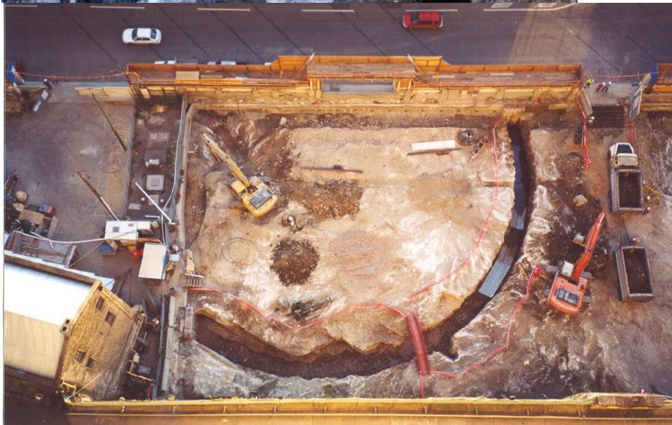
Figure 3.22: View of the the eastern part of the annulus, cut into bedrock, found beneath the Bond during works in 2002. Bedrock is quite high in this area. Mark Burns, Lend Lease.
