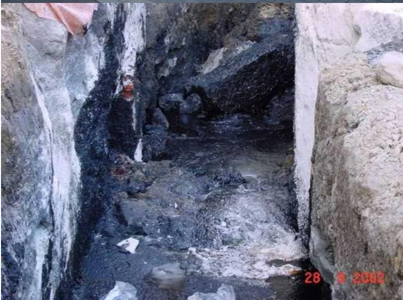
Figure 3.21: Tar contamination apparently uncovered during construction works in September 2002. Mark Burns, Lend Lease (Millers Point)
