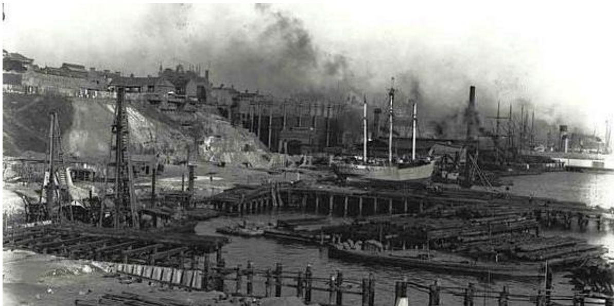
Figure 3.16: View to the southeast showing the large gas holder on Block 4 and the southern part of Hickson Road. The rocky face to the north of the gas holder was cut back when Hickson Road was built in the early twentieth century. View of the reconstruction of Darling Harbour from Millers Point showing Dalgetys Wharf No.1 partly completed, 1/1/1909, State Records 9856_ao17_AO17000007.
