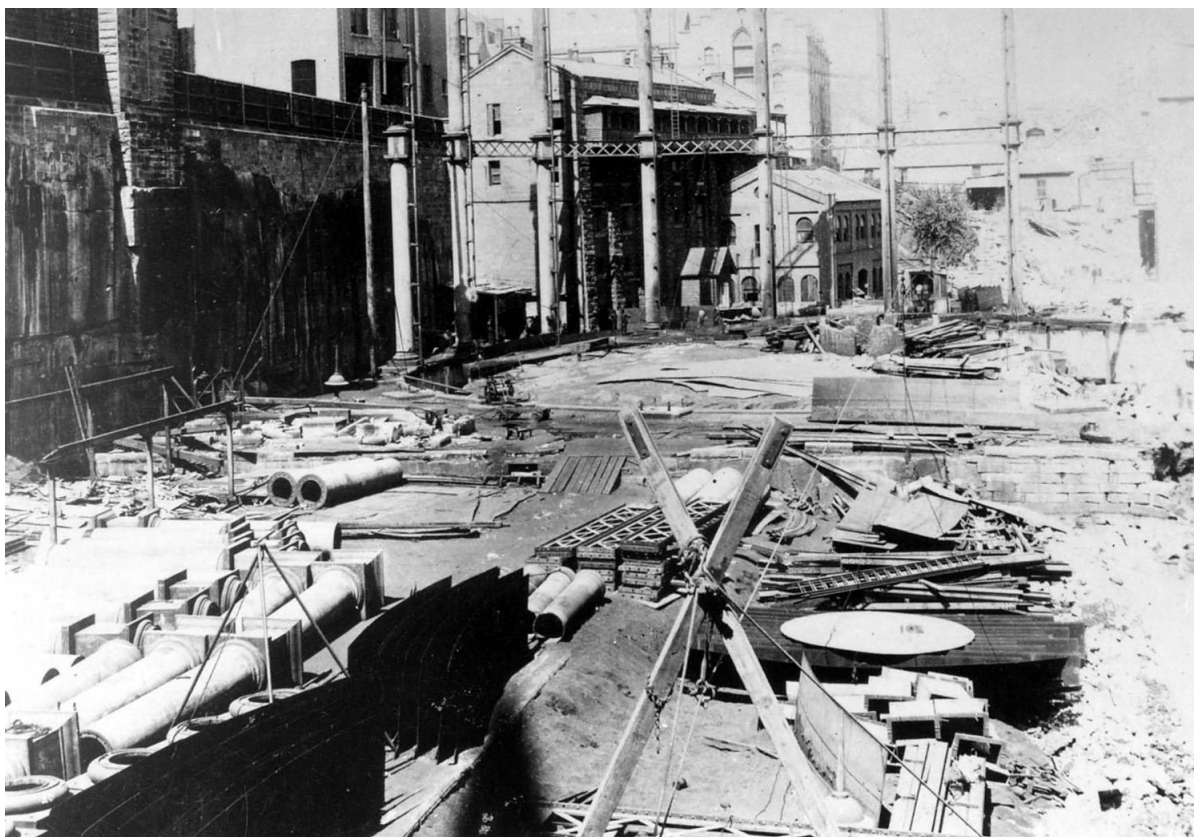
Figure 3.17: AGL site during demolition, c. 1922, showing the northern side of the five-storey sandstone office and store with the balcony on the western side and the brick building in front of it. The telescopic holder in the middle ground was being dismantled. The cutting for the holder, excavated deep into the bedrock, was recorded during the construction works for the Bond in 2002 (Archaeology & Heritage 2004). AGL Archives, from Broomham 2007:43.
