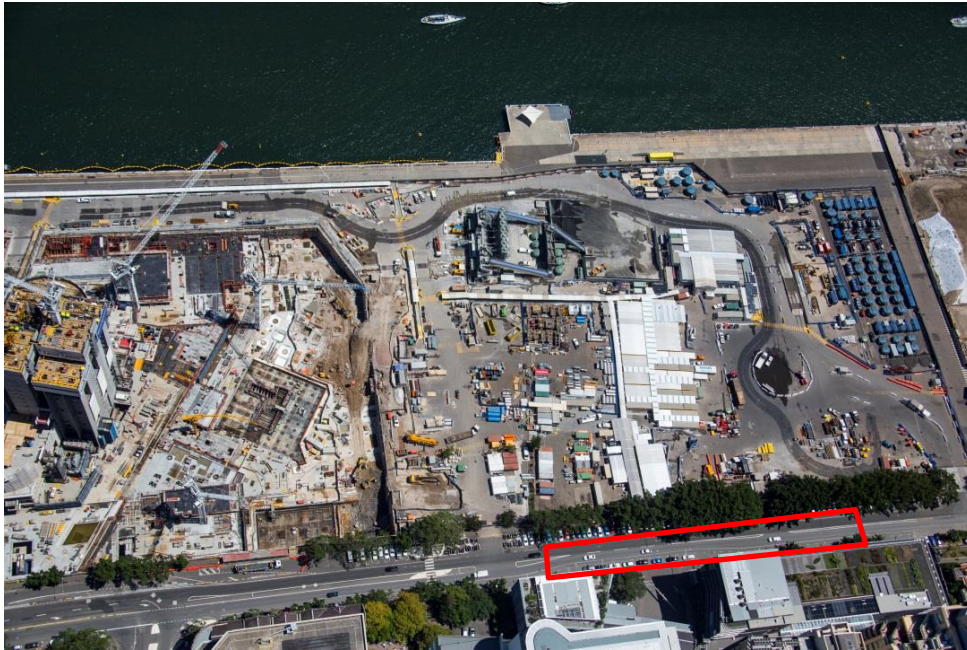
Figure 10 – Recent Visual Context of the site (from the east) (The red line shows the approximate extent of the Hickson Road Remediation Area)
