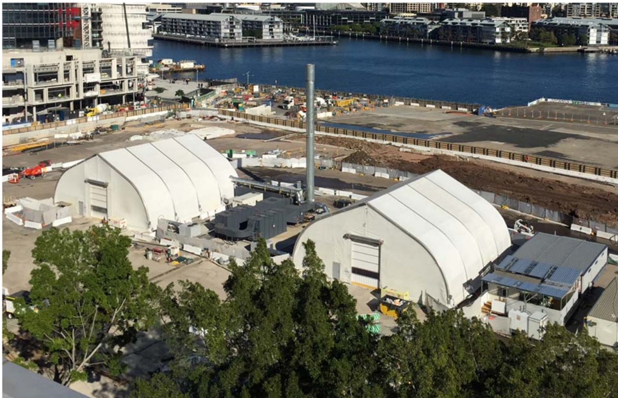
Figure 11: Example of excavation enclosures on site at Barangaroo (Source: site visit 29 June 2016)
