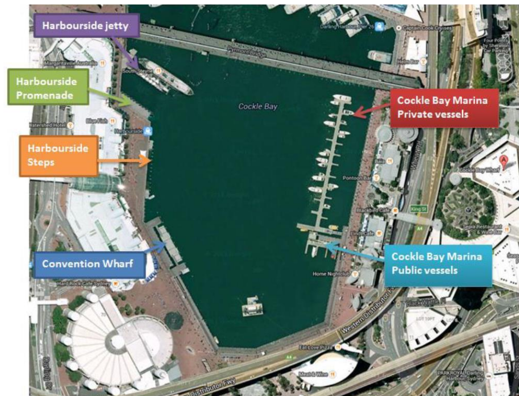
Figure 1.2 Existing Marine Structures in Cockle Bay (Source: Sydney Harbour Foreshore Authority, 2014b)
